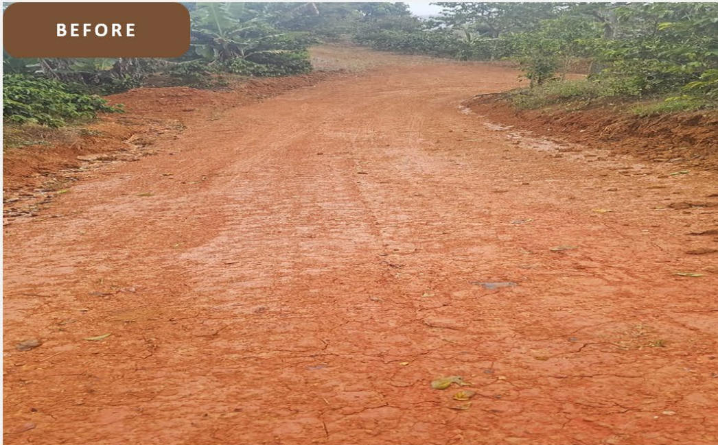
Bare clay running surface on grade, before construction (NRCS, May 2026)
