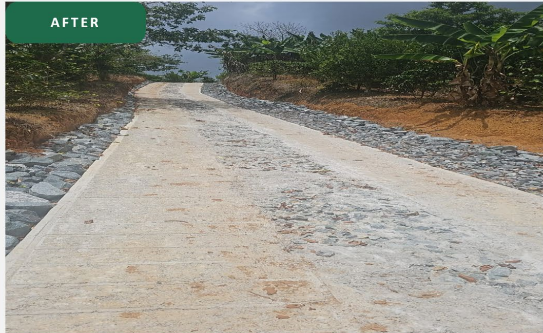
Completed placa huella on the same alignment (NRCS, July 2026)
