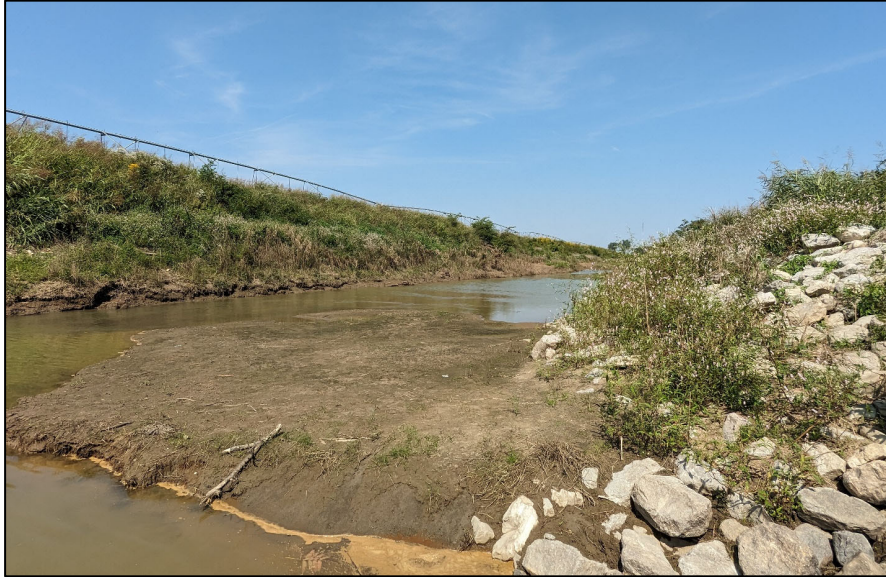
Photo: Ditch Number 1 at confluence with Caney Creek, looking upstream, Conservation Works Joint Venture Partner September 2023.
