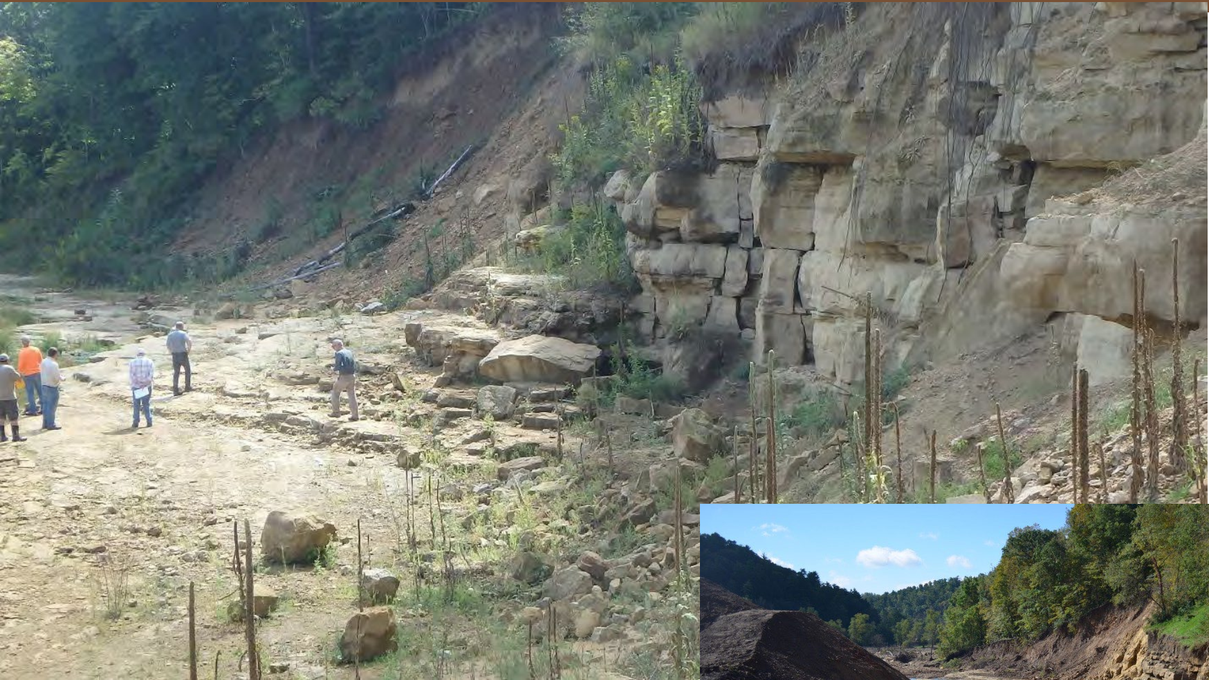
Fractured sandstone abutments exposed at WFK 1 after dam failure
