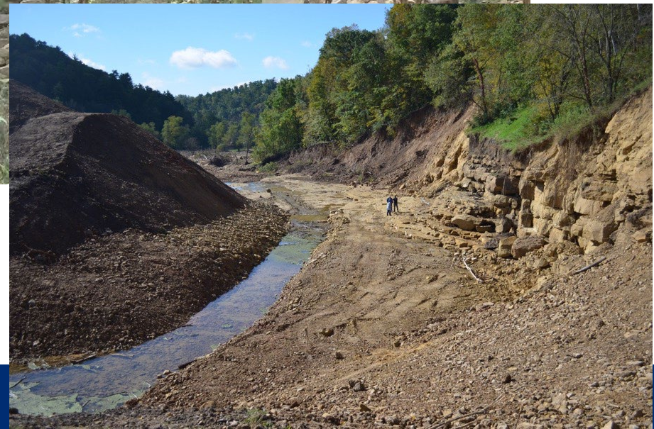
Fractured sandstone abutments exposed at WFK 1 after dam failure
