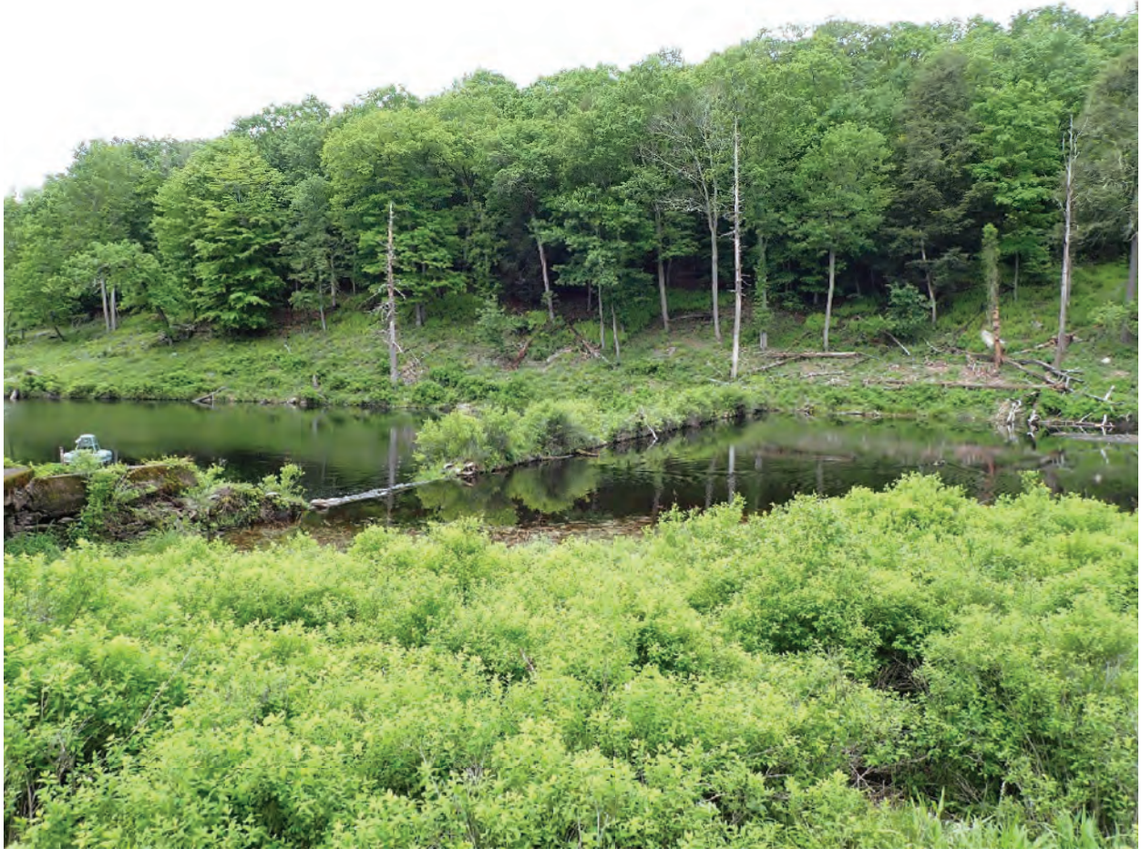
Southwest-facing view of early dam concrete structure constructed across Goose Pond (18N 480141 4561868). The early dam was documented having been constructed as early as the late 1930s
