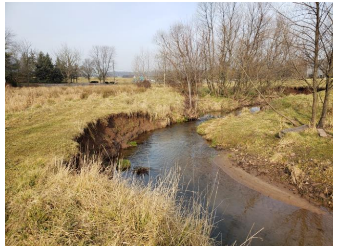
Figure 2: Typical section of stream at EU 5
