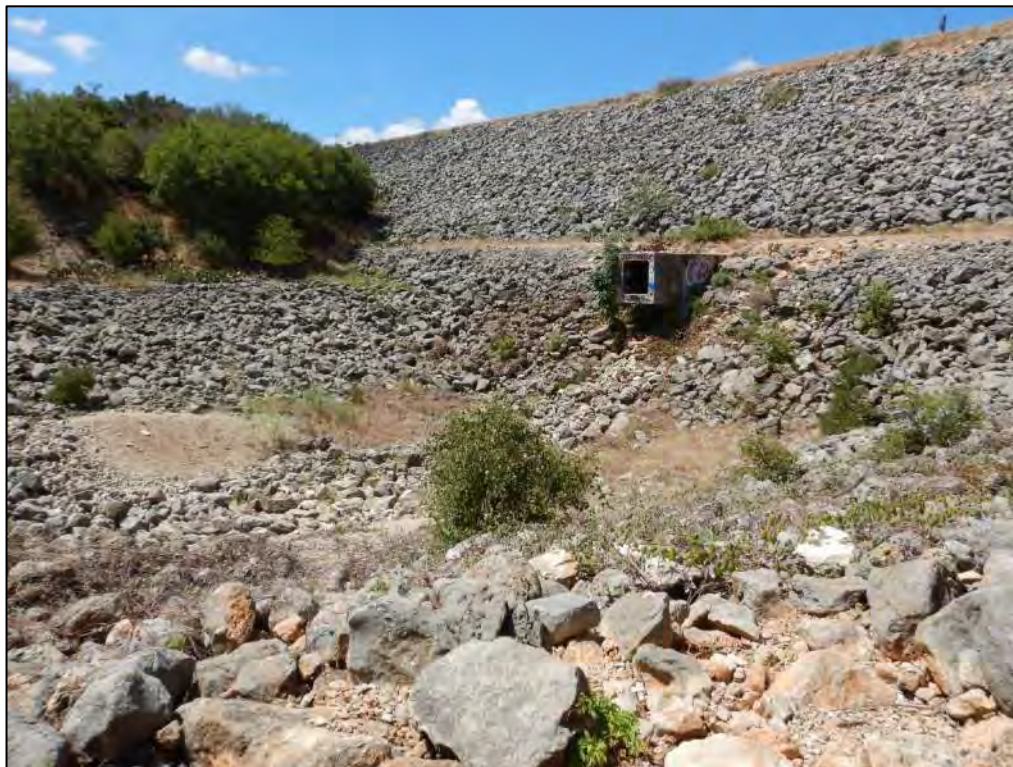
Photo 5. View looking southwest at the principal spillway outfall and plunge pool of the Upper San Marcos Site 5 FRS where it outfalls into the vegetated channel of Purgatory Creek.
