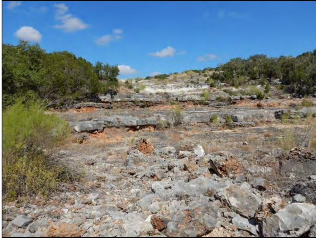
Photo 9. View looking northwest at the auxiliary spillway of the Upper San Marcos Site 4 FRS and adjacent Ashe juniper, which may be potential habitat for golden-cheeked warblers.
