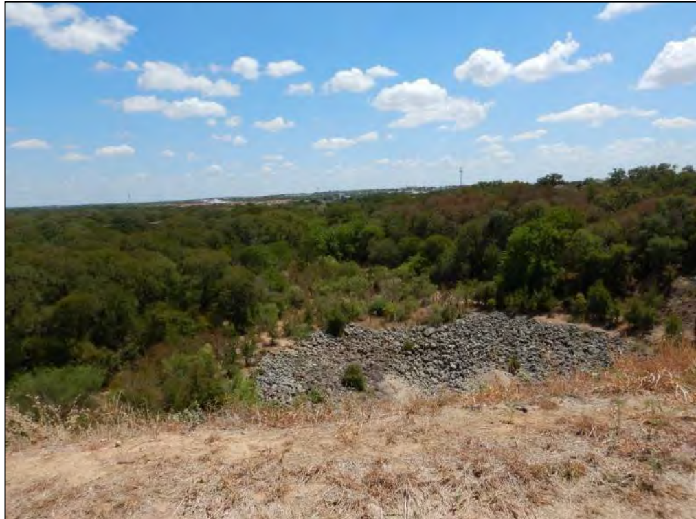
Photo 4. View looking east (downstream) at Purgatory Creek, and the principal spillway outfall and plunge pool of the Upper San Marcos Site 5 FRS.
