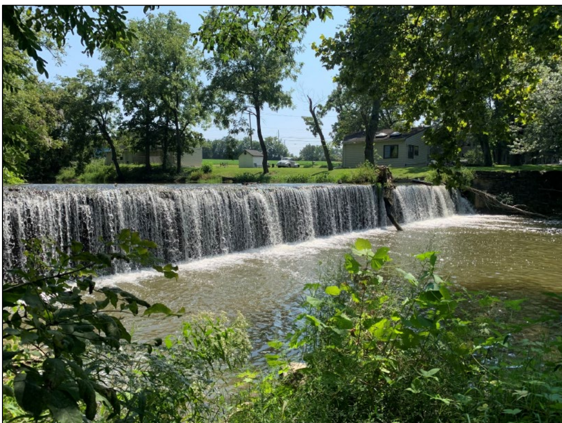
Figure 2.2 Chiques Roller Mill Dam Photo 2
