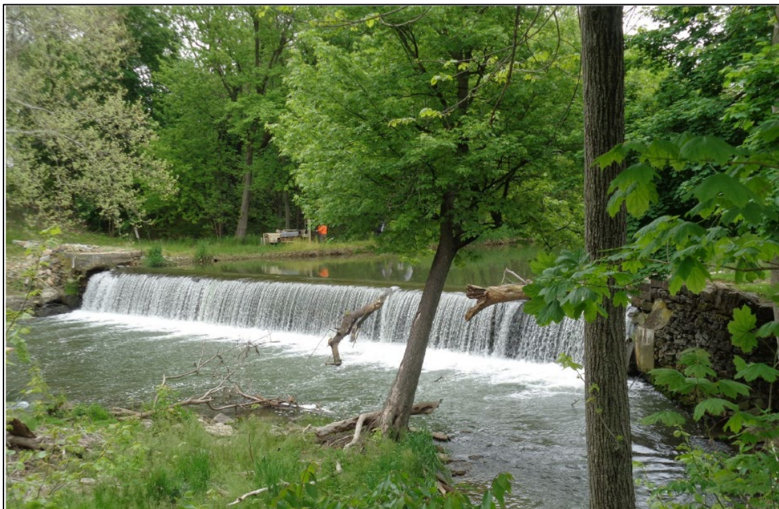
Figure 2.1 Chiques Roller Mill Dam Photo 1
