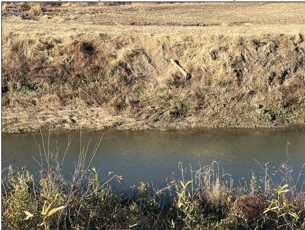
Figure 6.5. View of canal interior, facing west.
