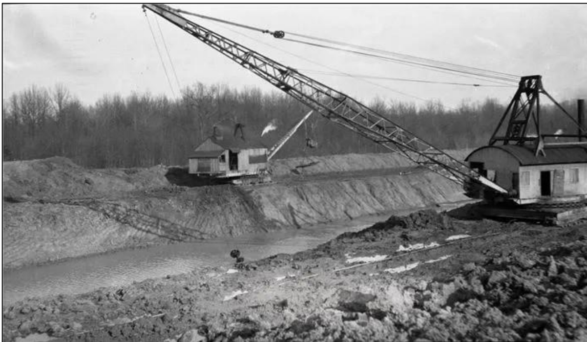
Figure 3.2. Canal construction, circa 1918 (The Little River Drainage District 2024).
