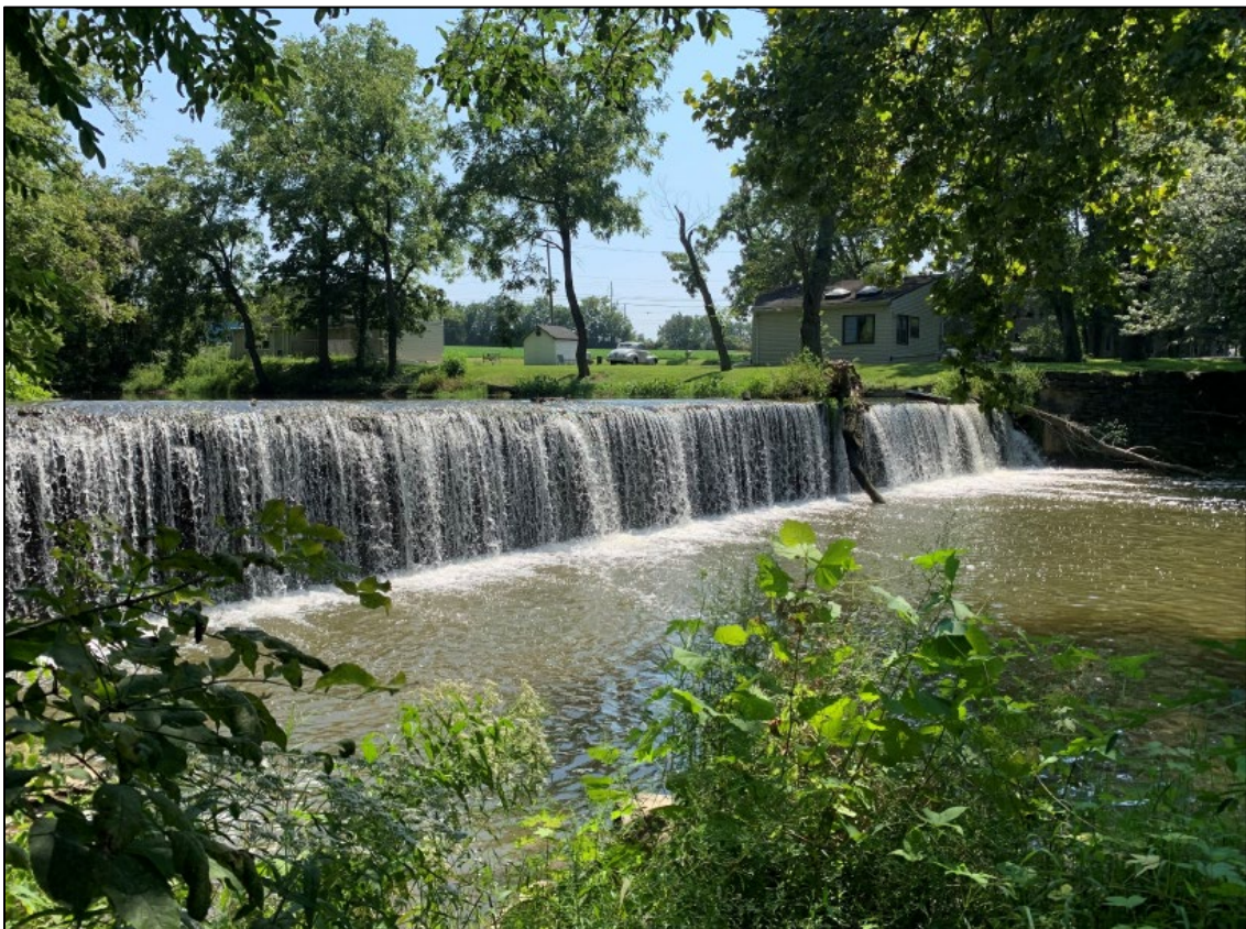
Figure 2.2 Chiques Roller Mill Dam Photo 2
