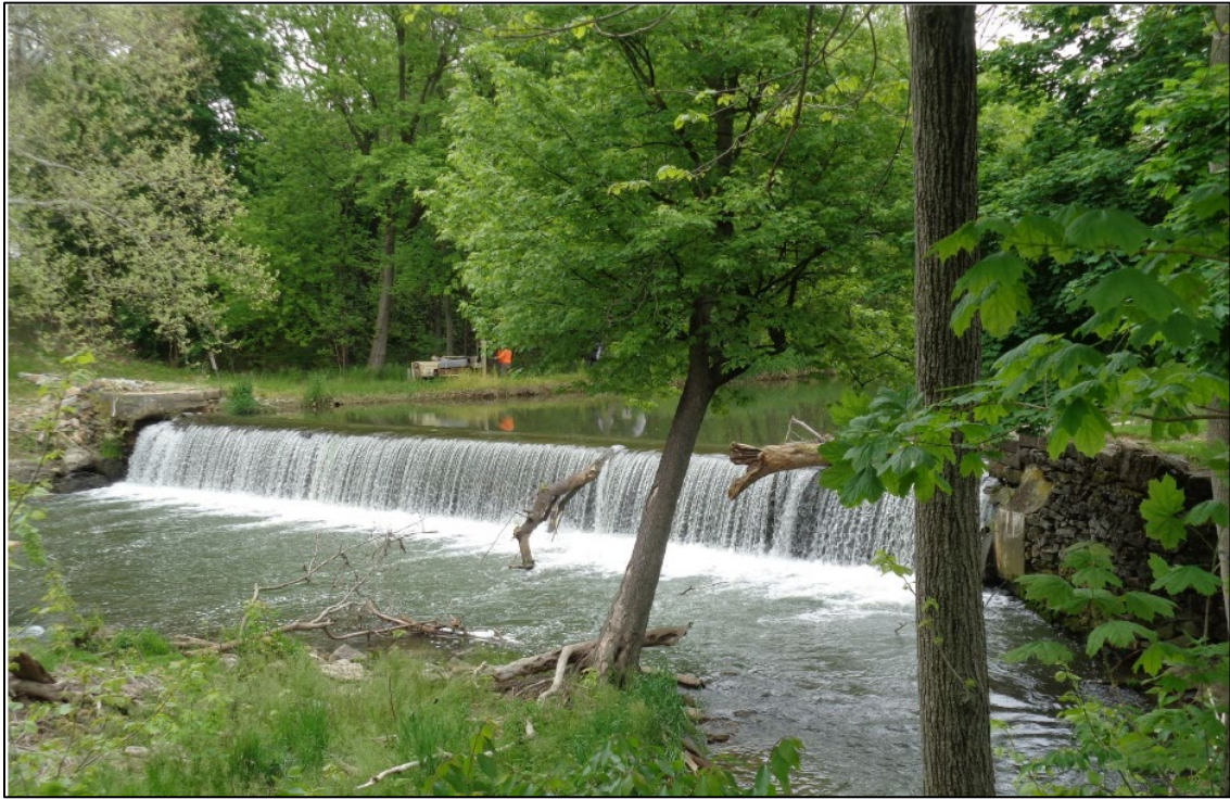
Figure 2.1 Chiques Roller Mill Dam Photo 1
