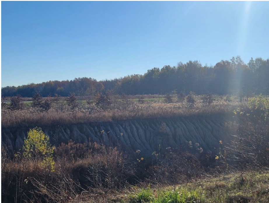
Photo: Erosion on Cypress Ditch, Conservation Works Joint Venture 12/7/2023
