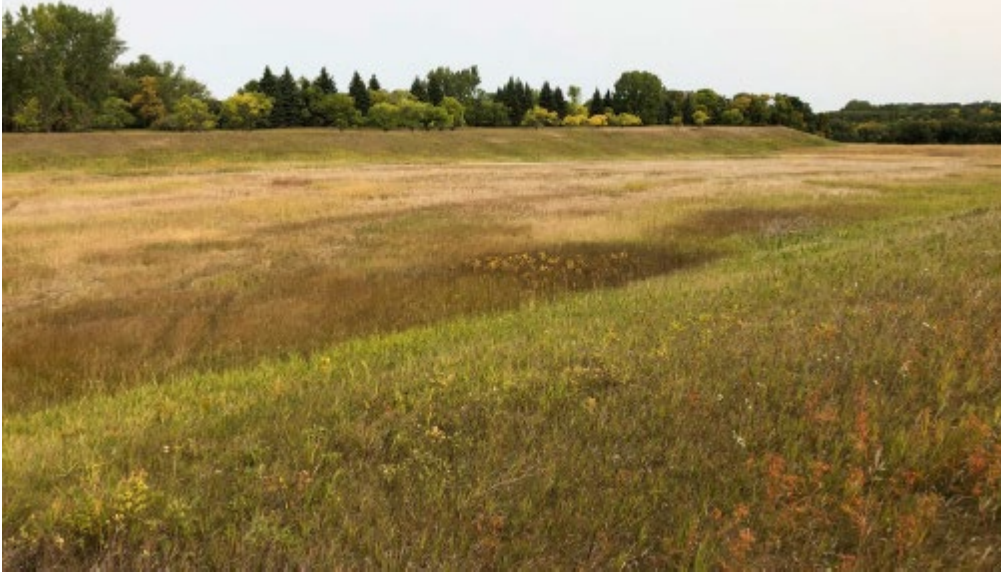
Figure 4 Tame grassland on auxiliary spillway
