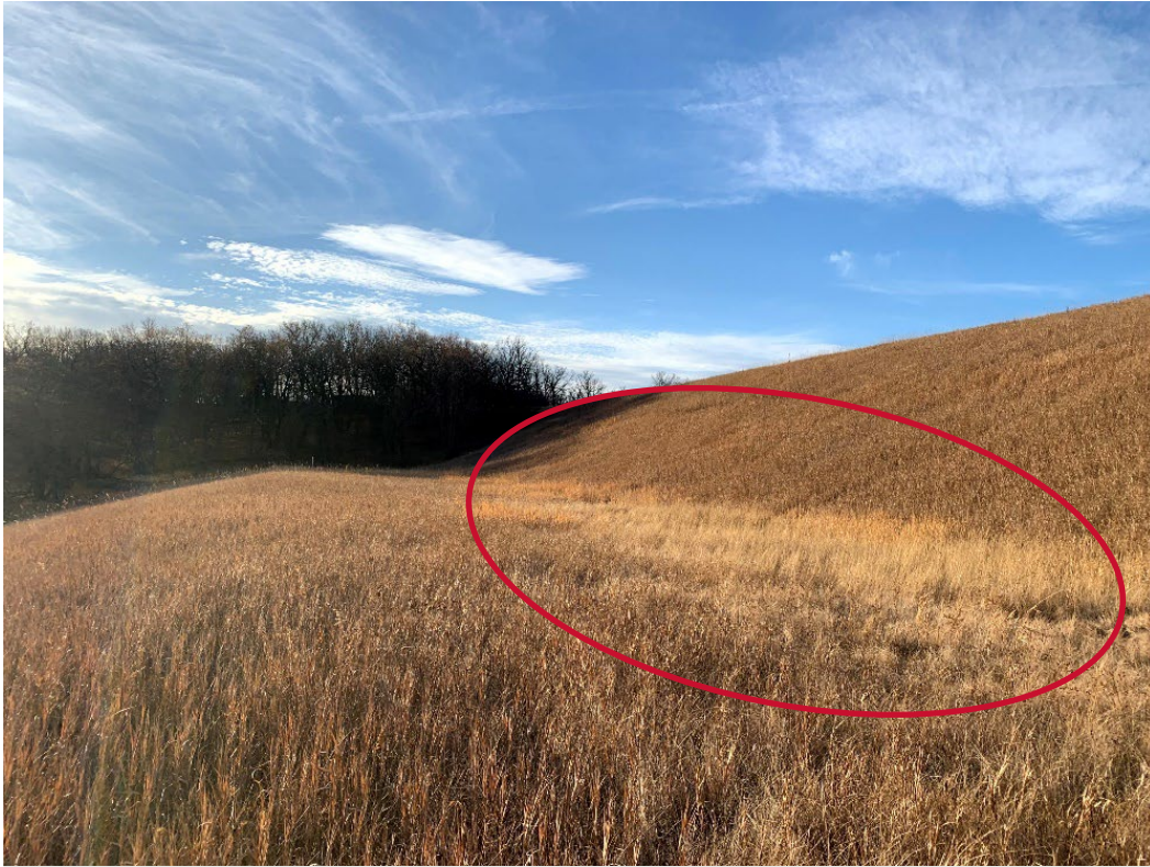
Photo 15: Wetland vegetation on downstream berm, looking south.
