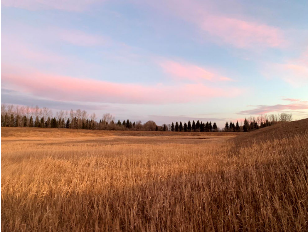
Photo 19: Auxiliary spillway, looking north.
