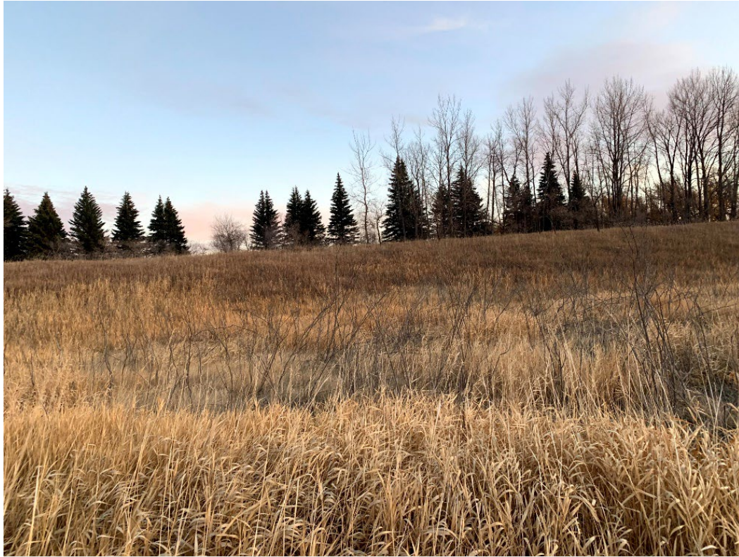
Photo 25: Woody vegetation, auxiliary spillway.
