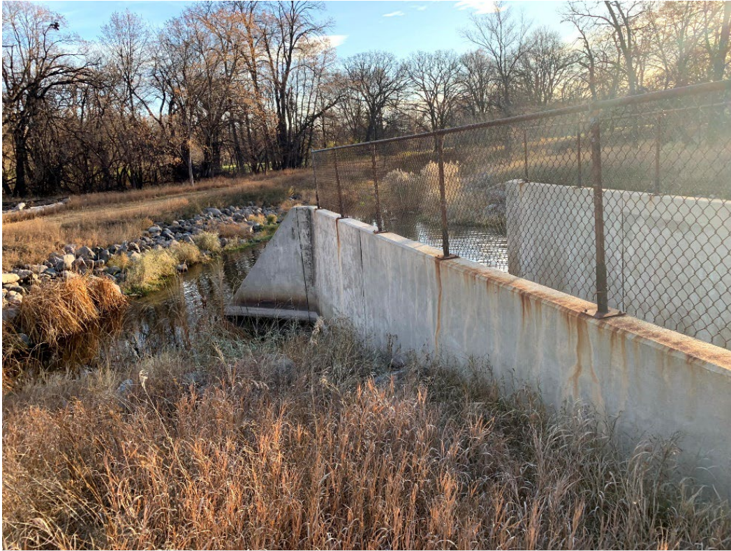
Photo 6: Left side of principal spillway outlet.
