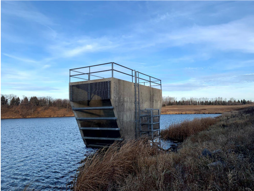
Photo 2: Principal spillway inlet, looking northwest.
