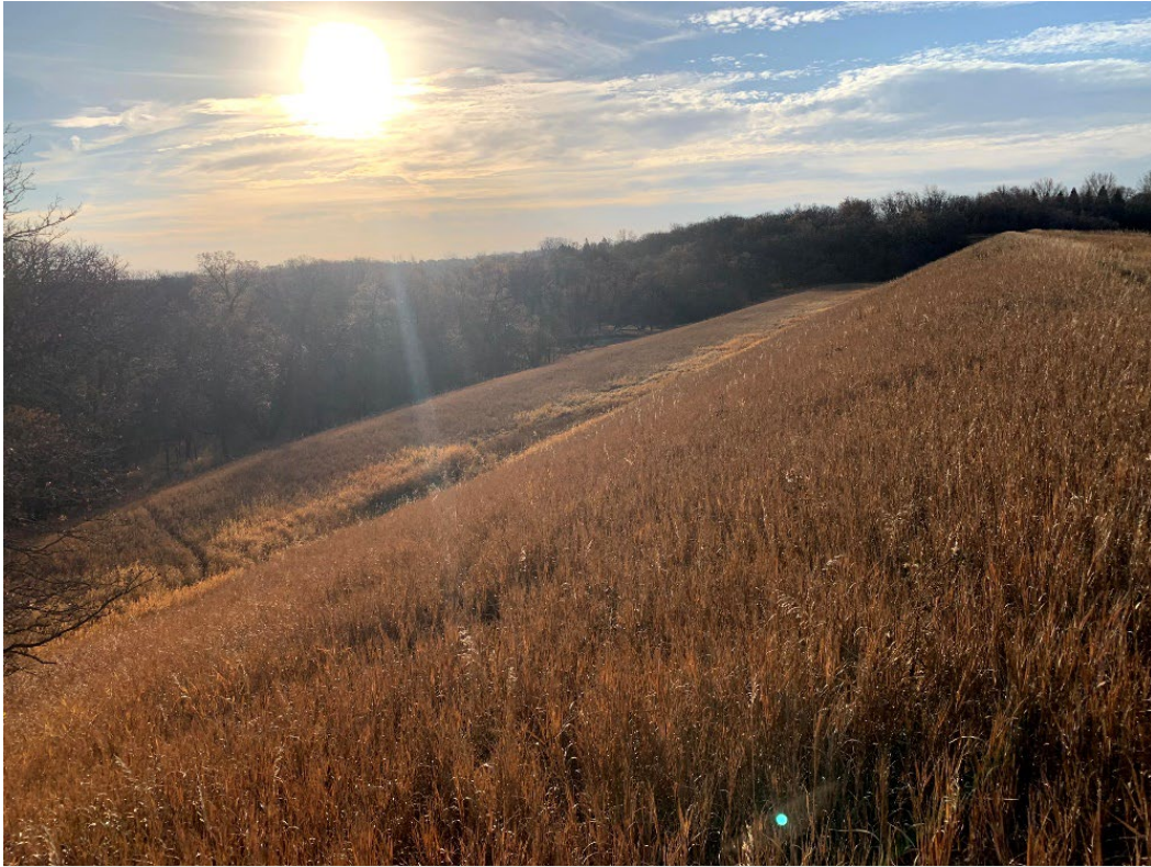
Photo 14: Downstream slope, looking south.
