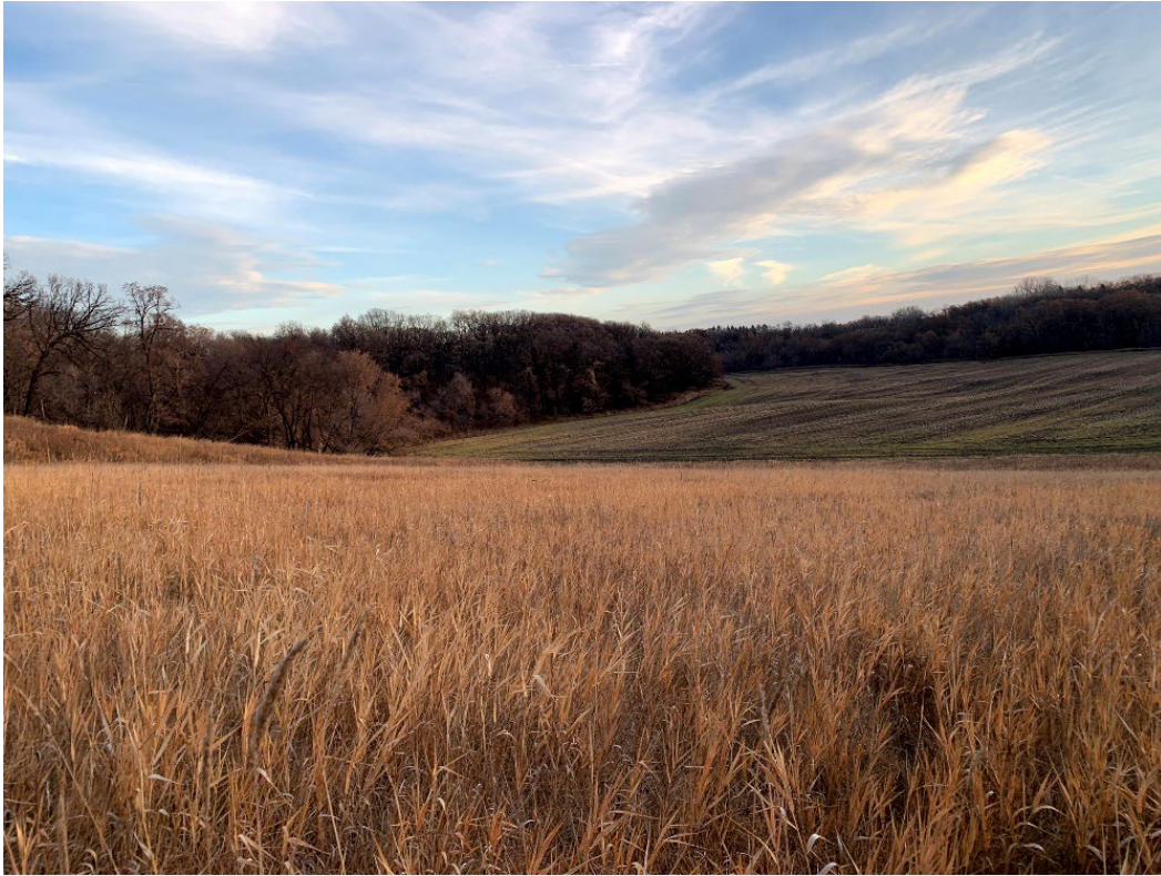
Photo 22: Exit section of auxiliary spillway, looking east.
