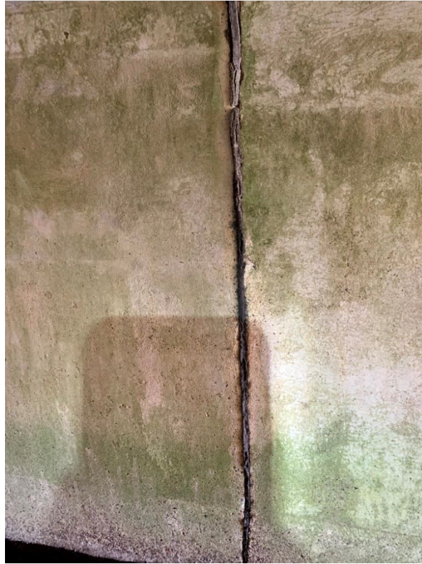
Photo 29: Joint filler, Joint #2.
