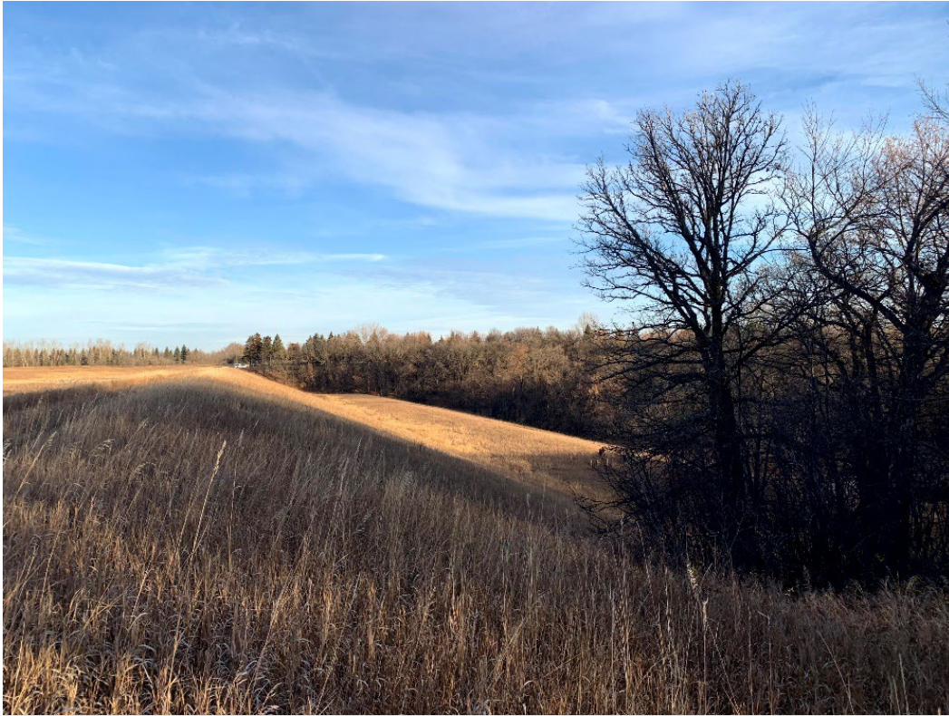
Photo 13: Downstream slope with trees in right abutment, looking north.
