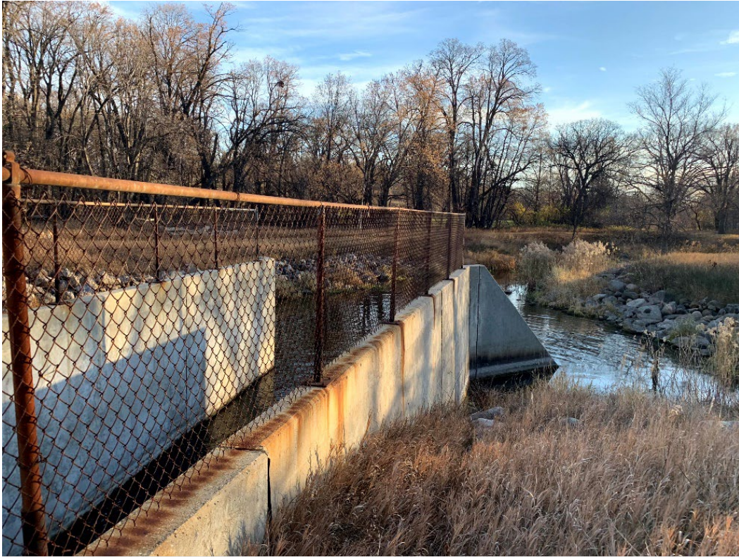
Photo 7: Right side of principal spillway outlet.
