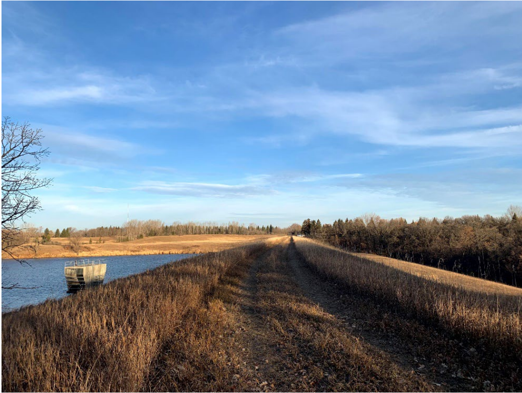
Photo 17: Crest of dam, looking north.
