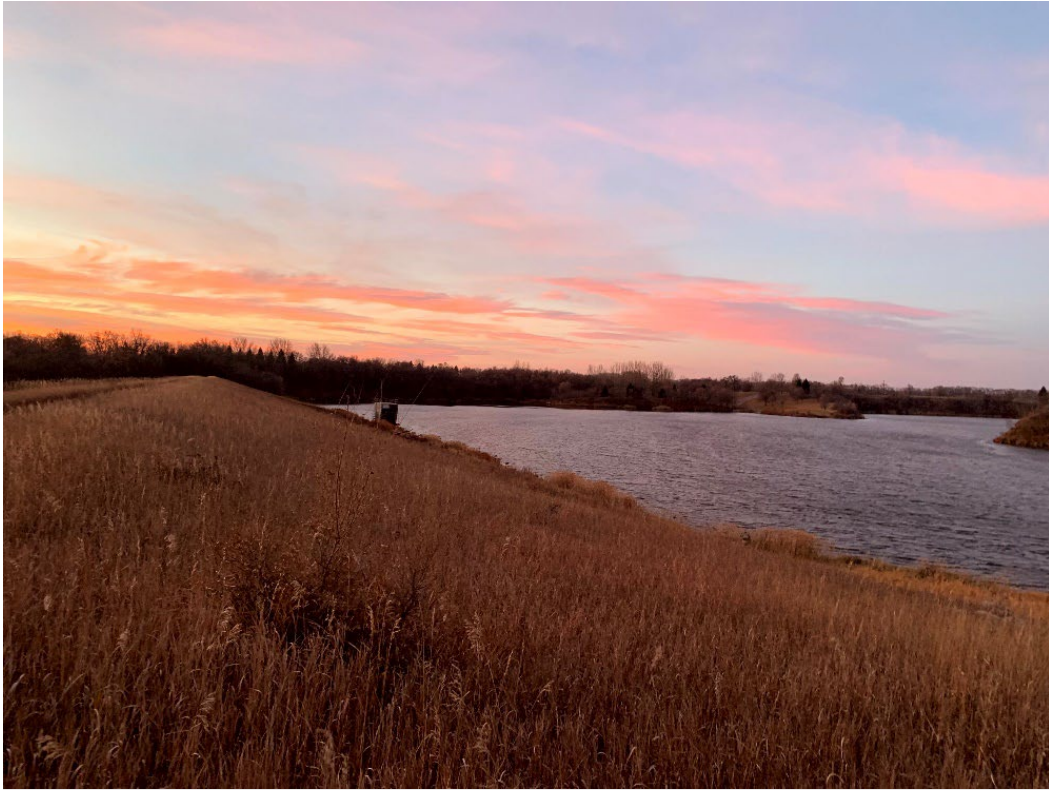
Photo 10: Upstream slope, looking south.
