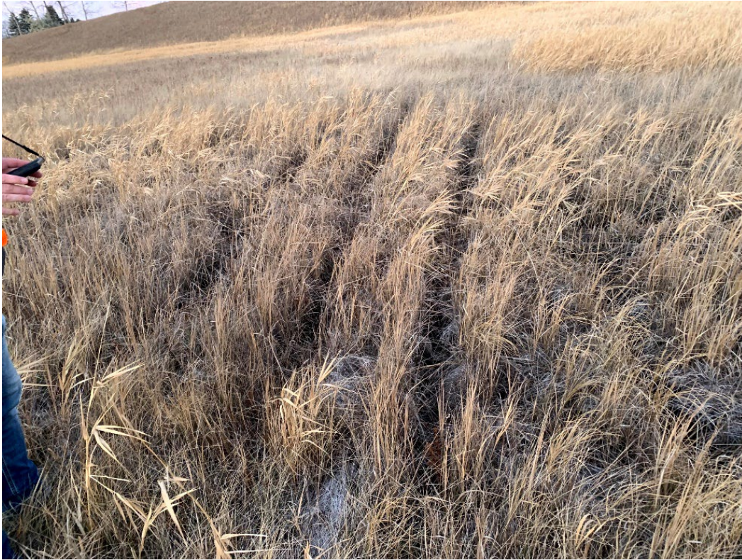
Photo 24: Rutting from ATVs, auxiliary spillway.
