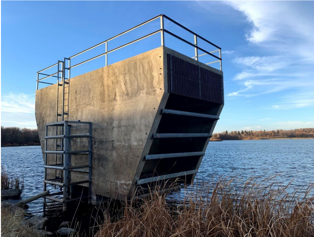
Photo 1: Principal spillway inlet, looking southwest (note water level, above crest of weir).
