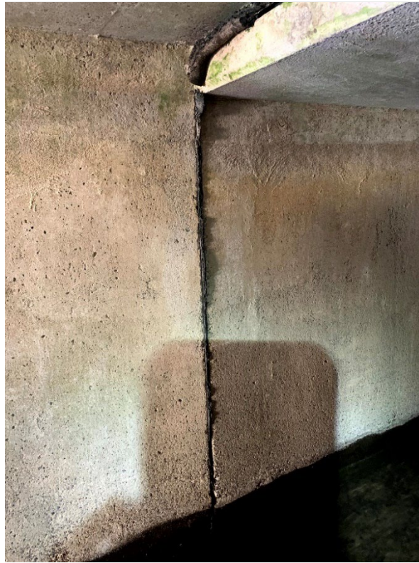
Photo 30: Joint filler, Joint #3.
