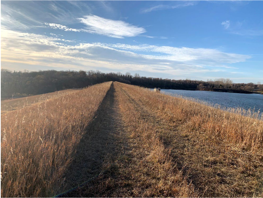
Photo 18: Crest of dam, looking south.
