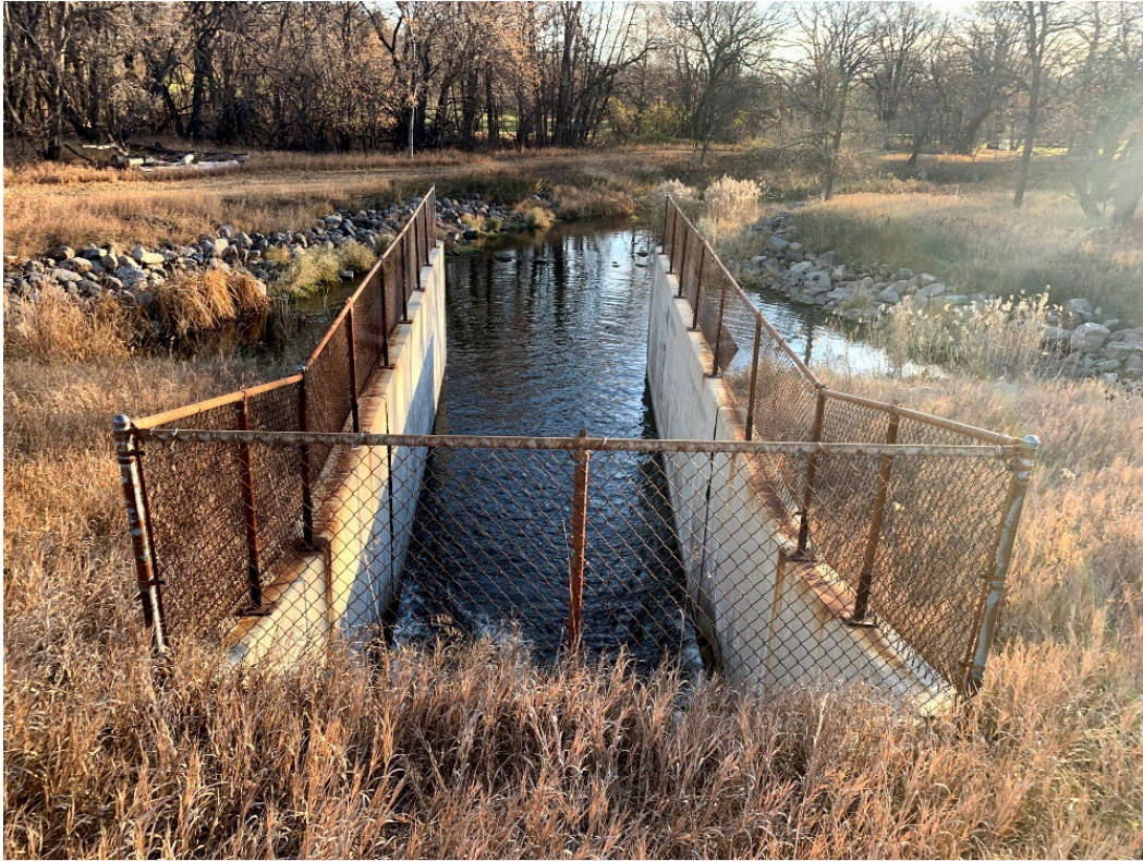
Photo 4: Principal spillway outlet, looking east.
