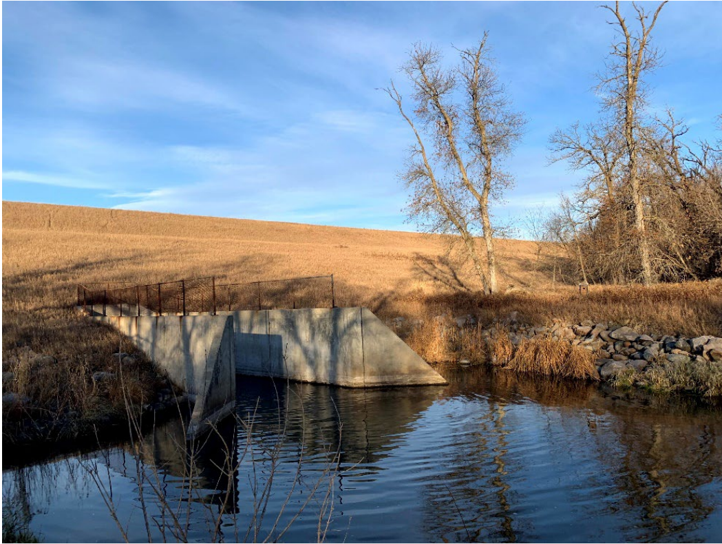
Photo 5: Principal spillway outlet, looking northwest.
