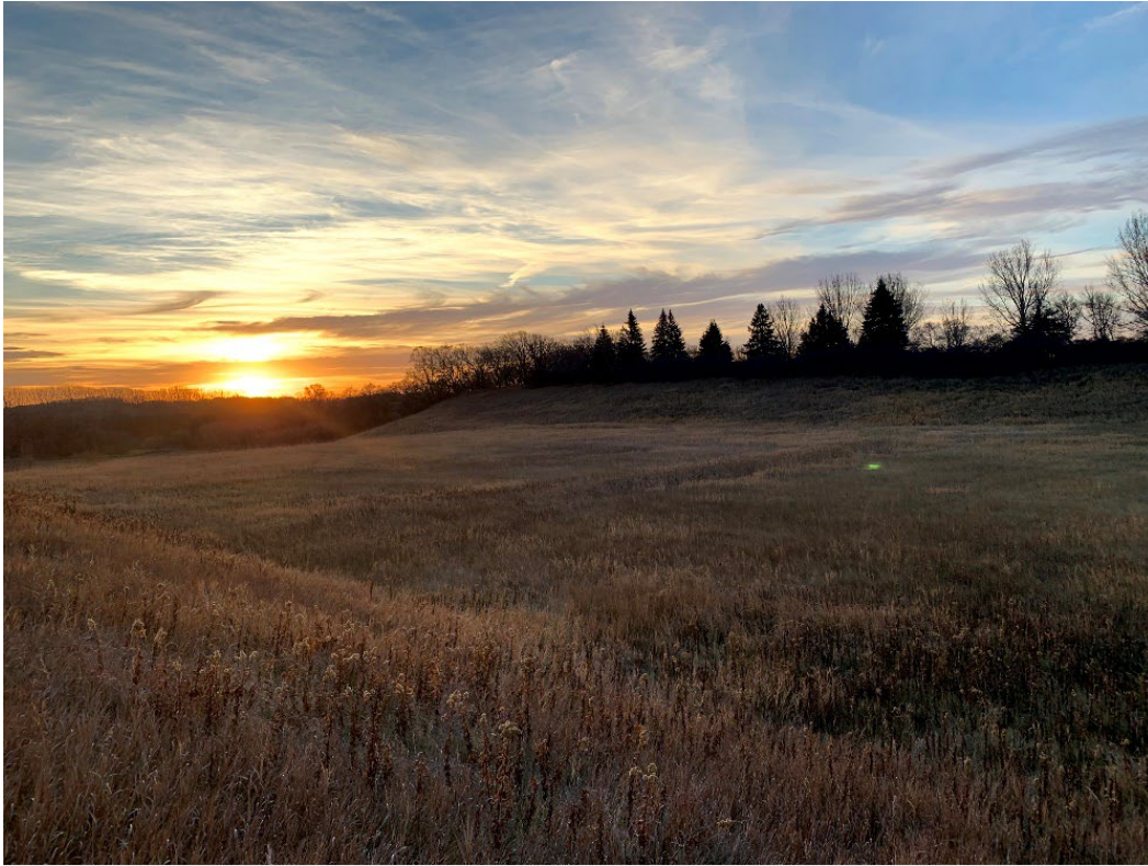
Photo 21: Auxiliary spillway, looking southeast.
