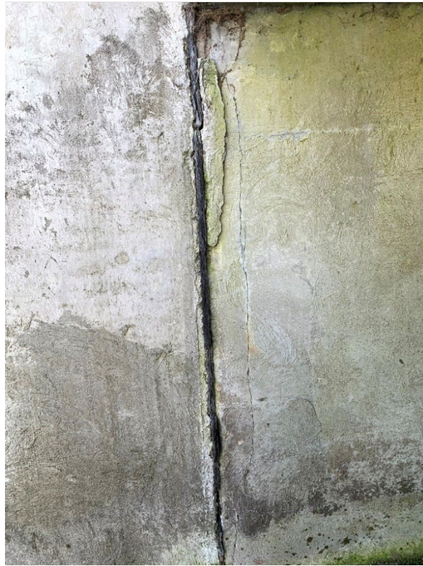
Photo 28: Cracking, Joint #1.
