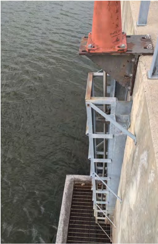
Figure 21 Larimore Dam Primary Inlet and Riser
