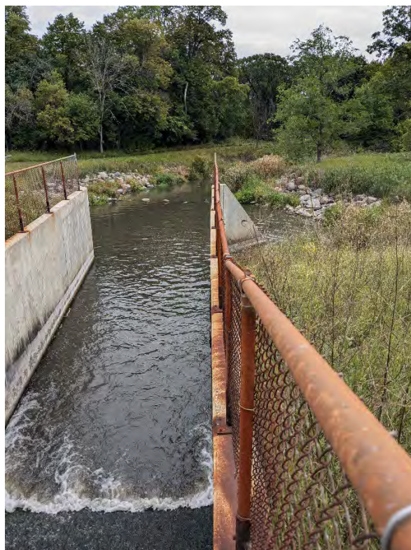
Figure 19 Larimore Dam Outlet structure looking east
