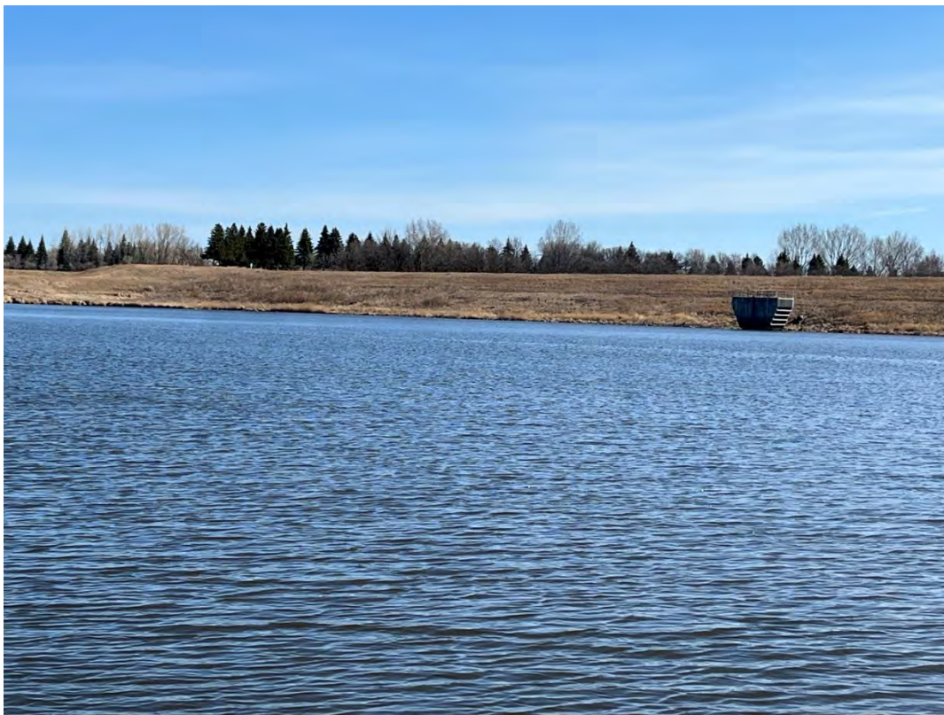
Figure 17 Larimore Dam Secondary Intake 2/29/2025
