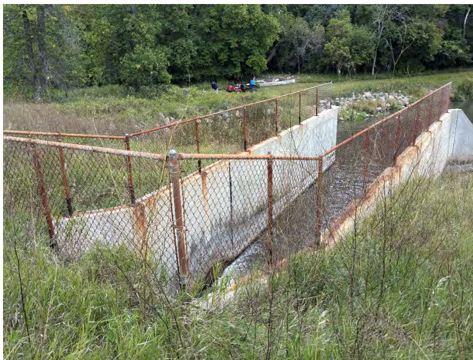
Figure 18 Larimore Dam Concrete Outlet structure - looking northeast
