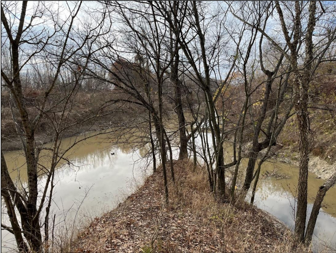
Figure 10. Overview of ditch system, facing S, taken from the terminus of the eastern berm of Cypress Lateral Number 1 in right foreground, Lick Creek in left foreground, St. Francis River in center background.
