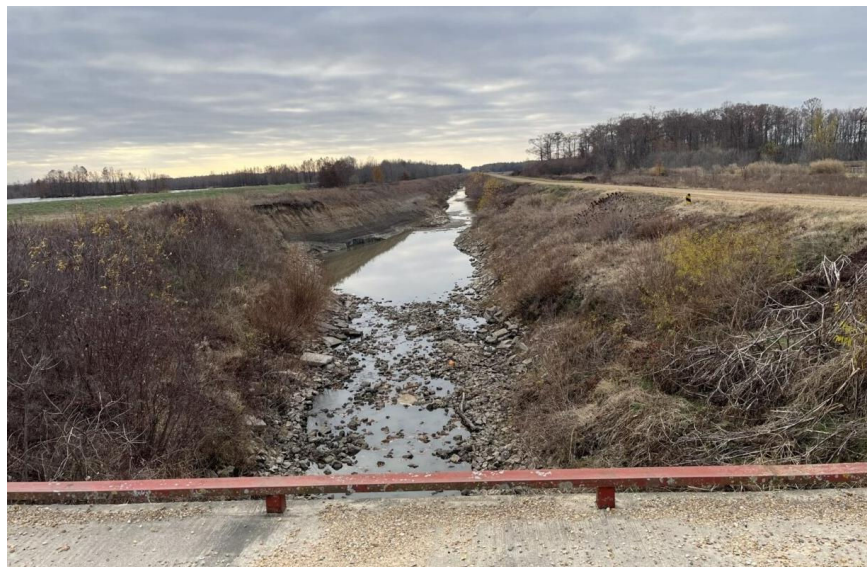
Figure 16. Overview of Cypress Lateral No. 1, View South from the Concrete Bridge (Structure No. 21905) at County Road 679 (Source: Terracon 2023).
