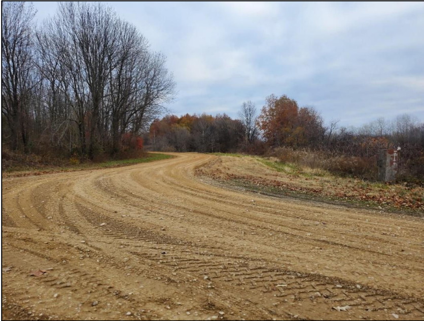
Figure 8: Evidence of disturbance to previously recorded site 23S0411 (bisected by road), facing N/NE, taken from intersection of split of Co. Rd. 691 and campsite turnoff.
