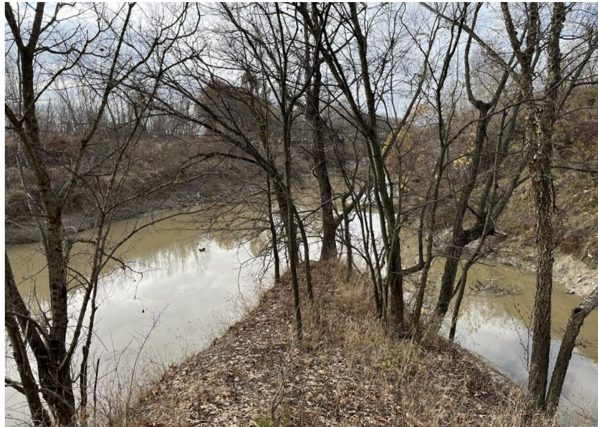
Figure 17. Junction between Cypress Lateral No. 1 and Sublateral Ditch near Feature K.
