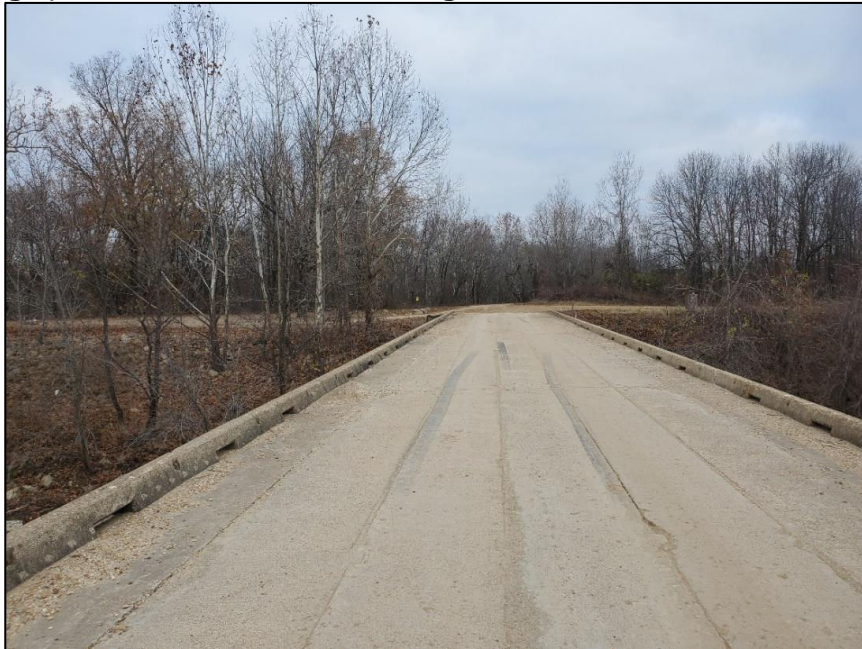
Figure 16. Co. Rd. 691 bridge across Lick Creek at southern end of the APE, facing NW, taken from bridge.
