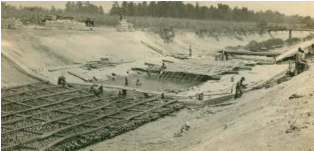
Figure 8. Construction of a Drainage Ditch in the Little River Drainage District (Stephens et al. 2008).
