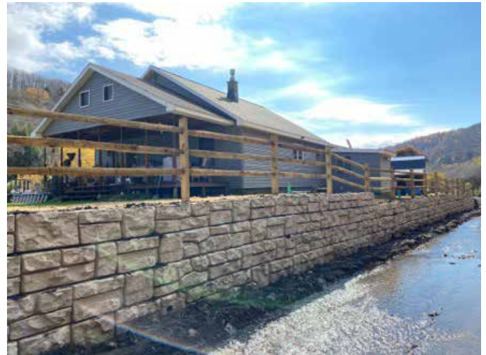
After: The streambank was stabilized through NRCS's Emergency Watershed Protection (EWP) Program.
