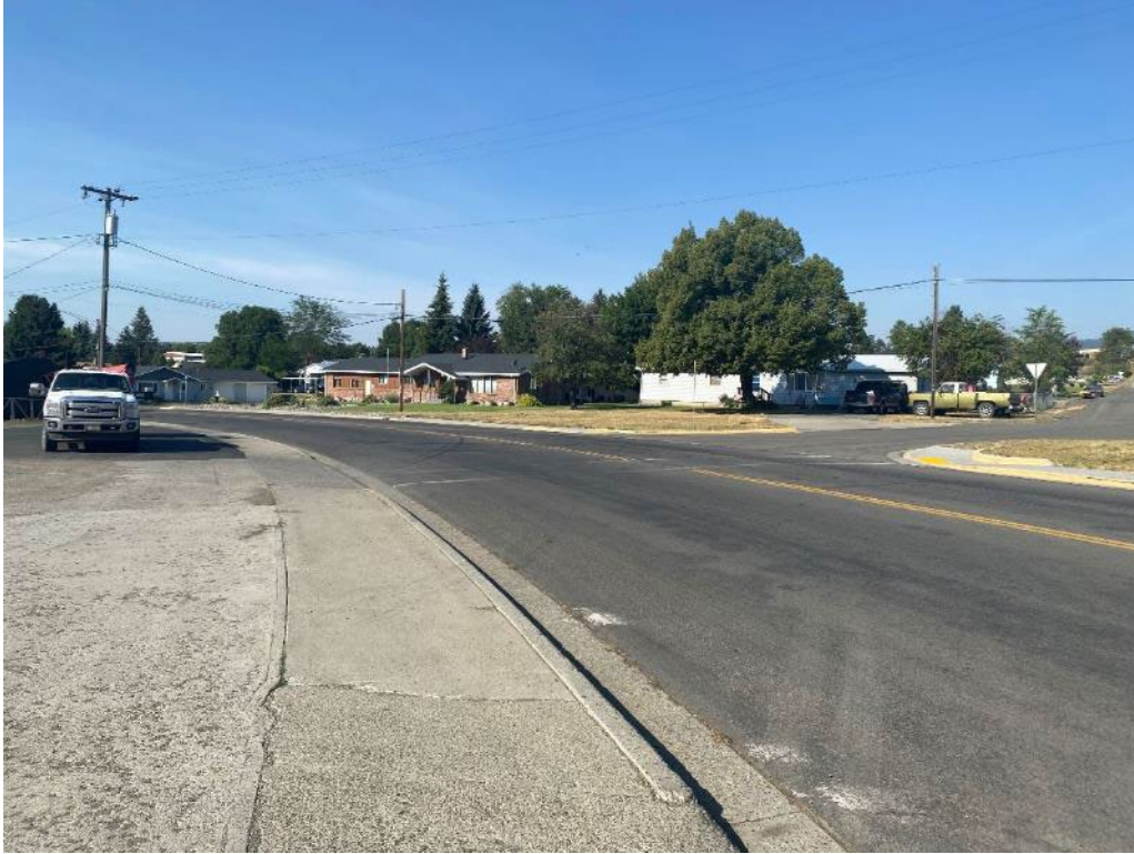
Photograph 3: South view of City of Cottonwood along Business US-95/King Street
