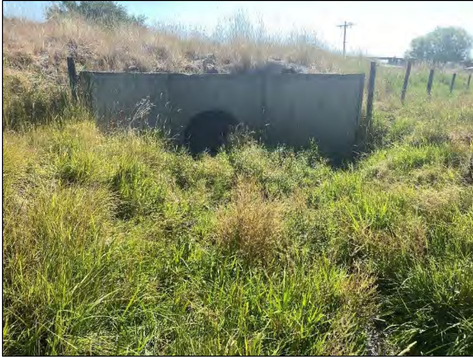
Photo 3: East view of Cottonwood Creek and culvert
