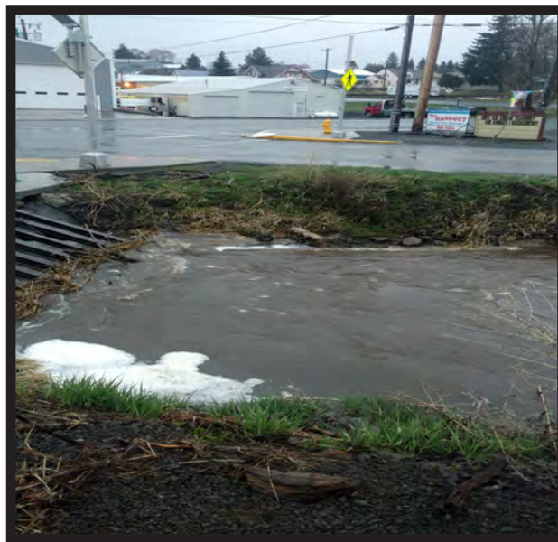
Lewiston Street Headwall
