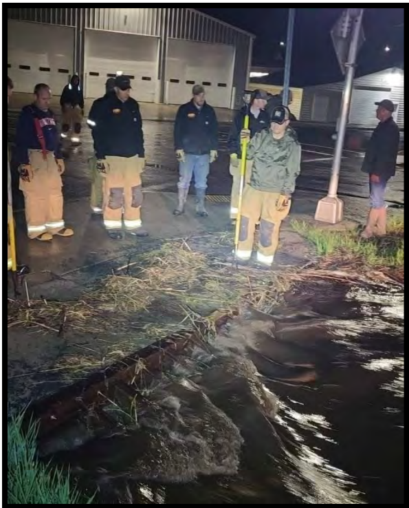
Lewiston Street Headwall and Grate
