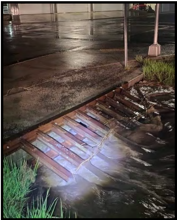
Lewiston Street Headwall and Grate
