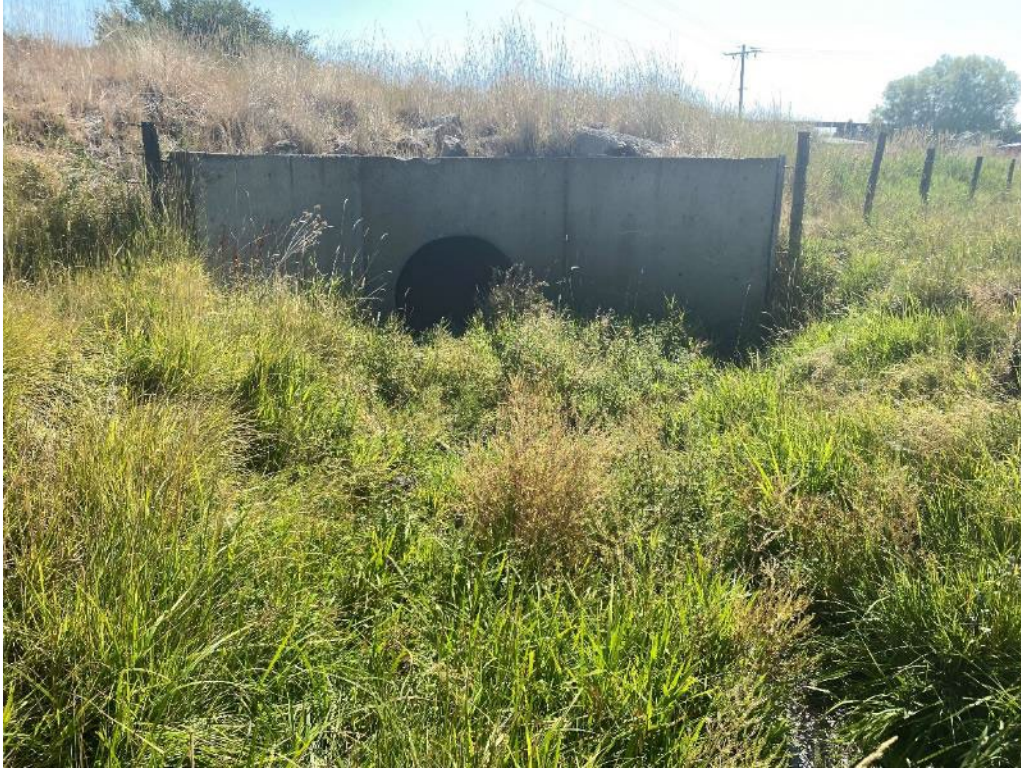
Photograph 5: East view of Cottonwood Creek and culvert, near Wetland 1
