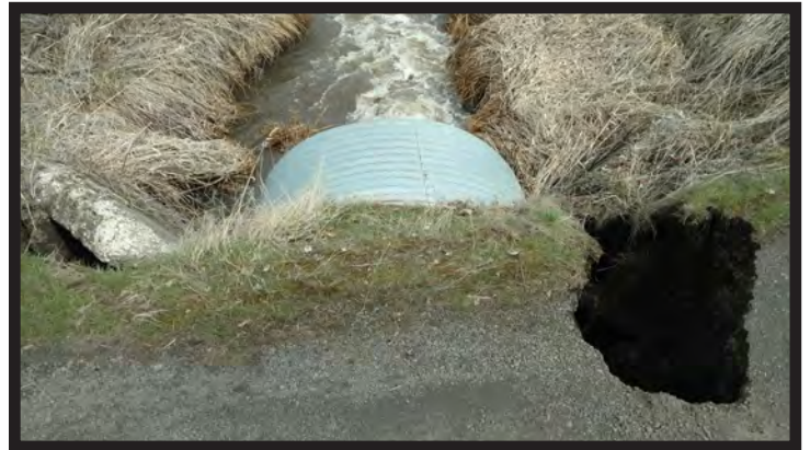
Front St. Culvert Hole
