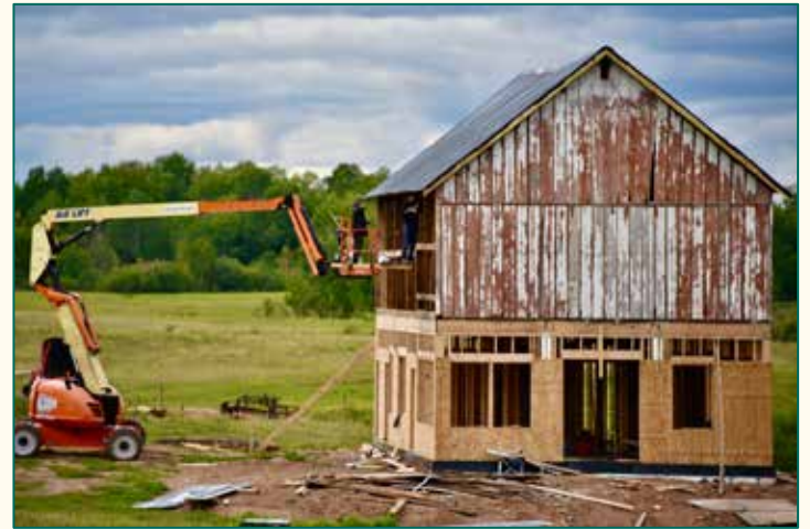
1880's Timber Frame Barn
