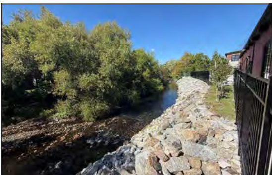
Completed streambank stabilization at United Way in Providence.
