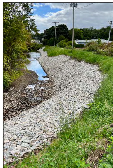
Woonasquatucket River streambank stabilized with riprap, erosion control blankets, and vegetation.
