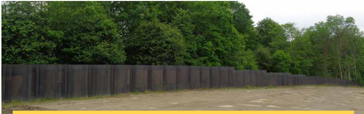
Regraded auxiliary spillway and new sheetpile training wall at Thatcher Run PA-112, Conneautville Dam.
