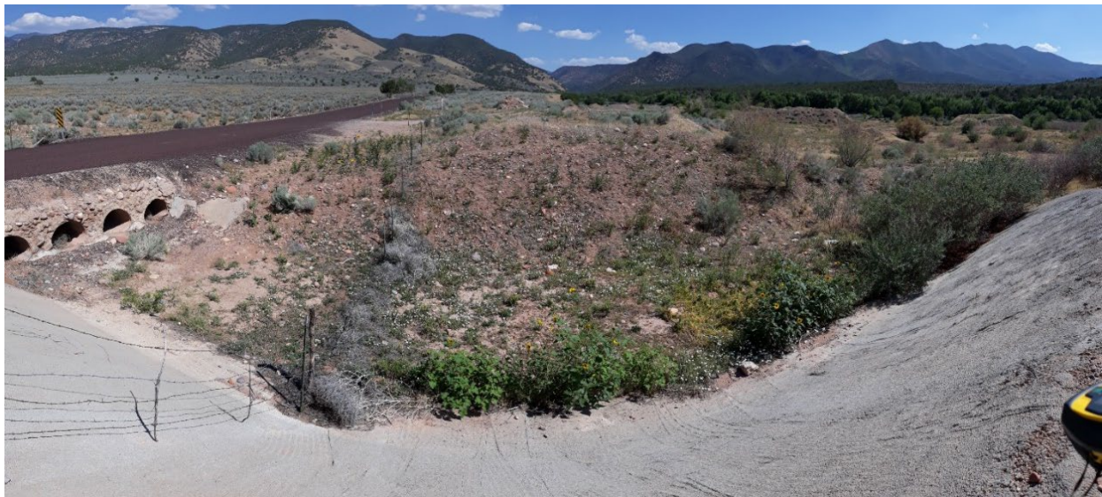
Figure 3-9: Emergency Spillway Culverts Upstream End
