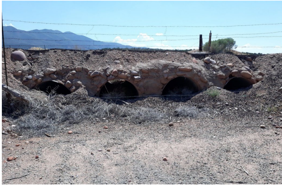
Figure 3-10: Downstream Side of Emergency Spillway Culverts
