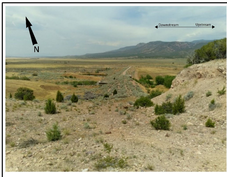
Figure 3-2: Dam Embankment – West End View
