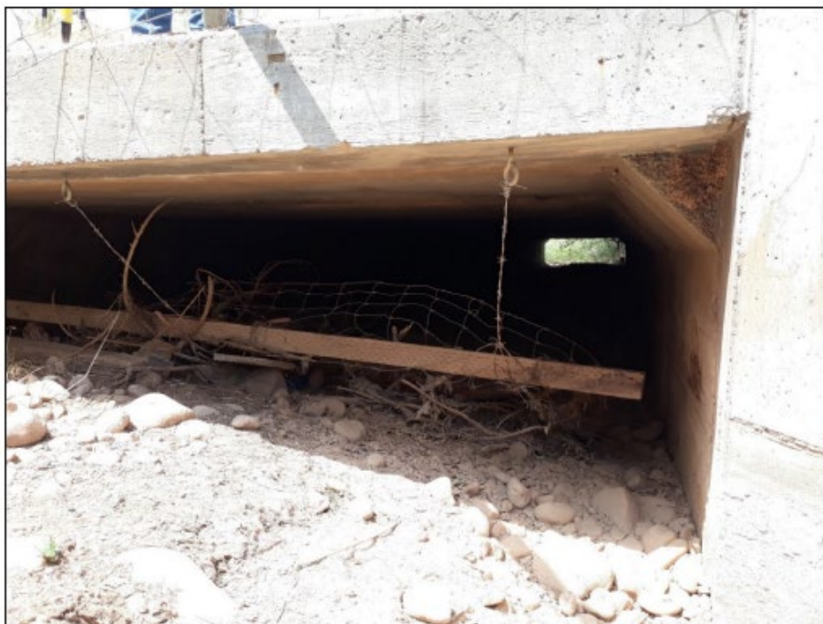
Figure 3-15: Box Culvert Crossing at Highway 133
