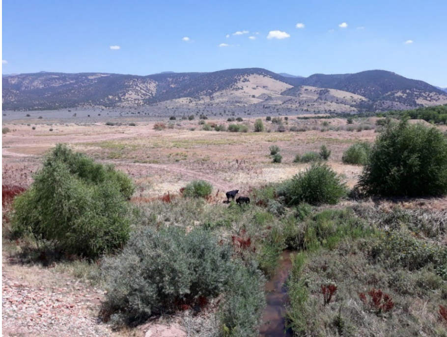
Figure 3-4: Debris Basin and Corn Creek – View from above the Spillway
