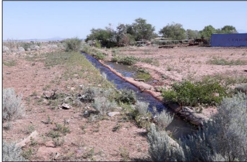
Figure 3-12: Leakage from the East Middle Hatton Ditch with Flow Approximately 3 cfs
