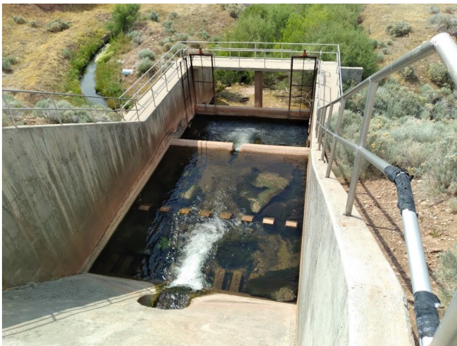
Figure 3-7: Primary and Secondary Spillway Stilling Basin
