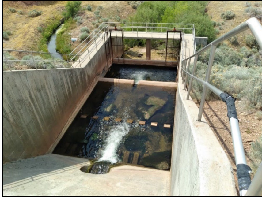
Figure 2: Outlet Works Stilling Basin, June 2021
