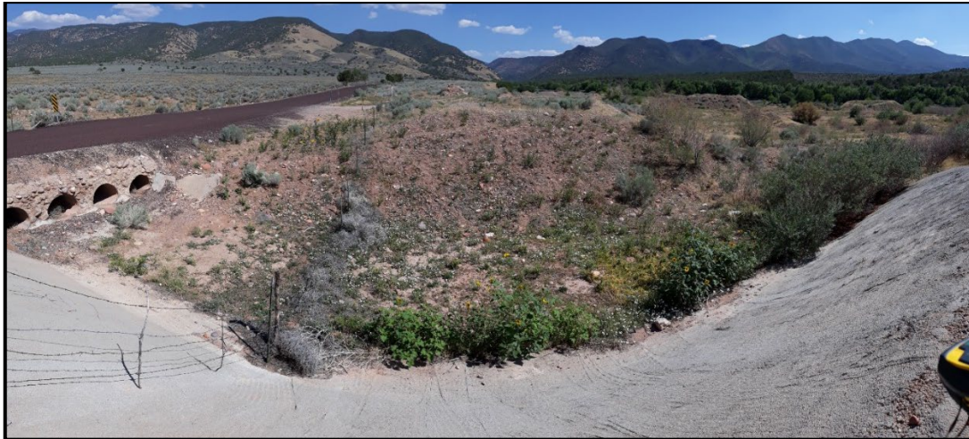
Figure 3: Emergency Spillway and Flood Channel, July 2021
