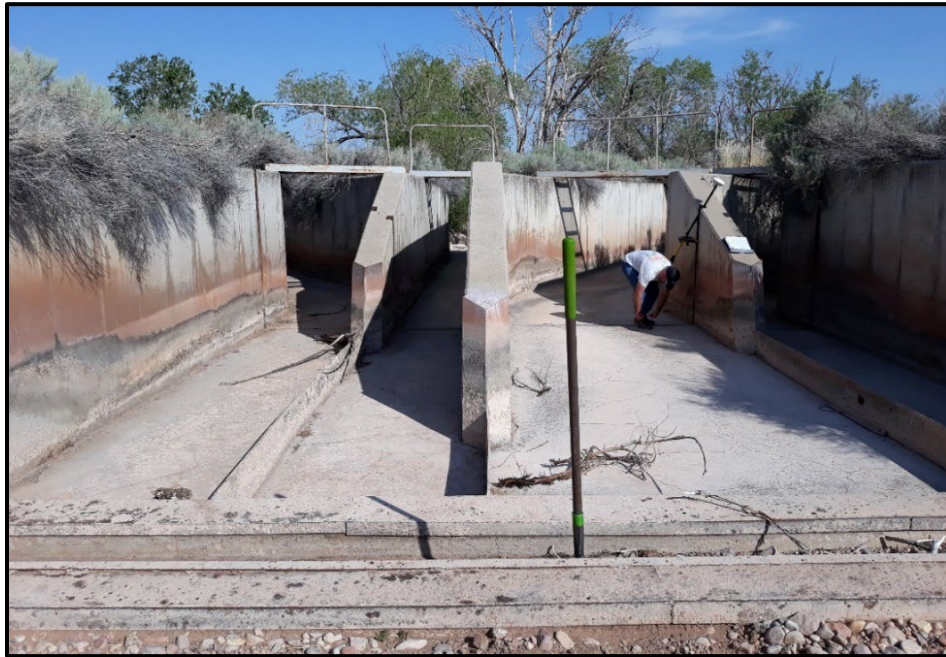
Figure 5: Diversion Structure, July 2021
