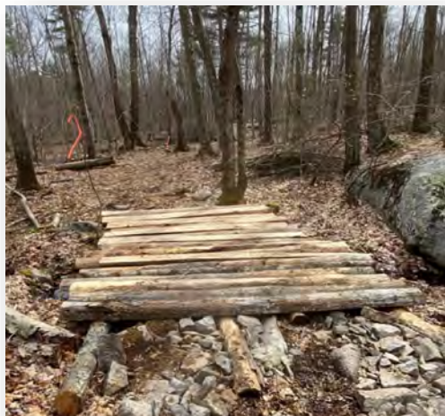
Forest Trails/Landings (Temp. Stream Crossing)
