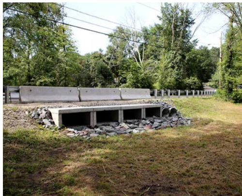
The roadway was raised to allow safe access and a box culvert was installed to allow storm water to flow under the road and back to the Pocasset River. (AFTER)
