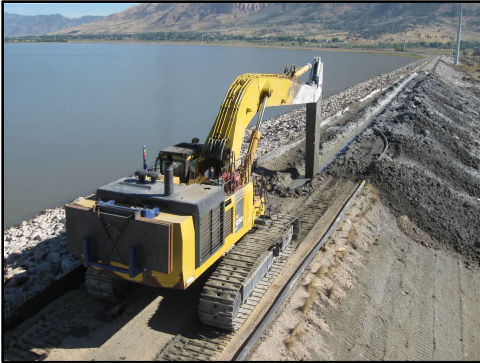
Figure 22: Photo of HydroMill Installation of Cutoff Wall
