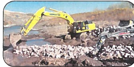
Streambank Grade Stabilization: Moreau River Stream Barbs
