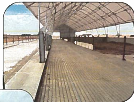
(Location and inside- look at the bedded pack barn with the hoop roof installed.)
