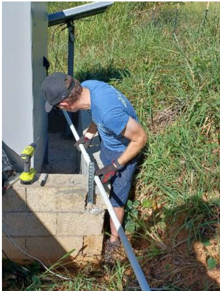
Tubing installation for Water sampler
