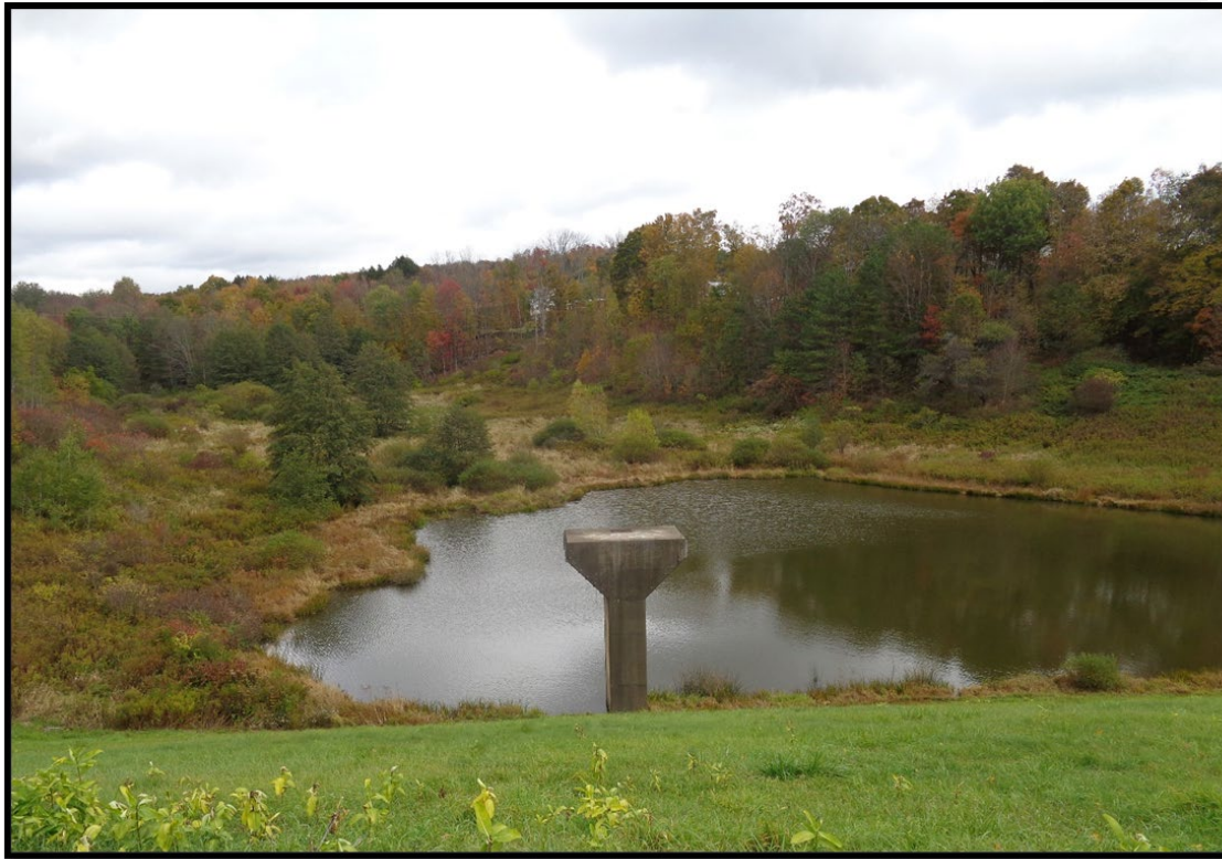
PA-467 Kingsley Dam Photo courtesy of NRCS
