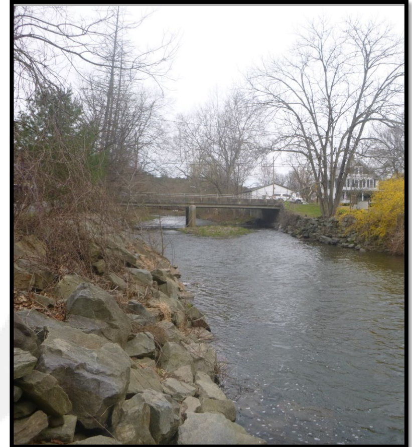
Martins Creek and State Street Bridge
