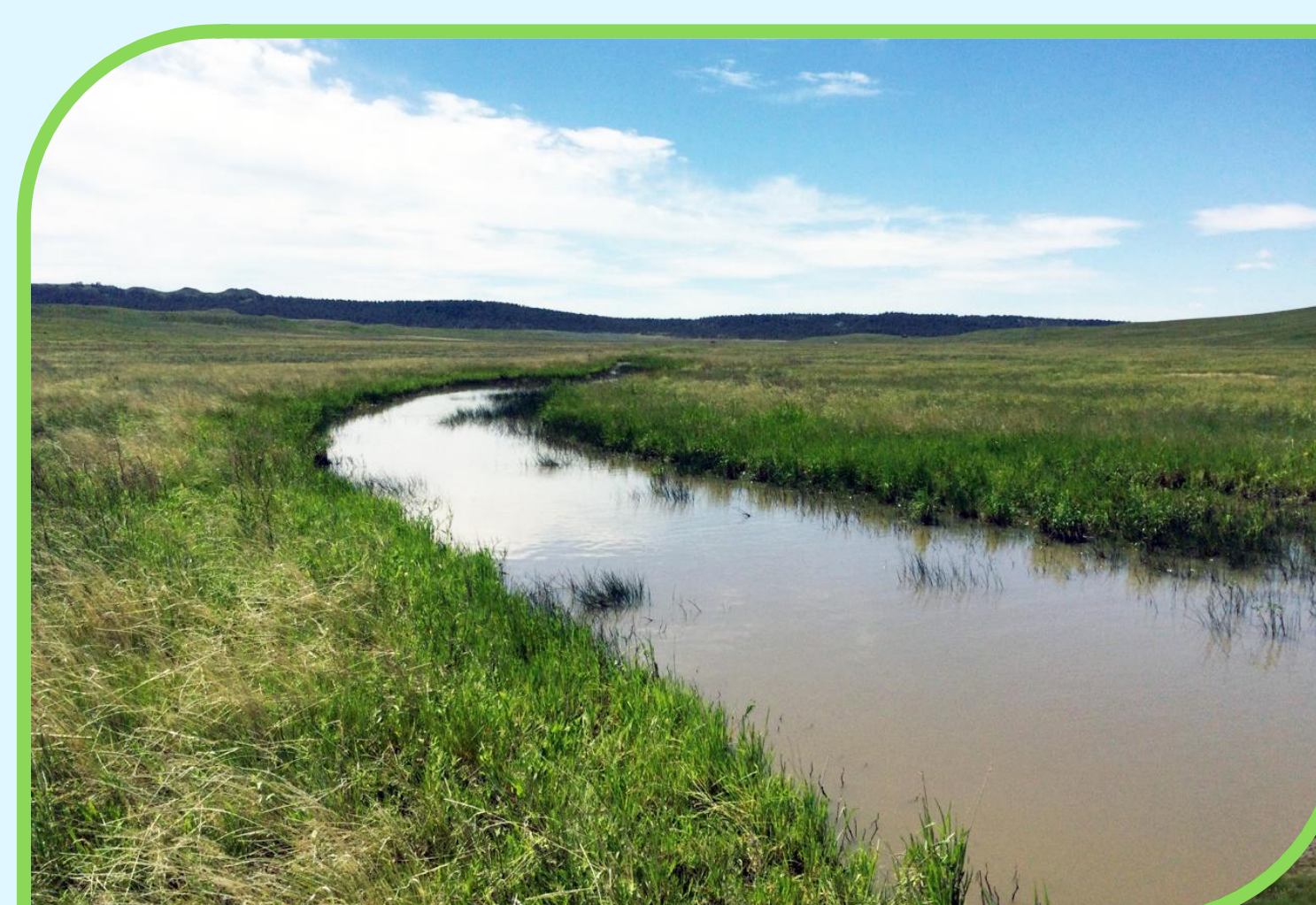
Little Suction Creek showing pooling water at failed portion of diversion structure
