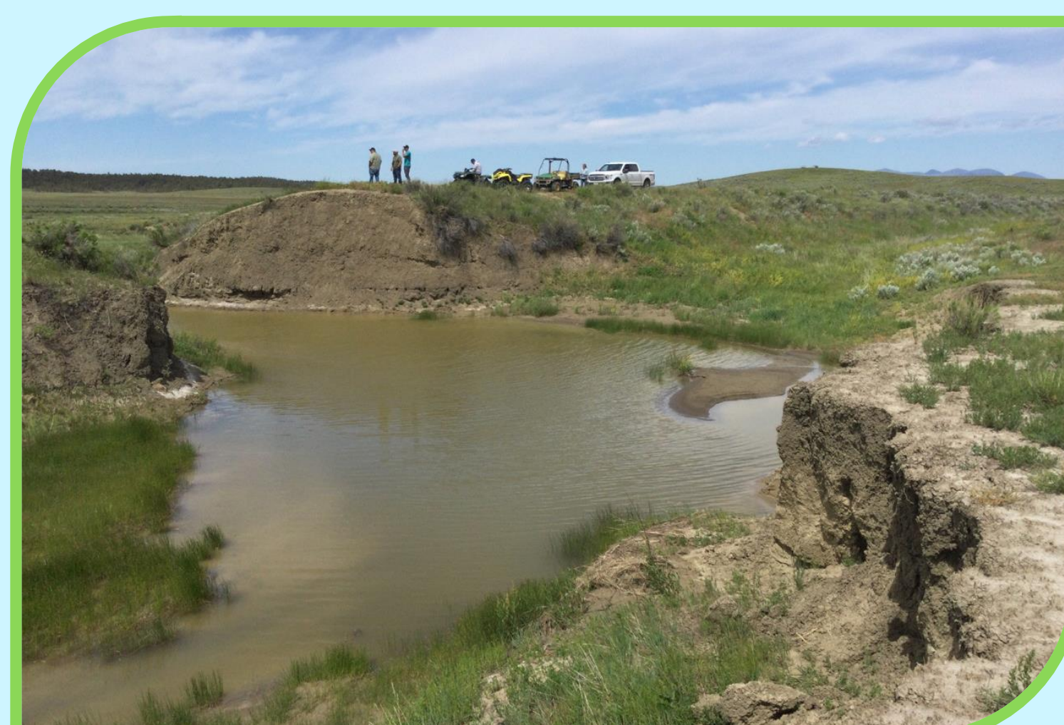
Little Suction Creek looking downstream toward the diversion structure
