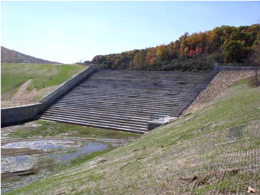
Figure 2 - Example of a Roller-Compacted Concrete Auxiliary Spillway
