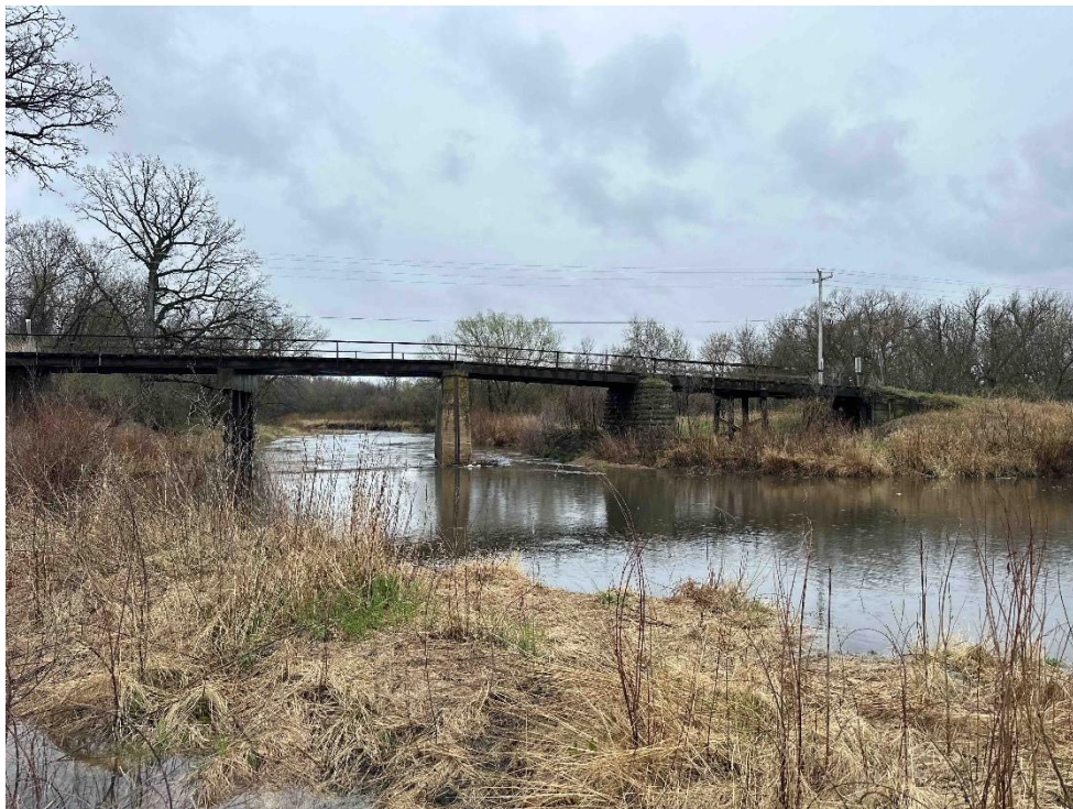
Photo 8 – Bridge over the Upper Iowa River – View to the South.
