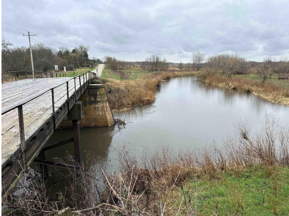
Photo 1 – Project Overview along the Upper Iowa River – View to the North.
