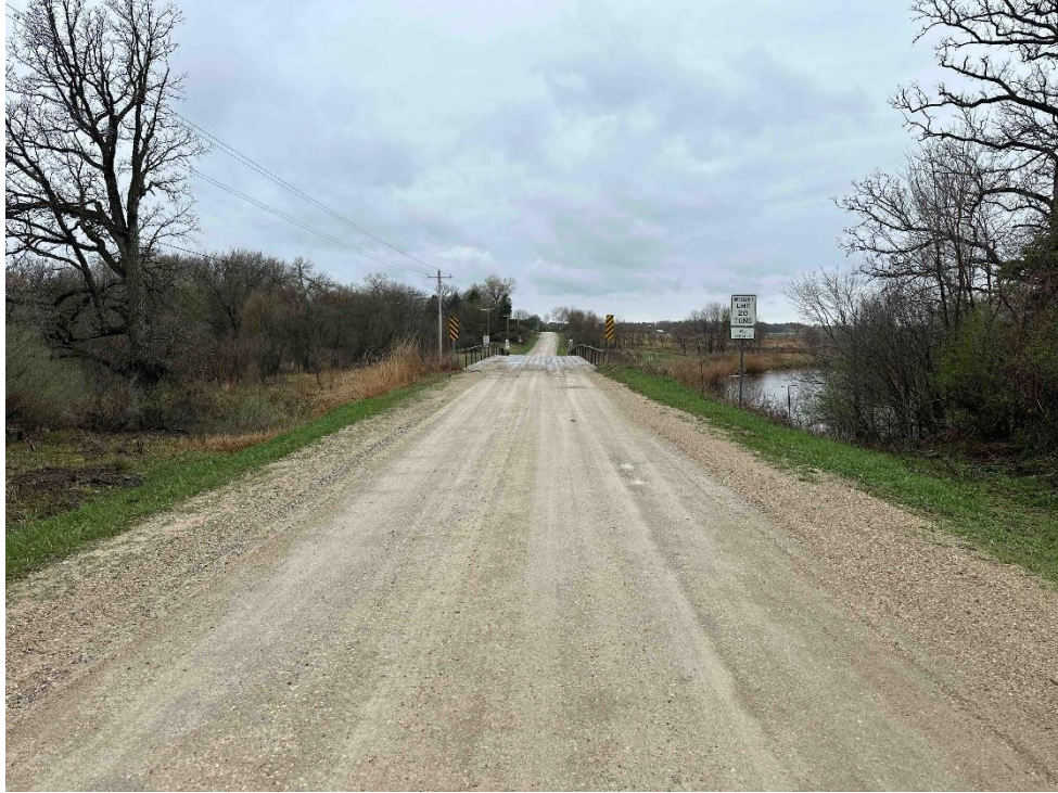
Photo 3 – Project Overview along 25 th Avenue – View to the Southwest.
