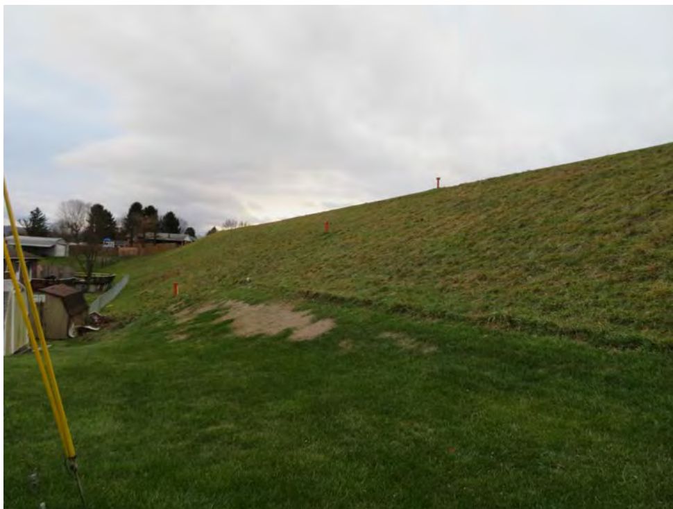
Photo 7: Downstream embankment slope, looking southwest.
