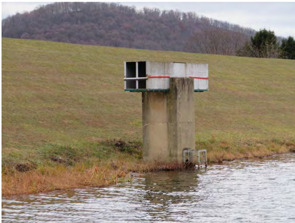
Photo 6: Principal spillway riser structure, looking south.
