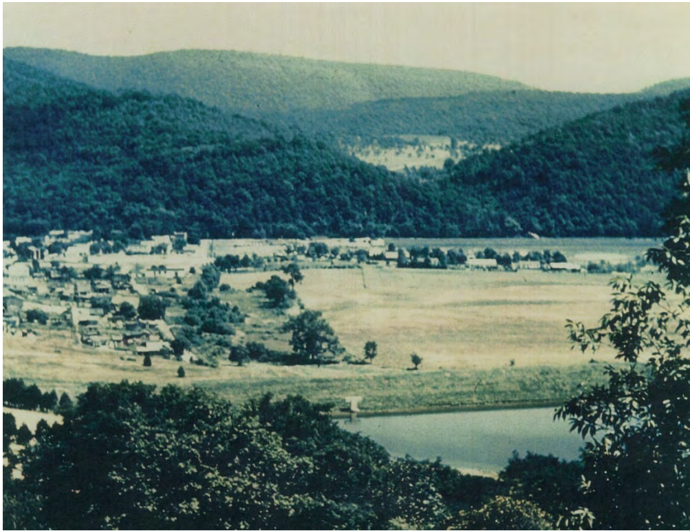
Figure 2- Aerial view of New Creek Site 1 sometime after construction.
