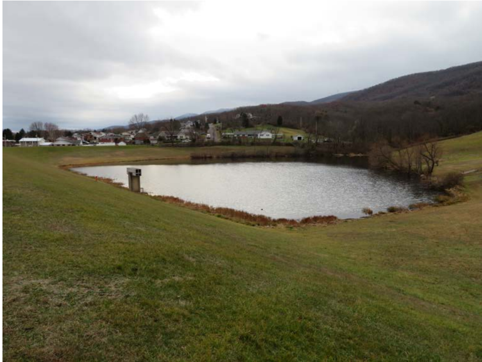
Photo 2: Reservoir, looking southwest.
