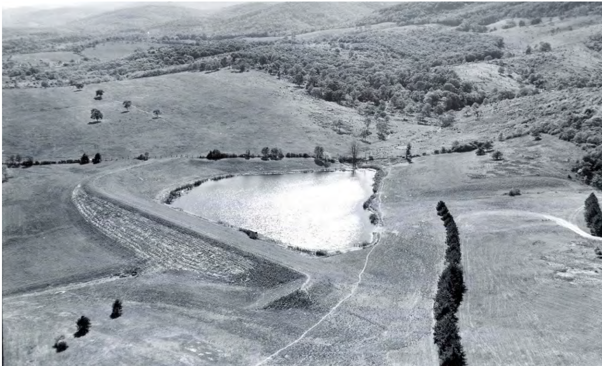
Figure 1 - Aerial View of New Creek Site 1 Following the Original Construction in 1957.
