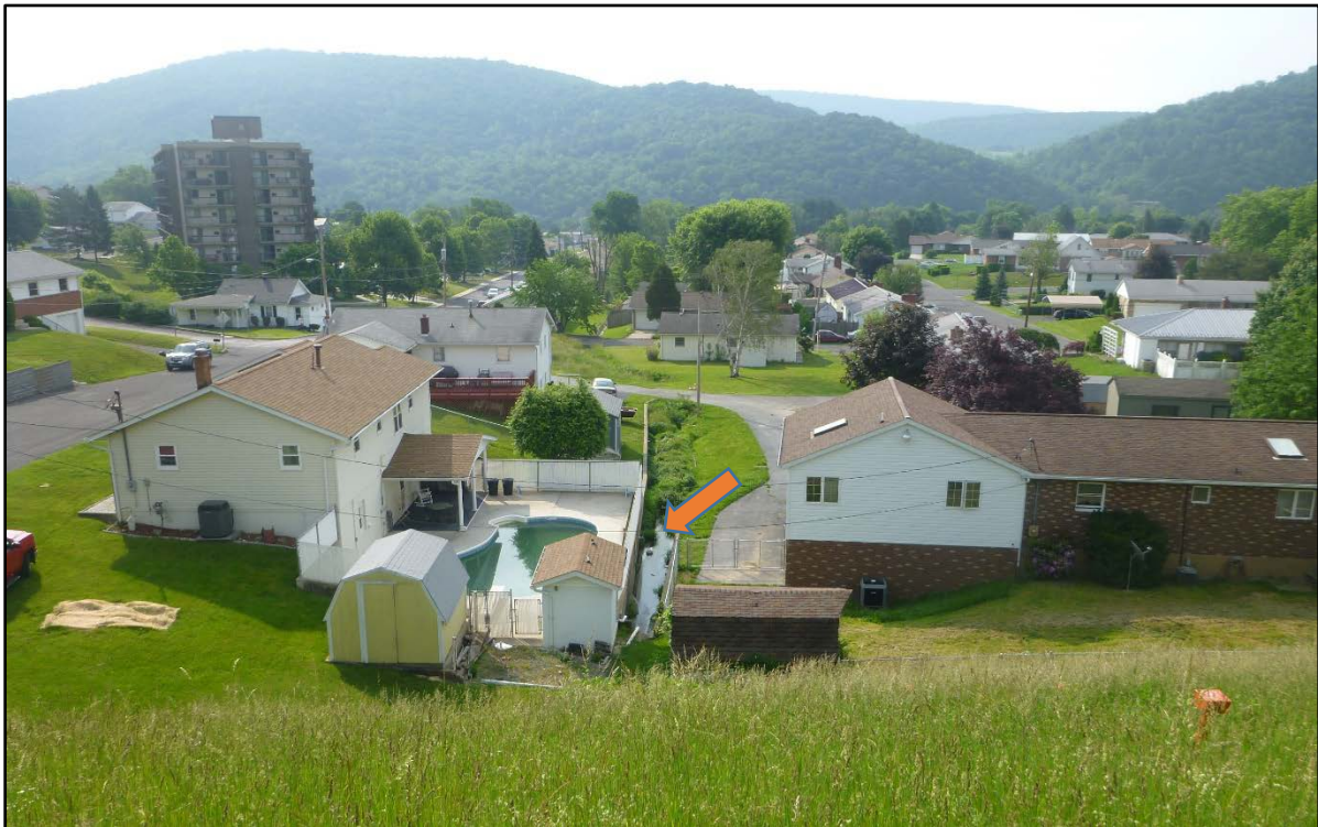
Looking southeast from top of New Creek Site 1 embankment – Carskadon Lane to left. Principal spillway outlet channel noted by arrow.
