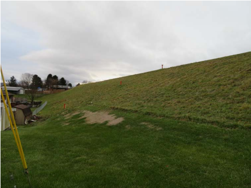
Photo 7: Downstream embankment slope, looking southwest.
