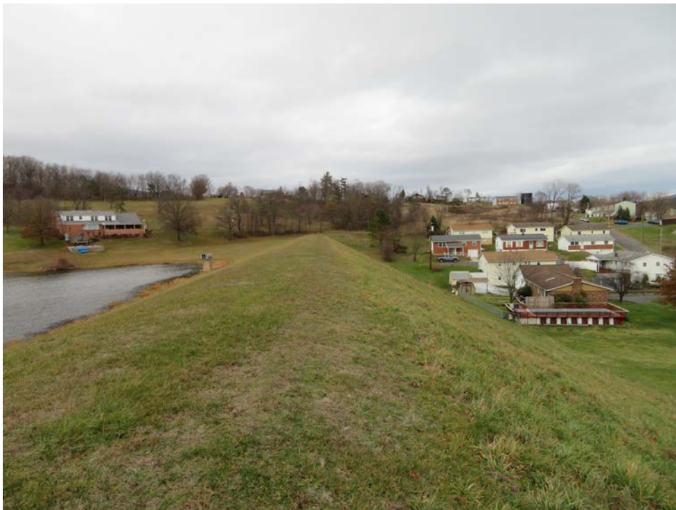
Photo 3: Crest of the dam, looking northeast.
