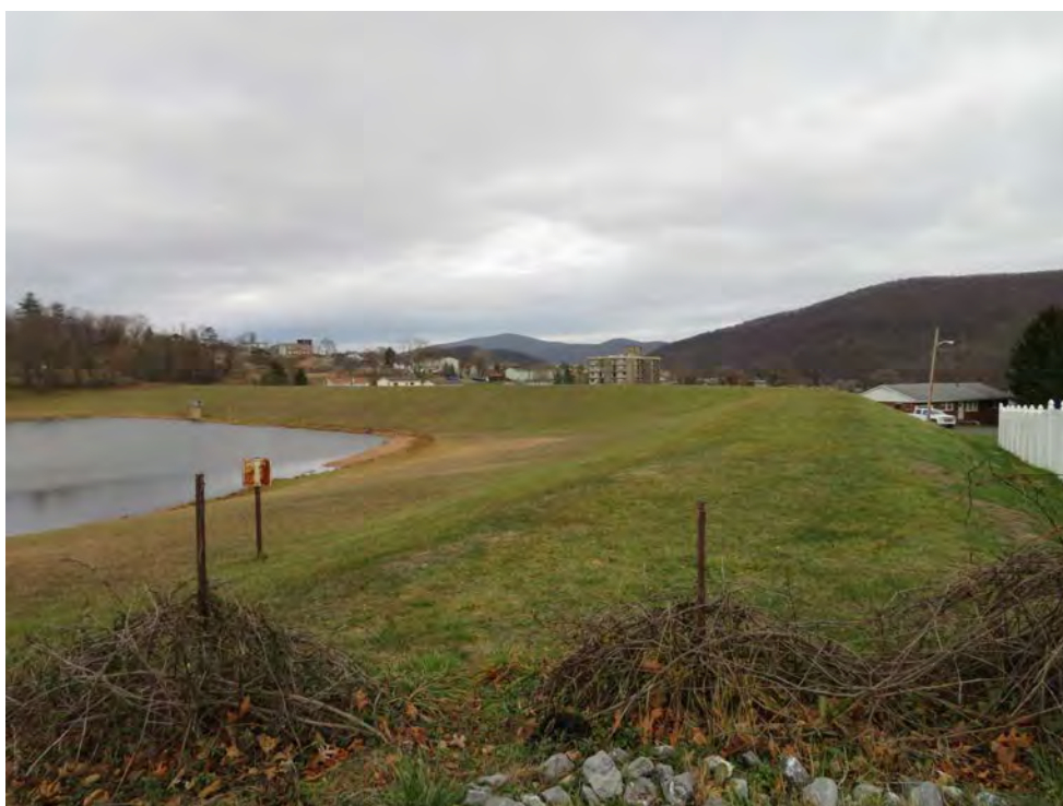
Photo 5: Overview of dam, looking northeast.
