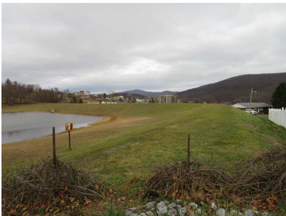
Photo 5: Overview of dam, looking northeast.
