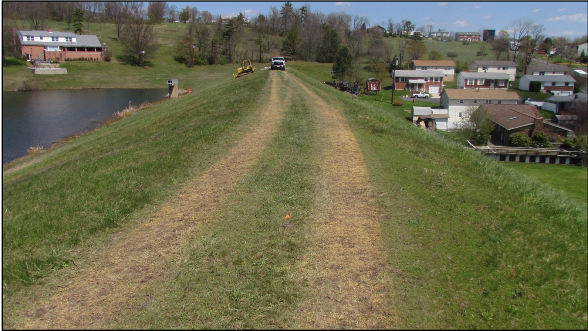
Looking northeast across New Creek Site 1 embankment
