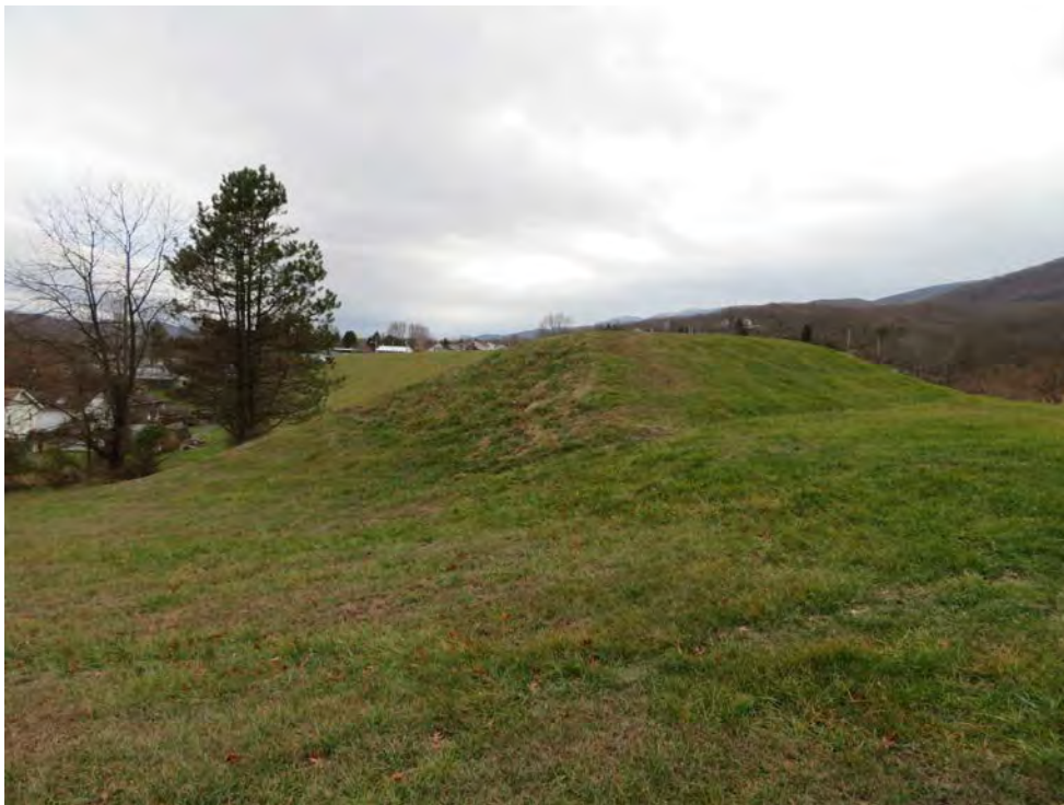
Photo 4: Northeast end of the dam, looking southwest.
