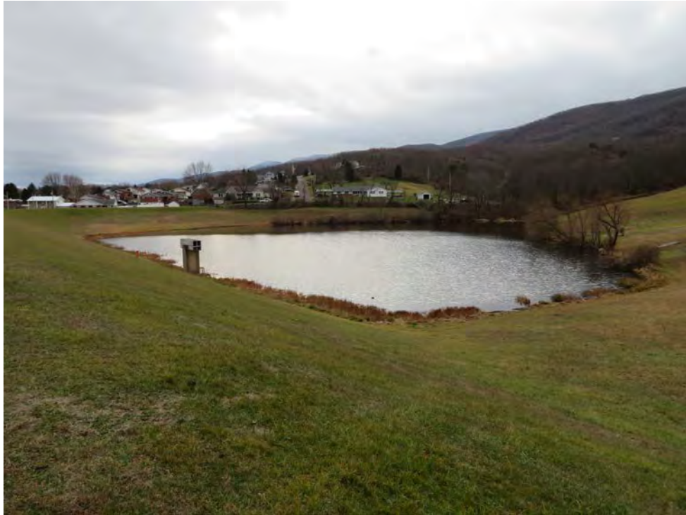
Photo 2: Reservoir, looking southwest.
