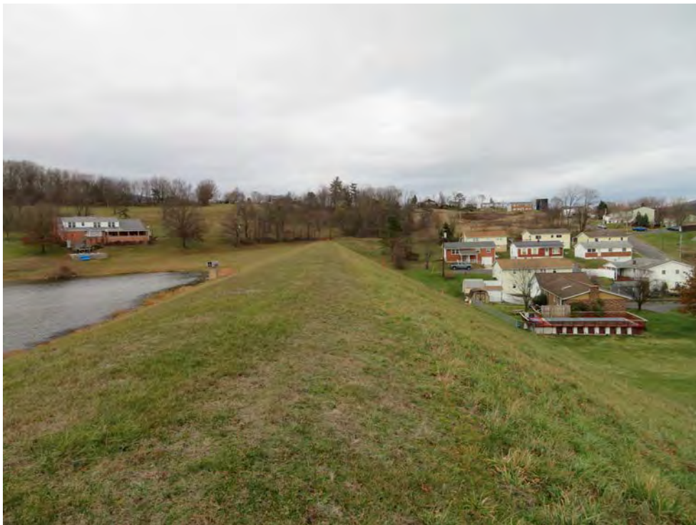
Photo 3: Crest of the dam, looking northeast.
