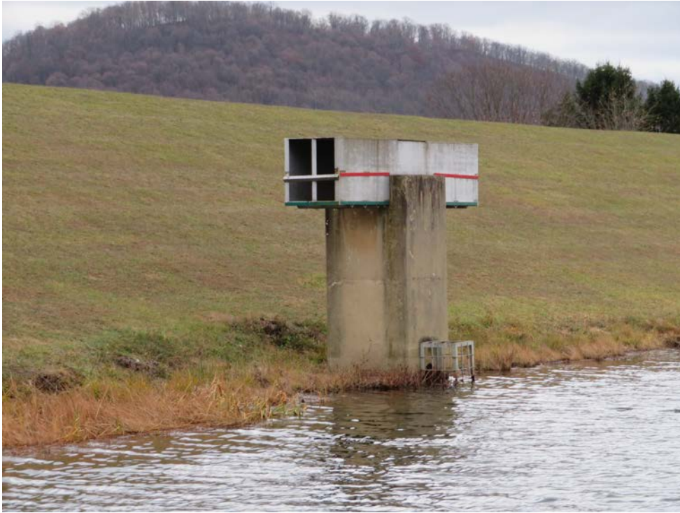
Photo 6: Principal spillway riser structure, looking south.
