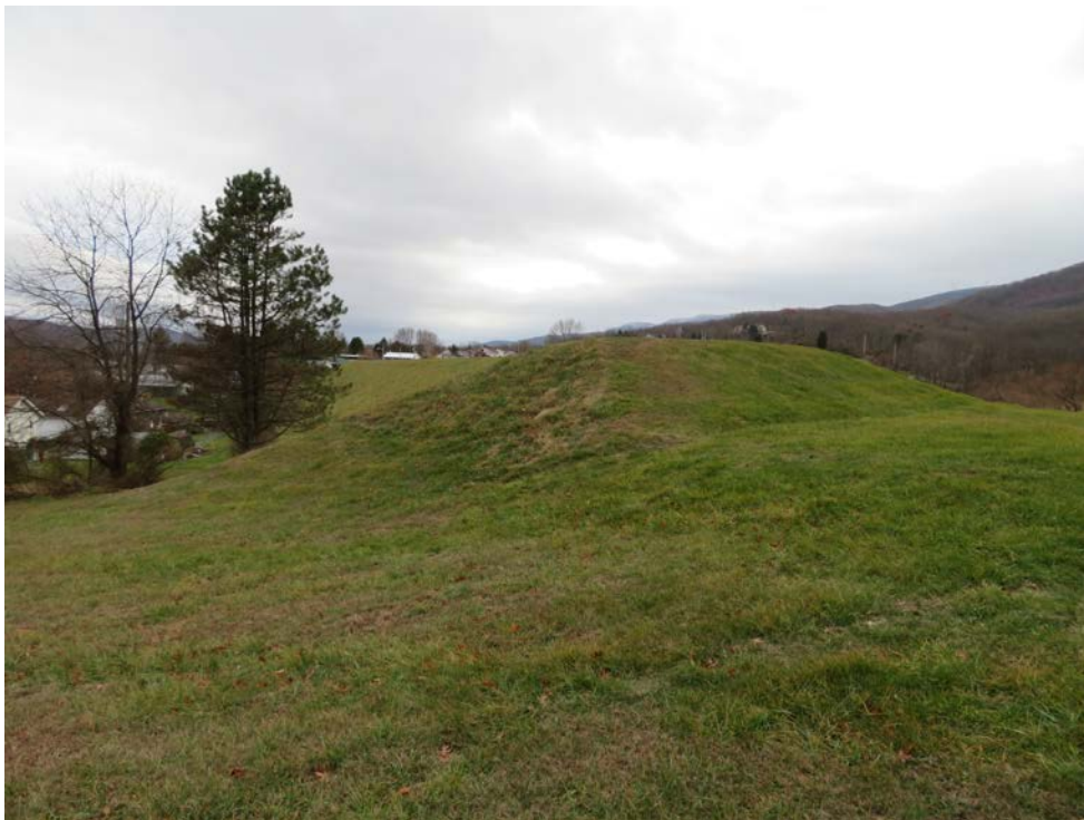
Photo 4: Northeast end of the dam, looking southwest.
