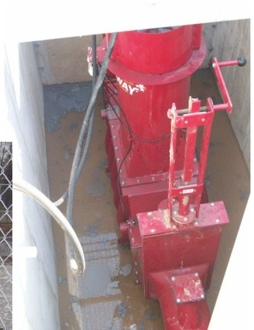
Piston transfer Pump
