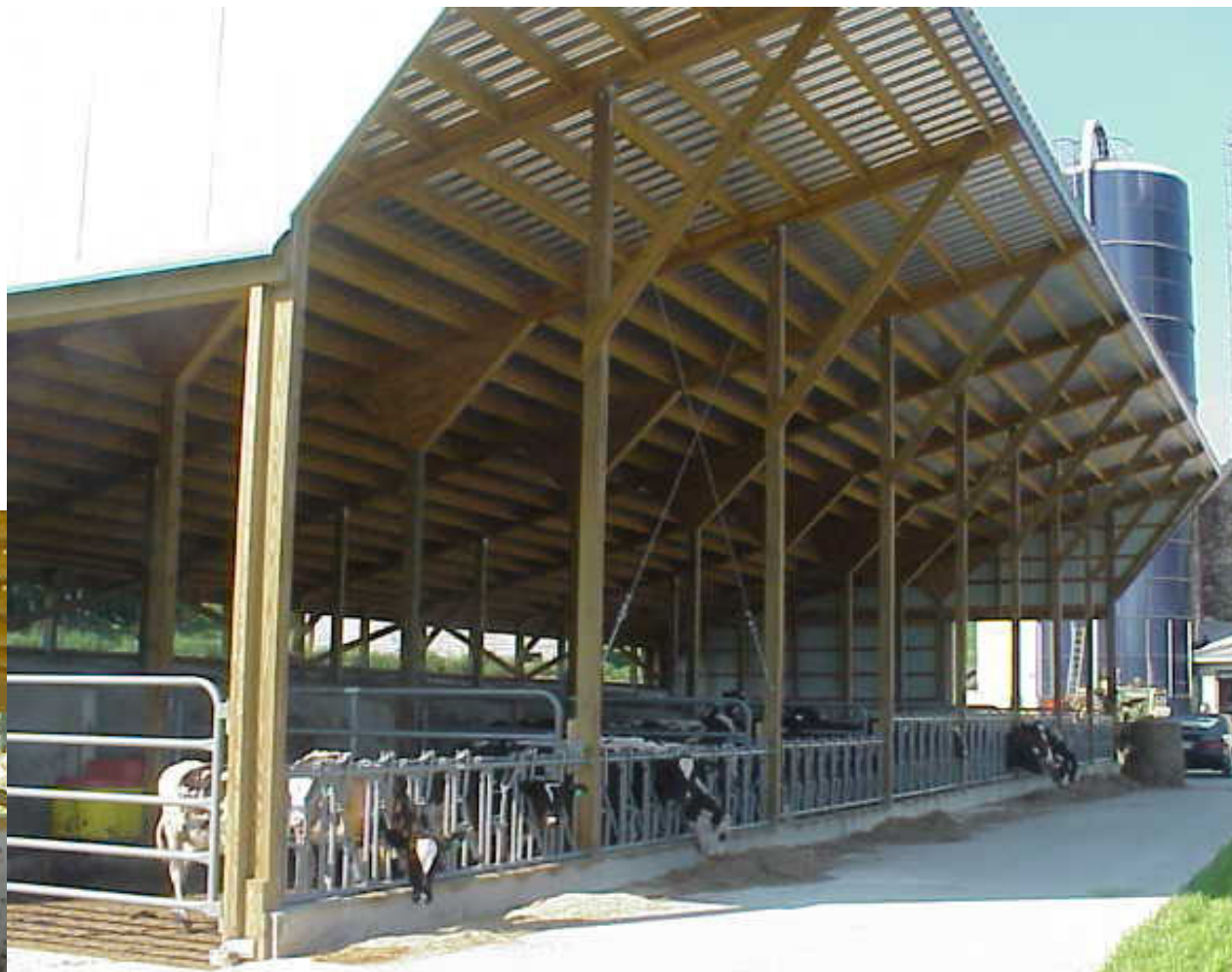
Virginia style, mono-slope roofed heifer facility with slatted floor above concrete storage tank
