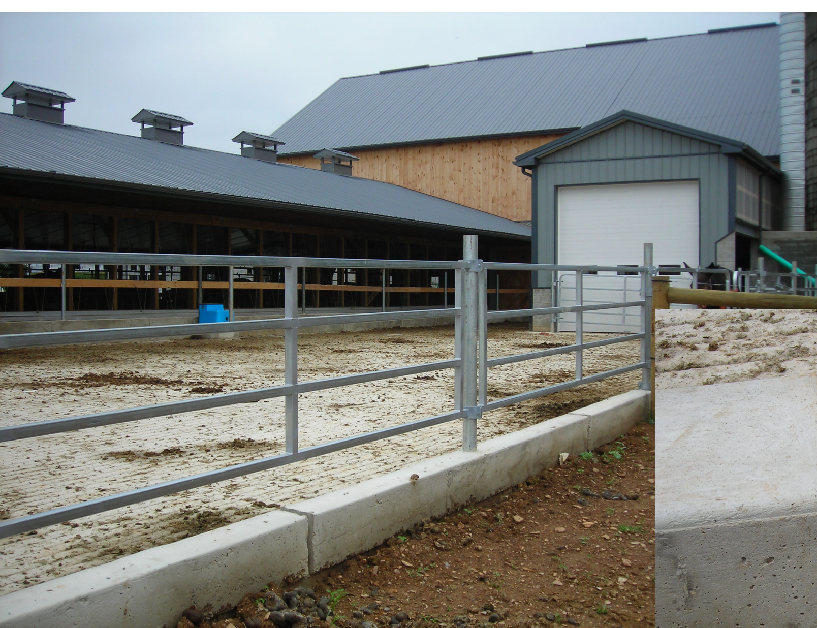
Barnyard paving and runoff collection with a perforated curb
