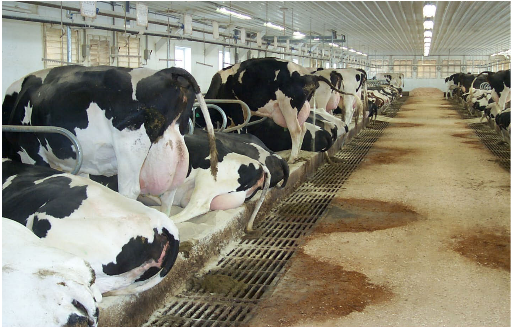
Tie stall barn with extra large gutters used to hold sand laden manure for several days and then cleaned out with chain and flight system
