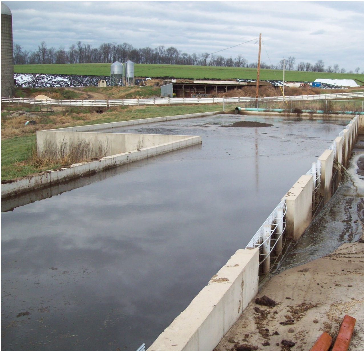
Long term settling basin using weeping walls to dewater solids on a flush alley dairy
