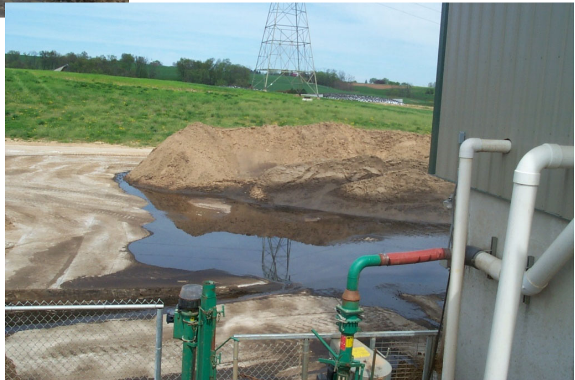
Processing area for gravity separated sand from an alley flush systems
