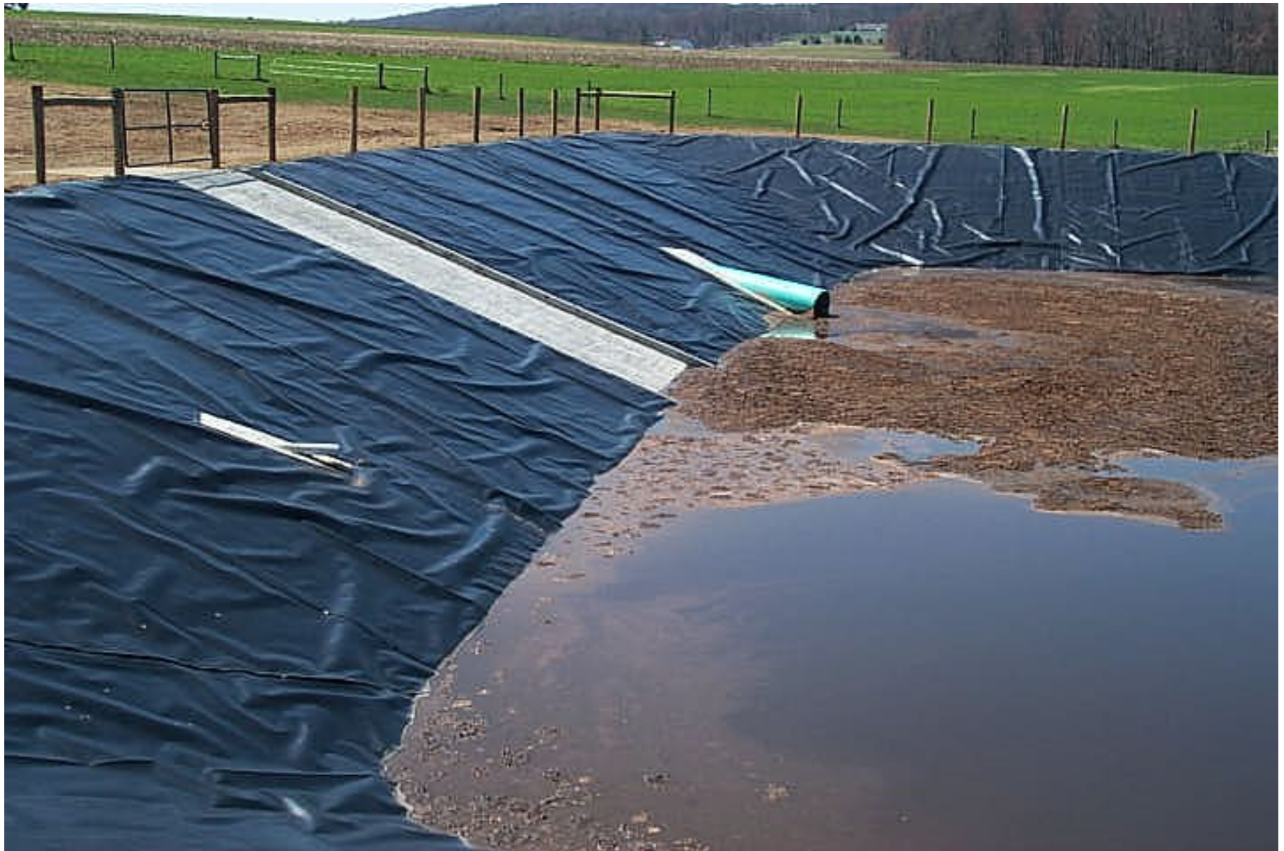
HDPE lined earthen storage with access ramp and gravity fill pipe for manure and leachate
