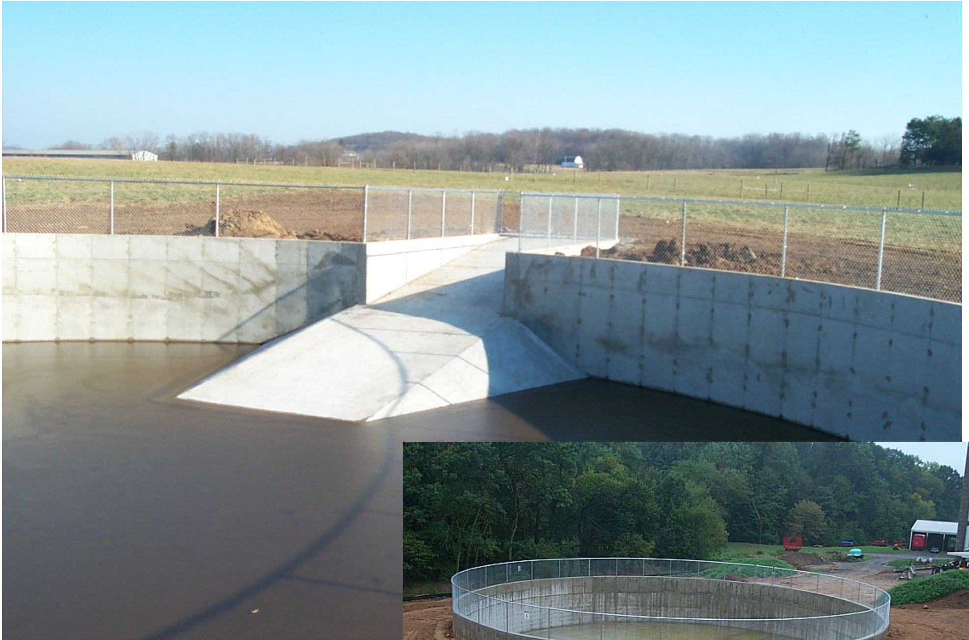
Concrete tank with Ramp
