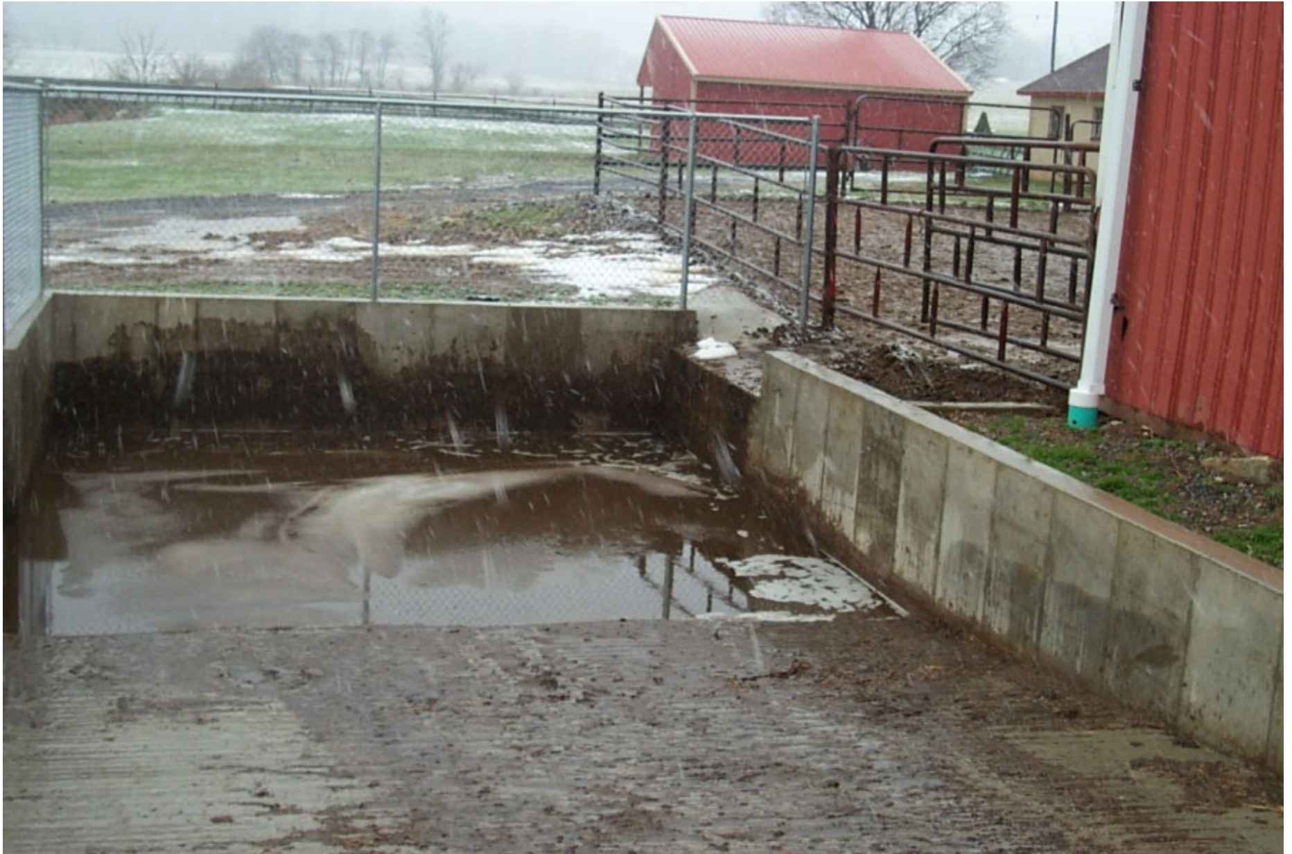
Settling basin off concrete barnyard
