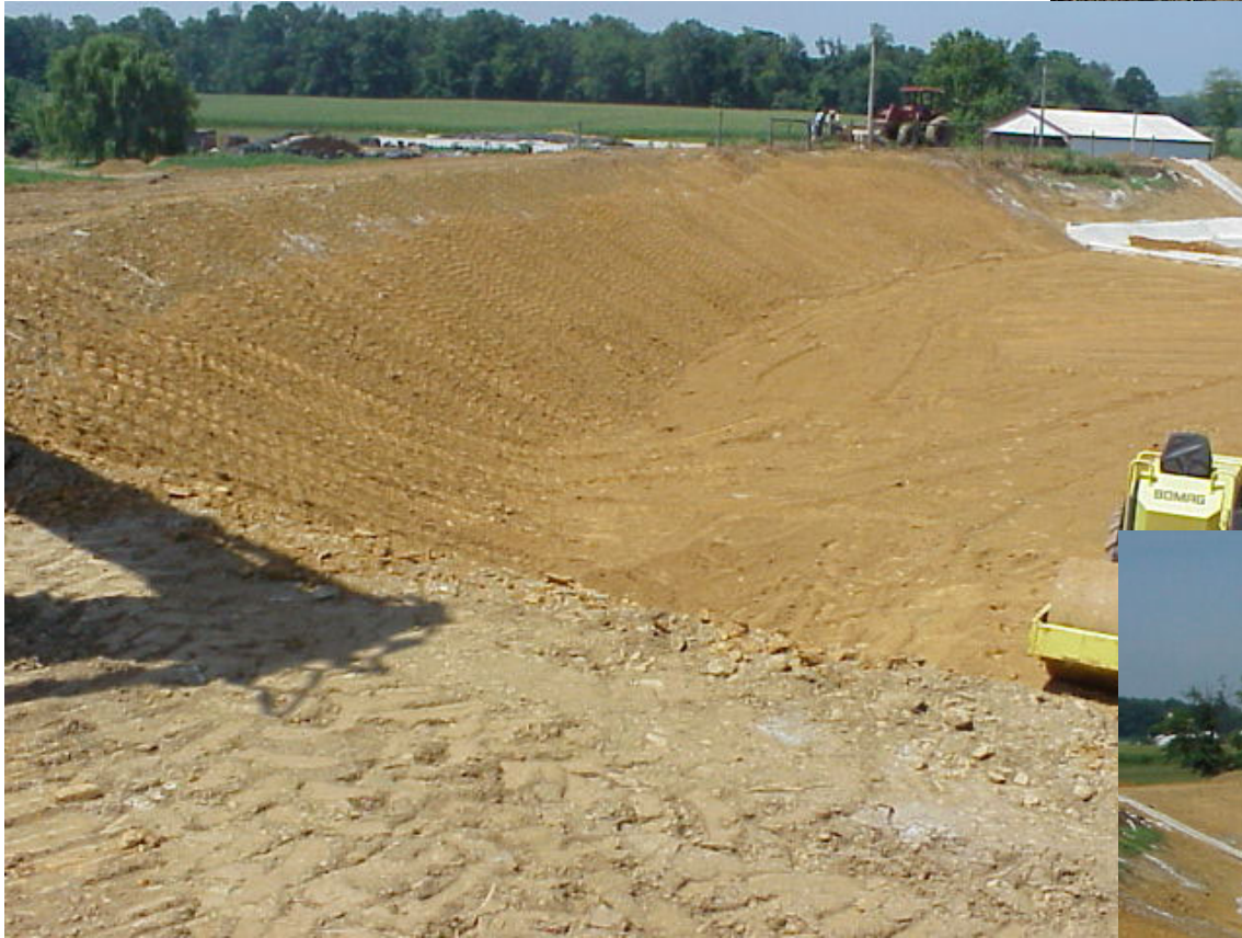
Relining existing earthen storage with bentonite and concrete
