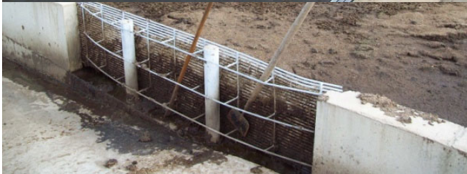
Long term settling basin using weeping walls to dewater solids on a flush alley dairy
