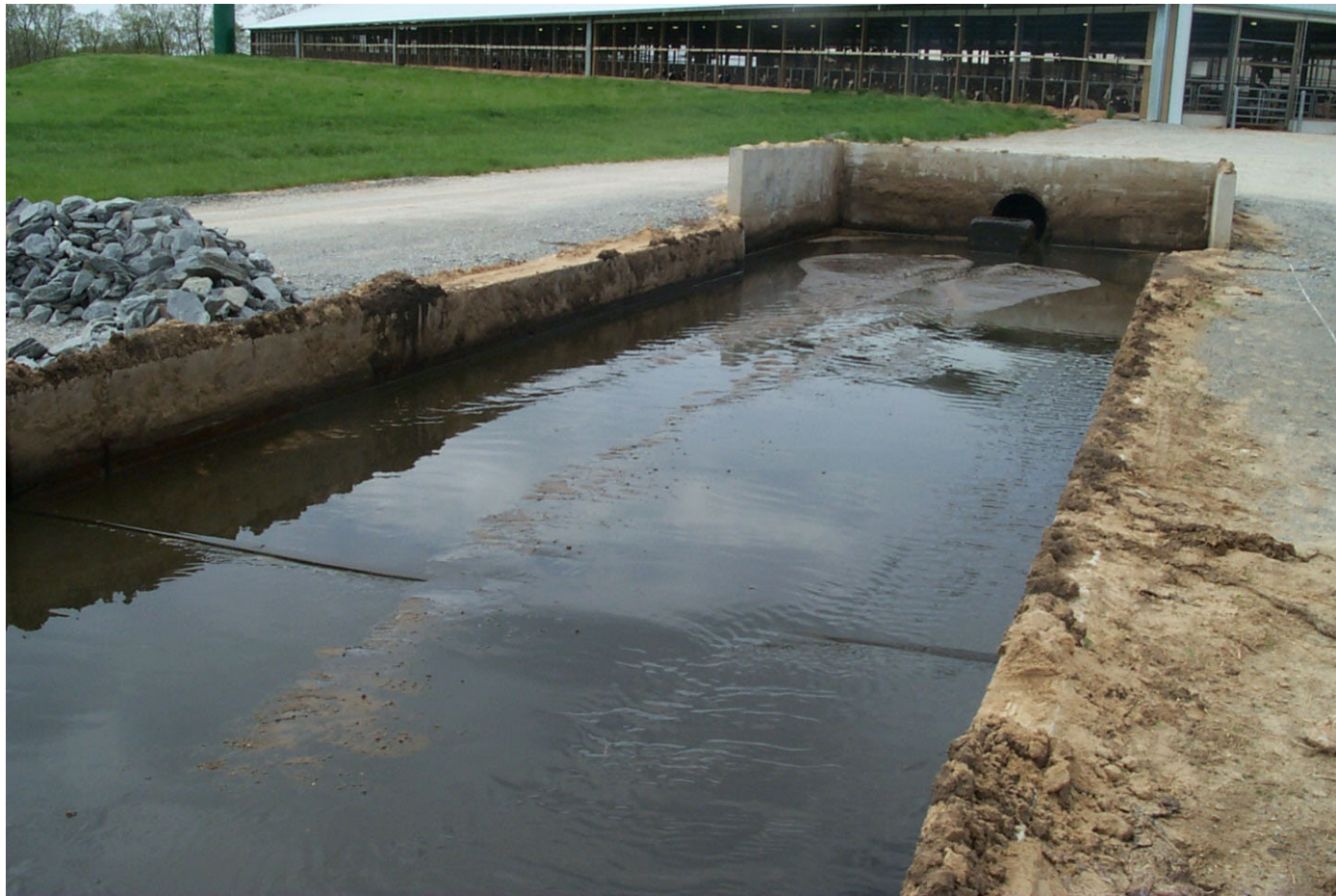
Sand Settling lane looking upstream during flush discharge
