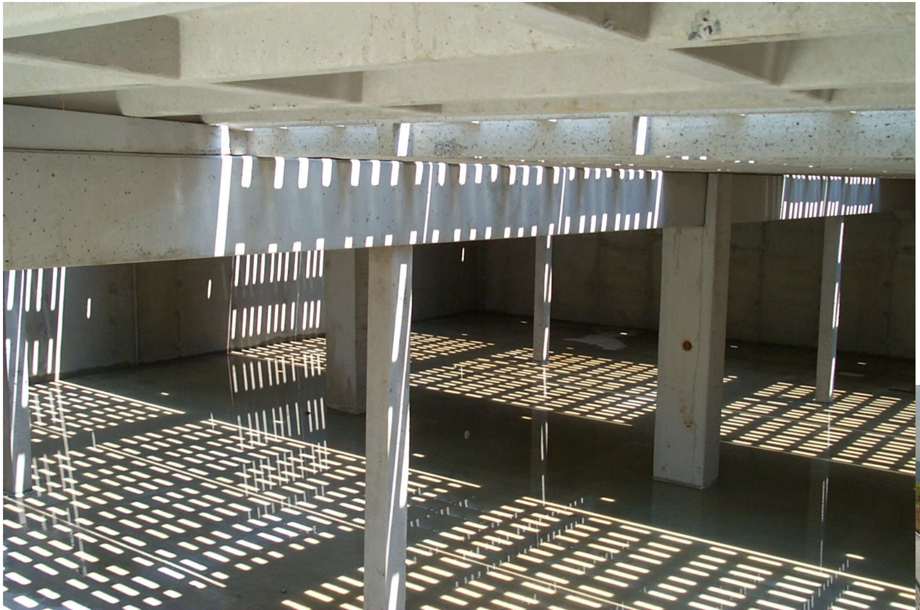
Interior view of slatted floor storage facility showing post and beam supports
