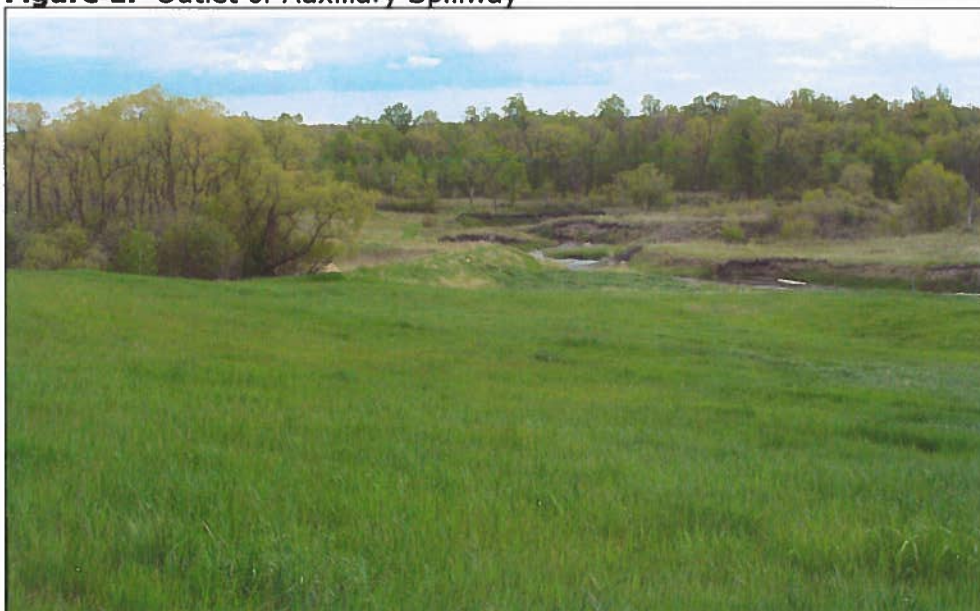
Figure 1. Outlet of Auxiliary Spillway
