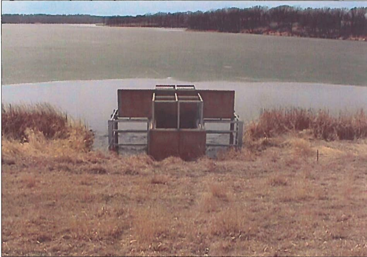
Figure 4. Principal Spillway - Renwick Dam
