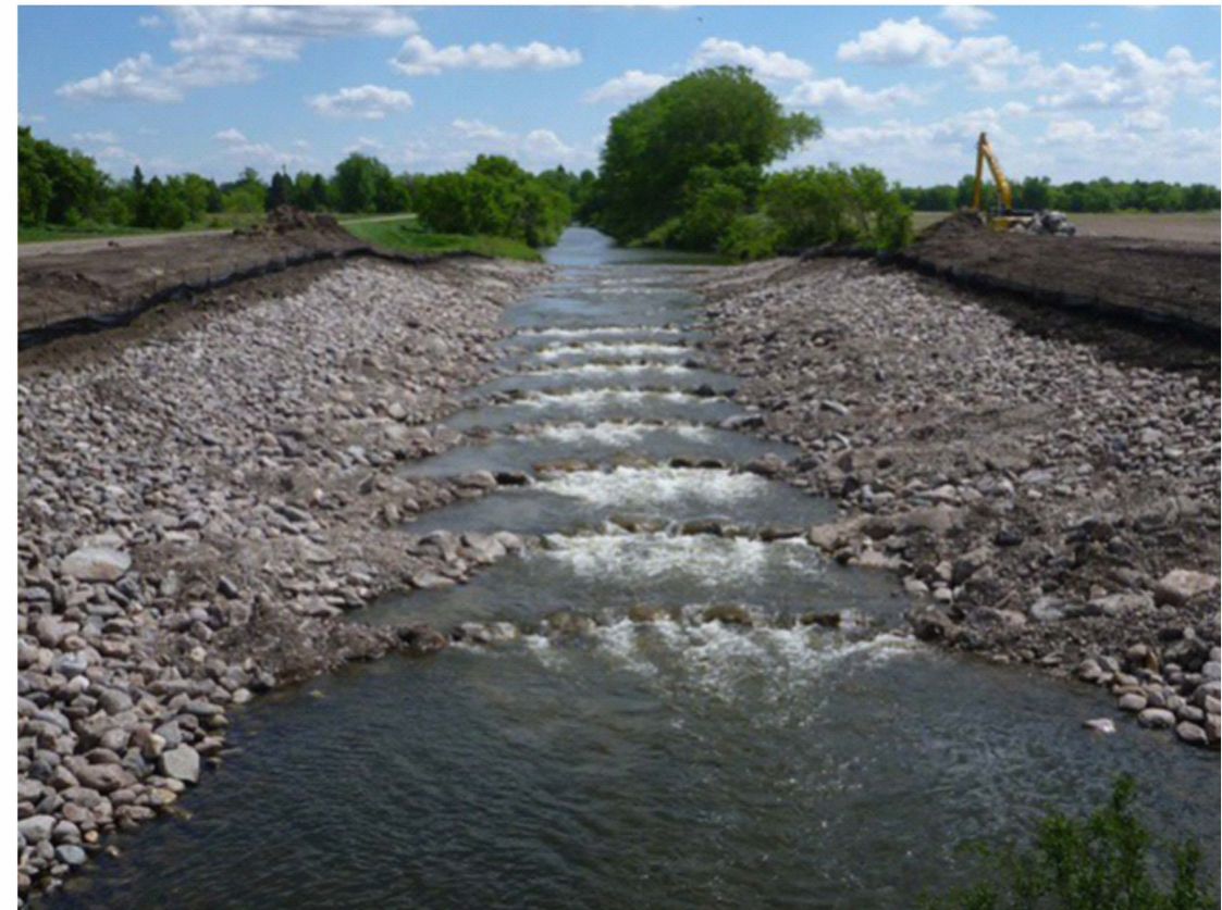
EXAMPLE STRUCTURE LOOKING UPSTREAM
