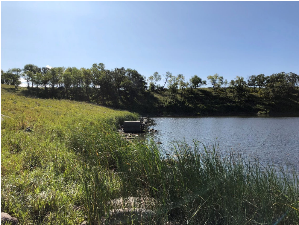
Photo 4 – upstream embankment looking SE
