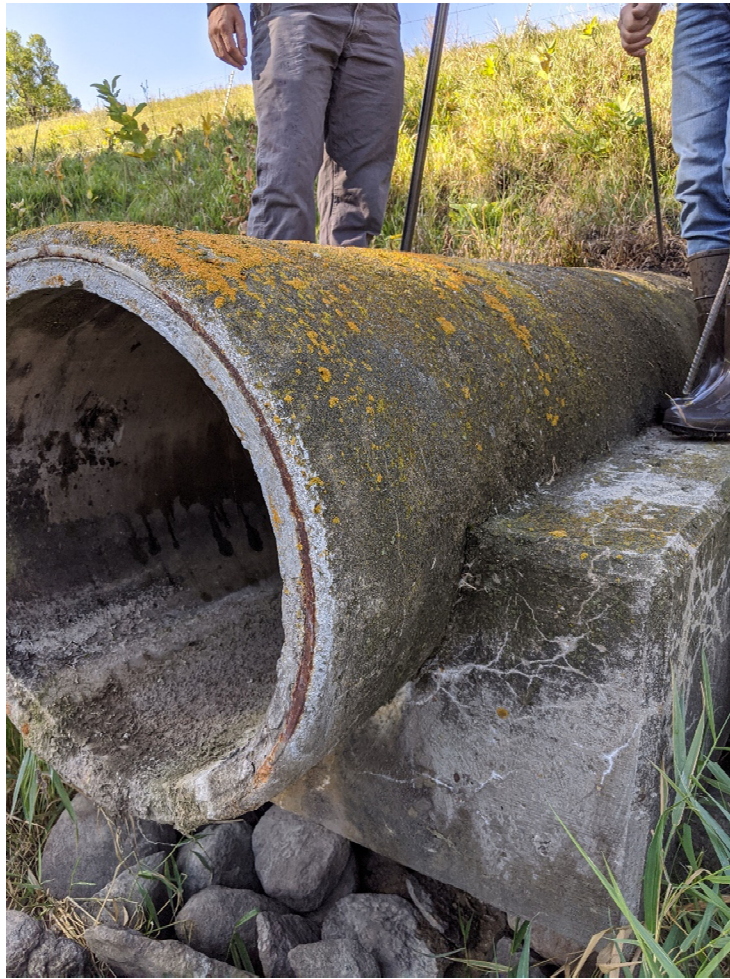
Photo 23 – principal spillway conduit outlet looking S
