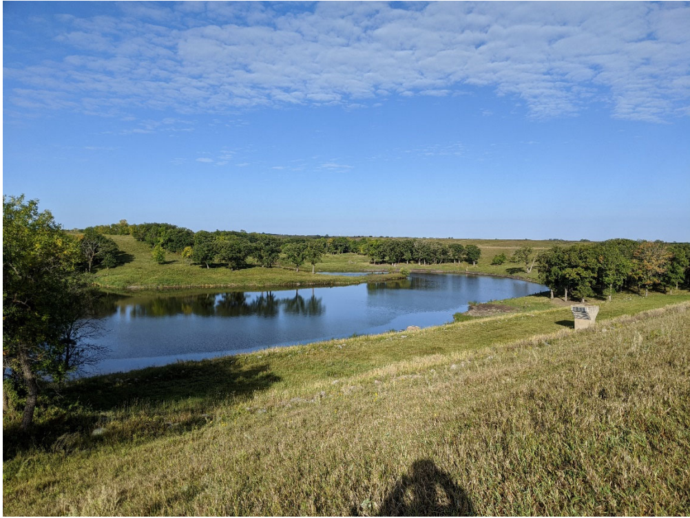
Photo 27 – reservoir looking NW
