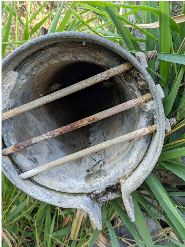
Photo 26 – foundation drain animal guard
