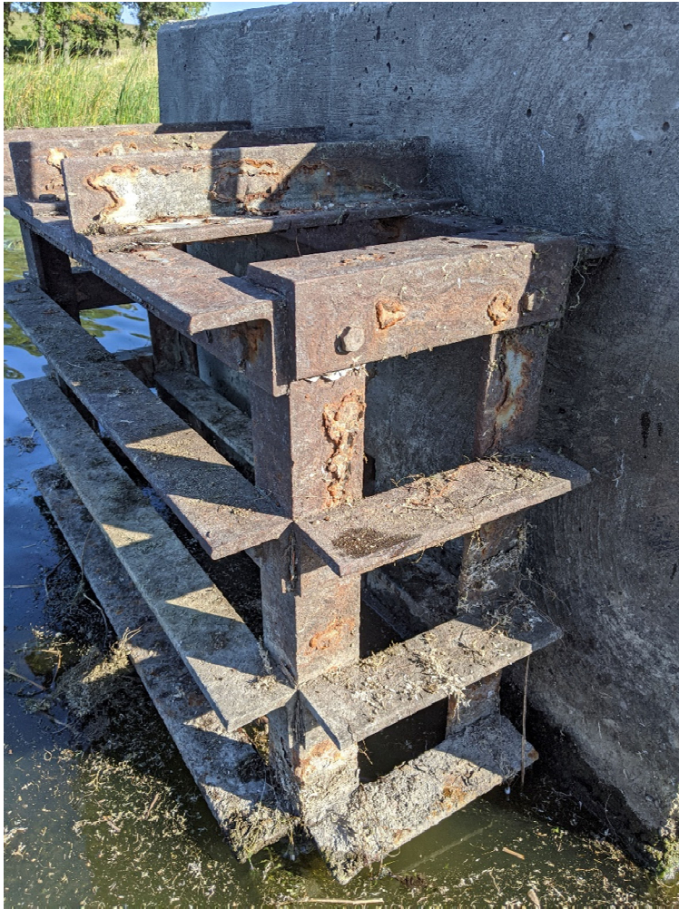
Photo 19 – low-stage riser trash rack
