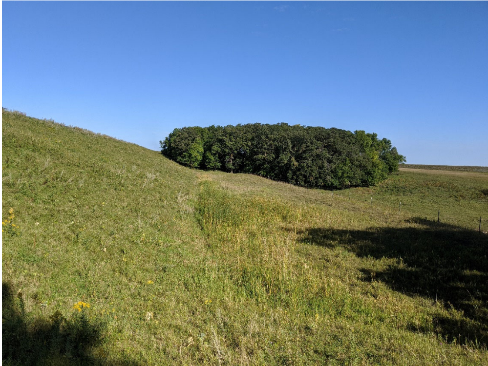
Photo 9 – downstream slope bench looking NW
