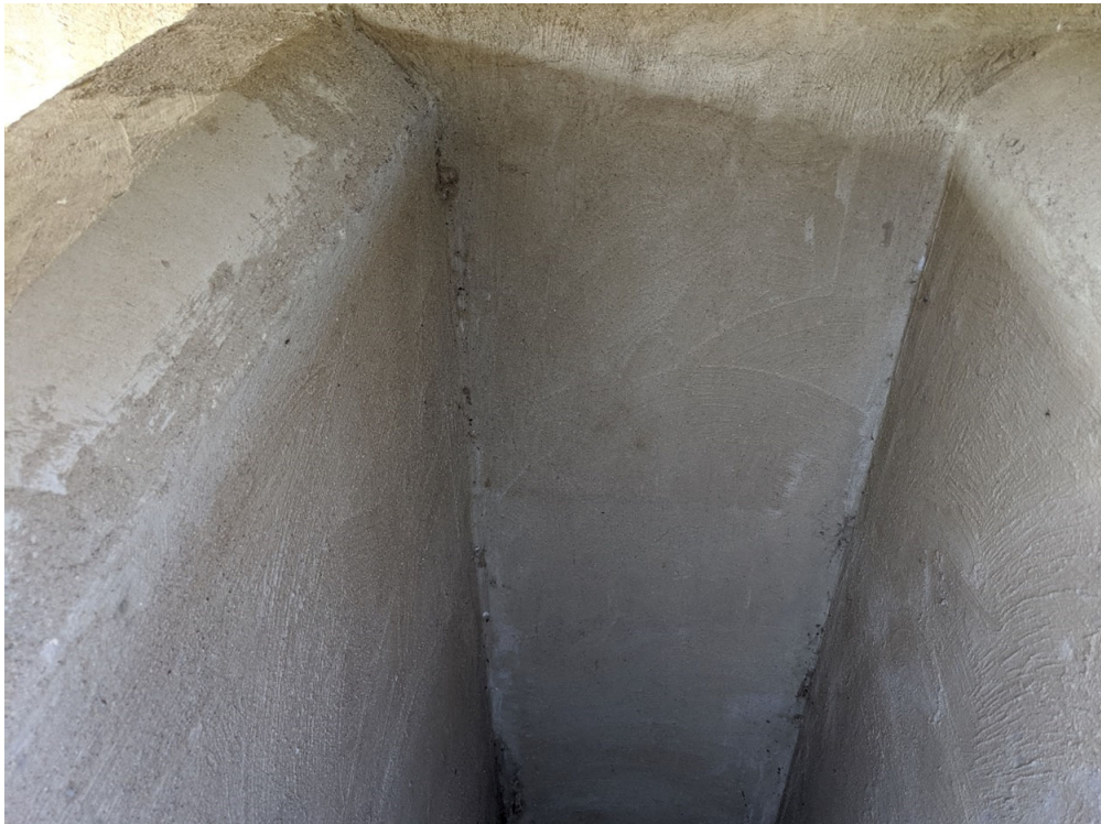
Photo 22 – crest of principal spillway tower looking NE
