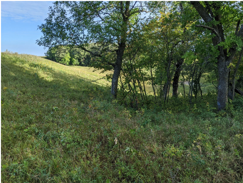
Photo 12 – tree encroachment on right downstream abutment looking N
