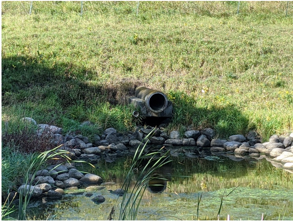
Photo 25 – principal spillway and foundation drain outlet looking W
