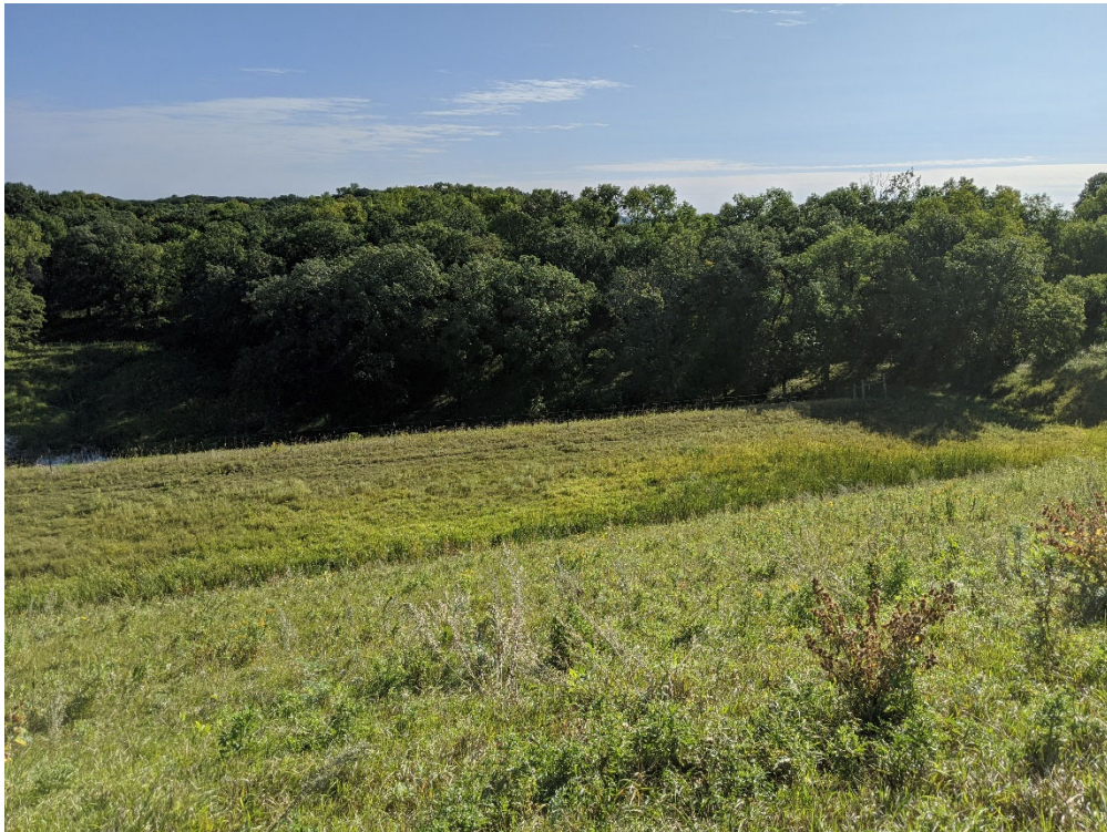
Photo 10 – weeds and cattails on downstream bench looking E
