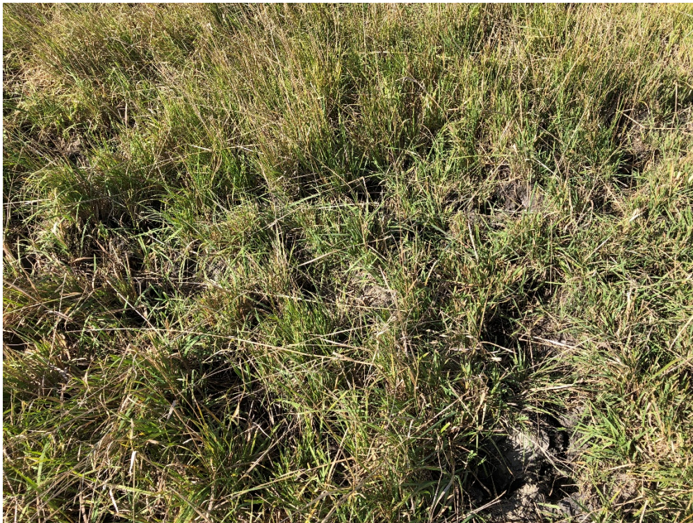
Photo 16 – rutting in auxiliary spillway
