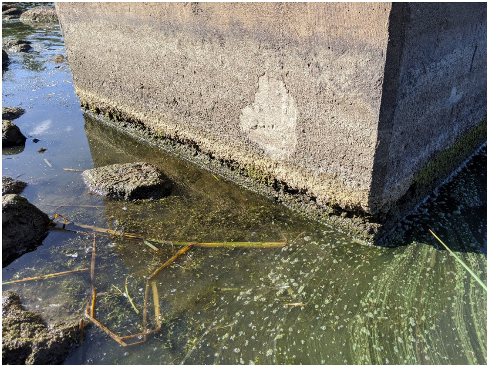
Photo 20 – exterior of low-stage riser looking S
