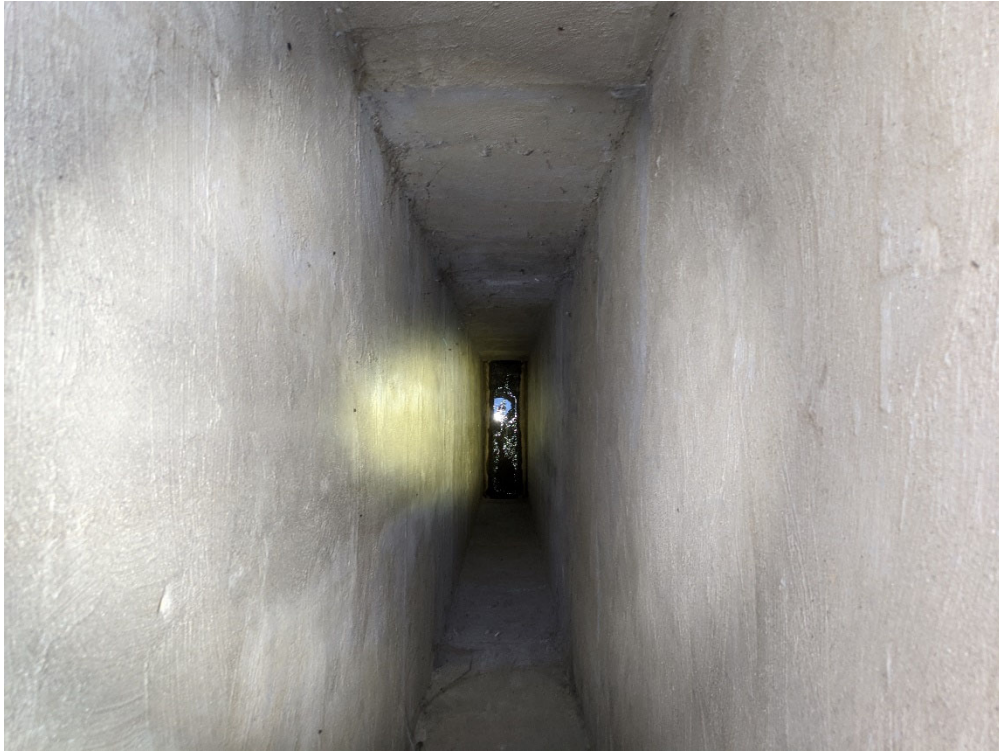
Photo 3 – principal riser tower
