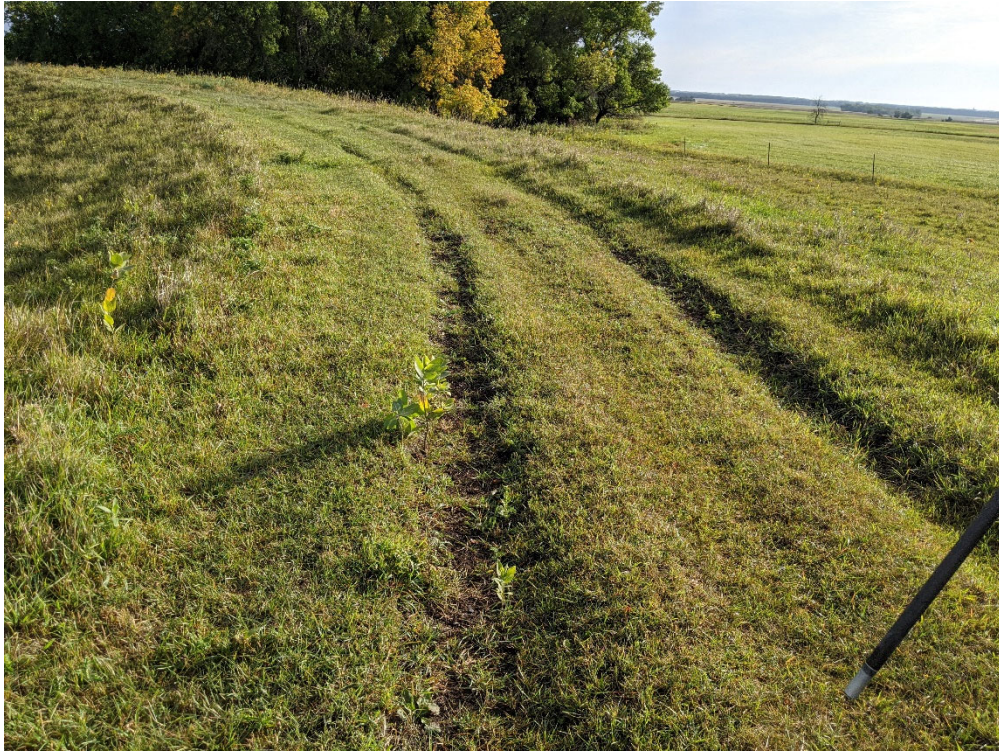
Photo 7 – rutting on the crest looking NE
