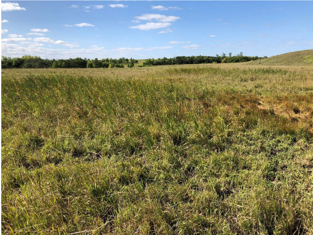
Photo 17 – distinct vegetation change in auxiliary spillway looking SE
