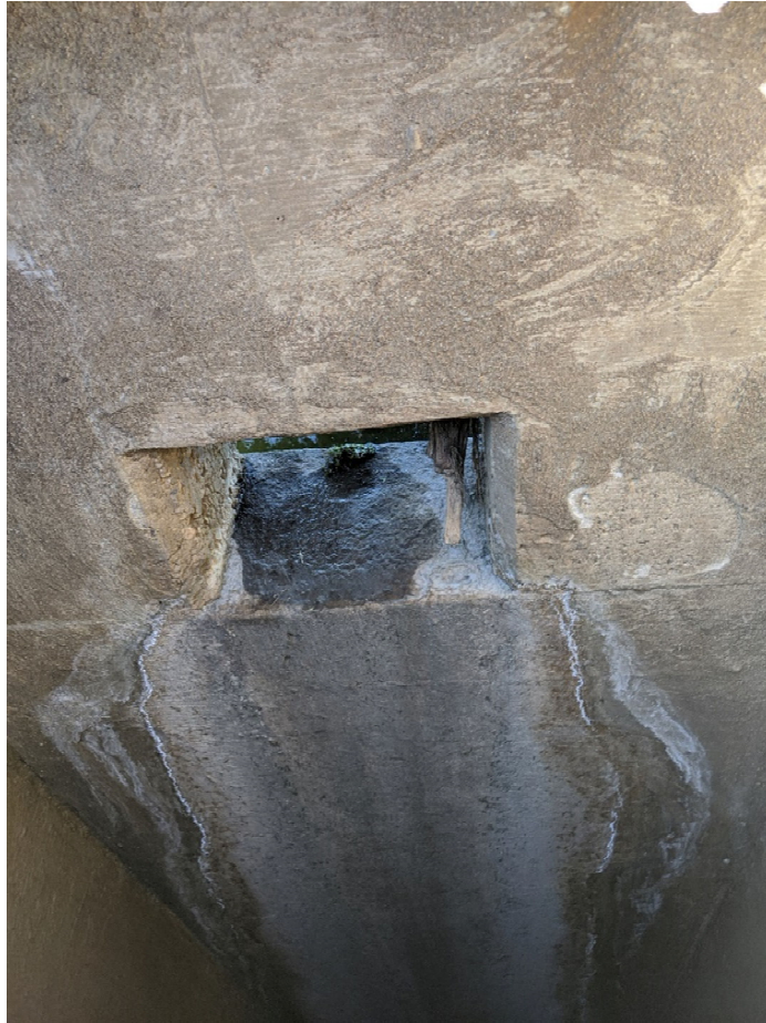
Photo 1 – low-stage riser orifice
