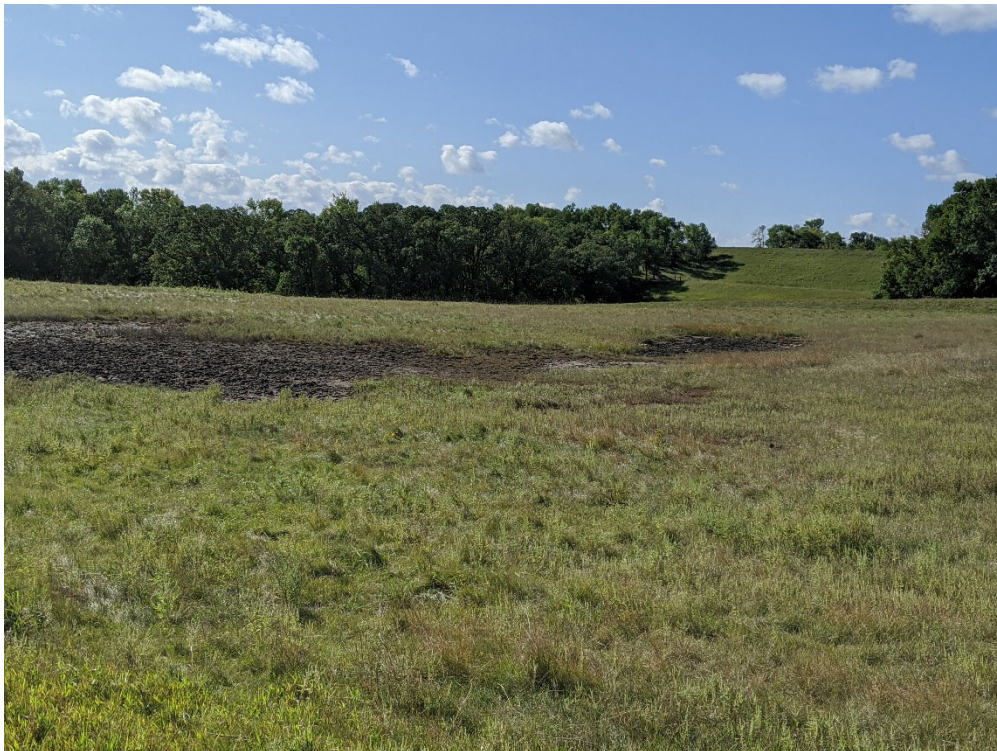
Photo 18 – unvegetated portion of auxiliary spillway looking NE
