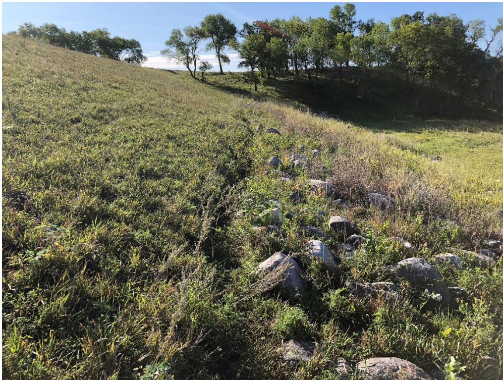
Photo 6 – animal trail along riprap looking SE
