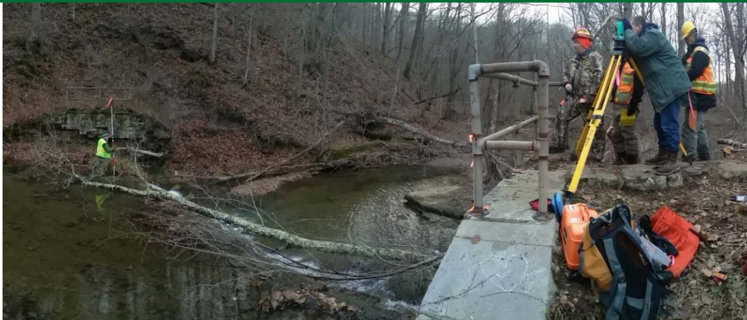
Surveying for stream restoration to improve fish passage and sediment transport
