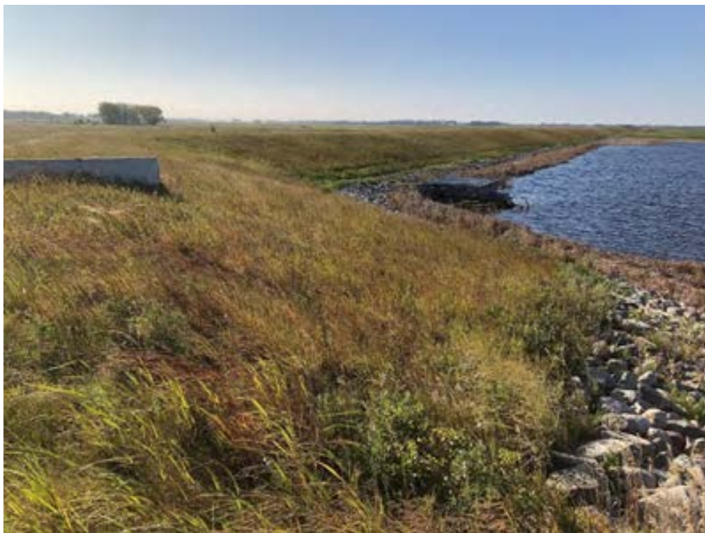
Photo 19 Principle spillway inlet structure; concrete barrier on top of dam to discourage vehicle activity
