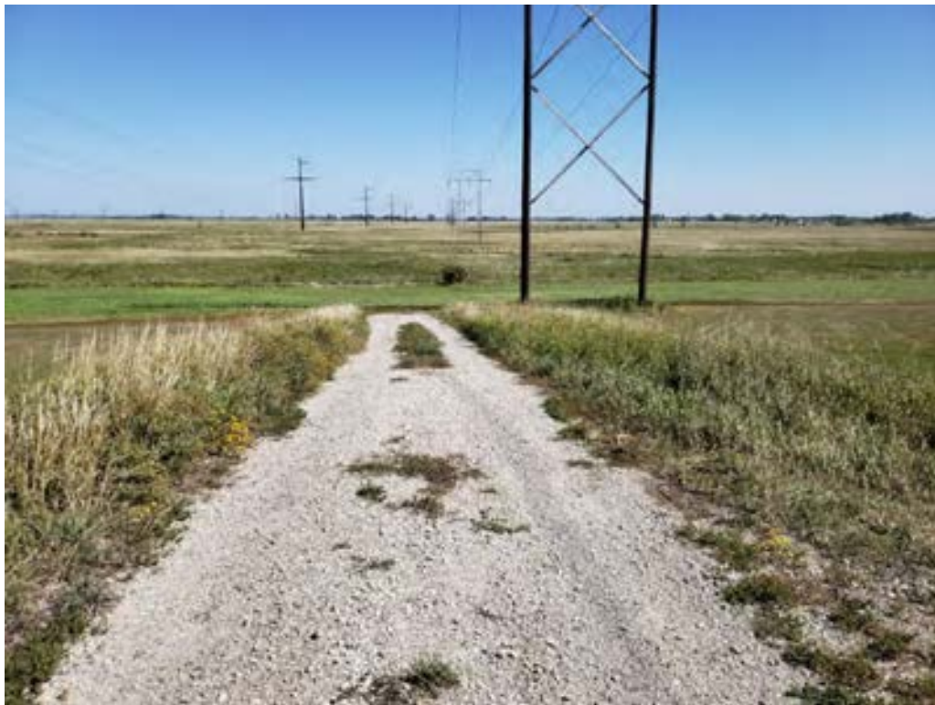
Photo 37 Access road across embankment for powerline causeway
