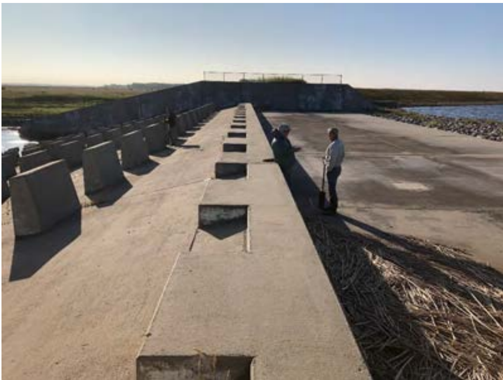
Photo 2 Auxiliary spillway inlet crest
