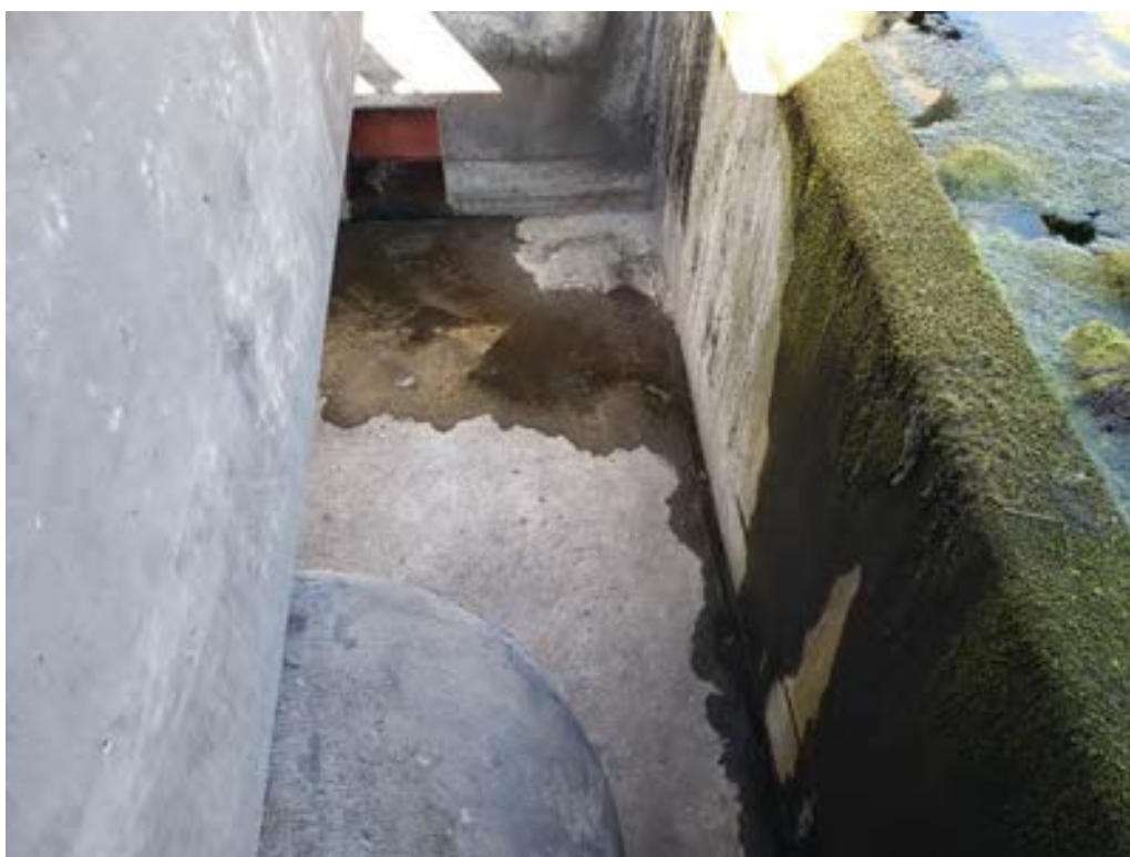
Photo 20 Principle spillway inlet: weir invert and low level drawdown gate
