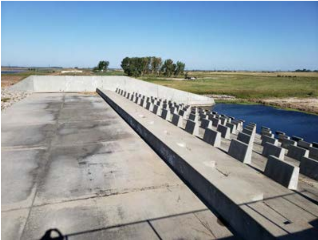
Photo 1 Auxiliary spillway weir crest and baffled chute
