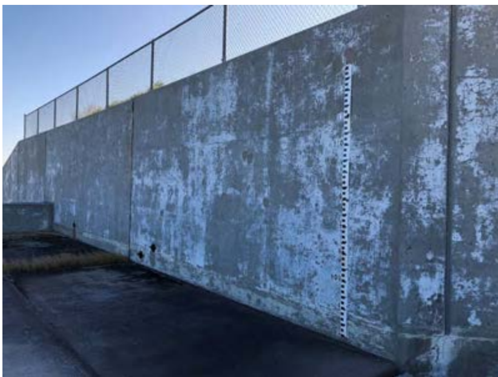
Photo 10 Staff gauge on right wall of AS; board members noted gauge is difficult to read from opposite side during high water events
