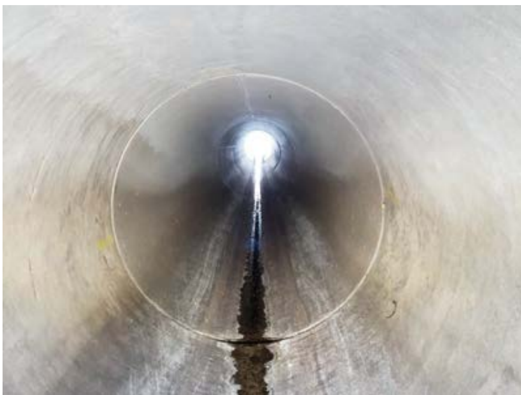
Photo 26 Looking down the principle spillway conduit
