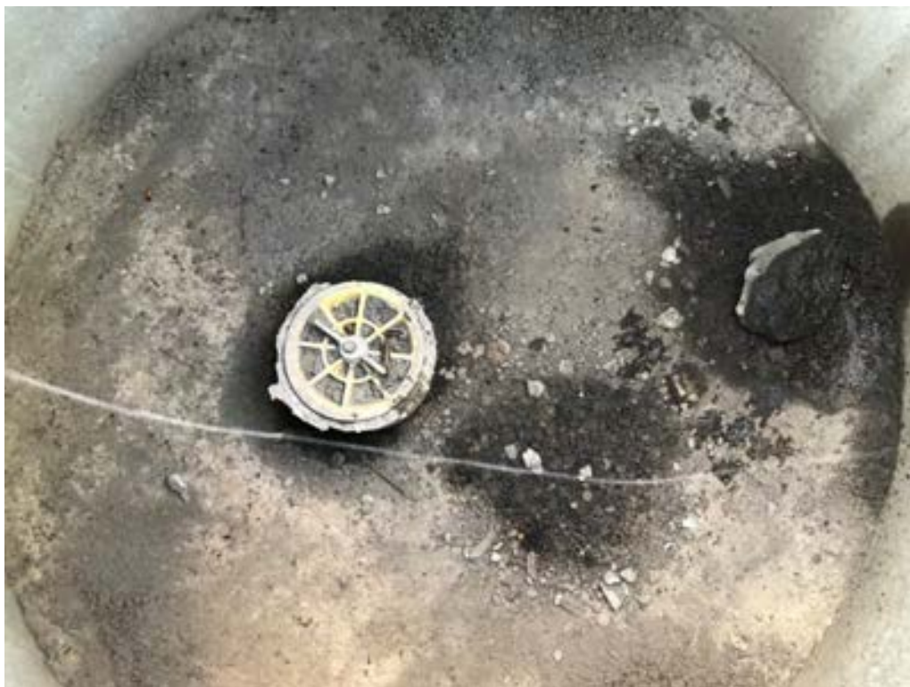
Photo 13 Inside of drain access manhole (typical)
