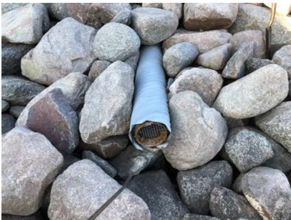
Photo 18 Auxiliary spillway foundation drain outlet (either side)
