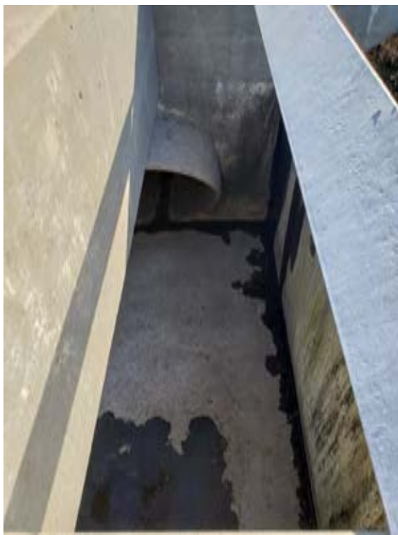
Photo 21 Principle spillway inlet: entrance to conduit
