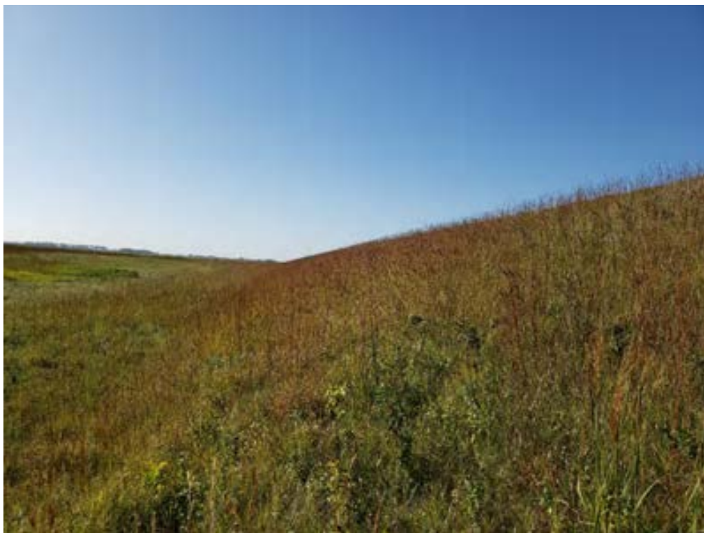
Photo 27 Downstream face of North/South right embankment
