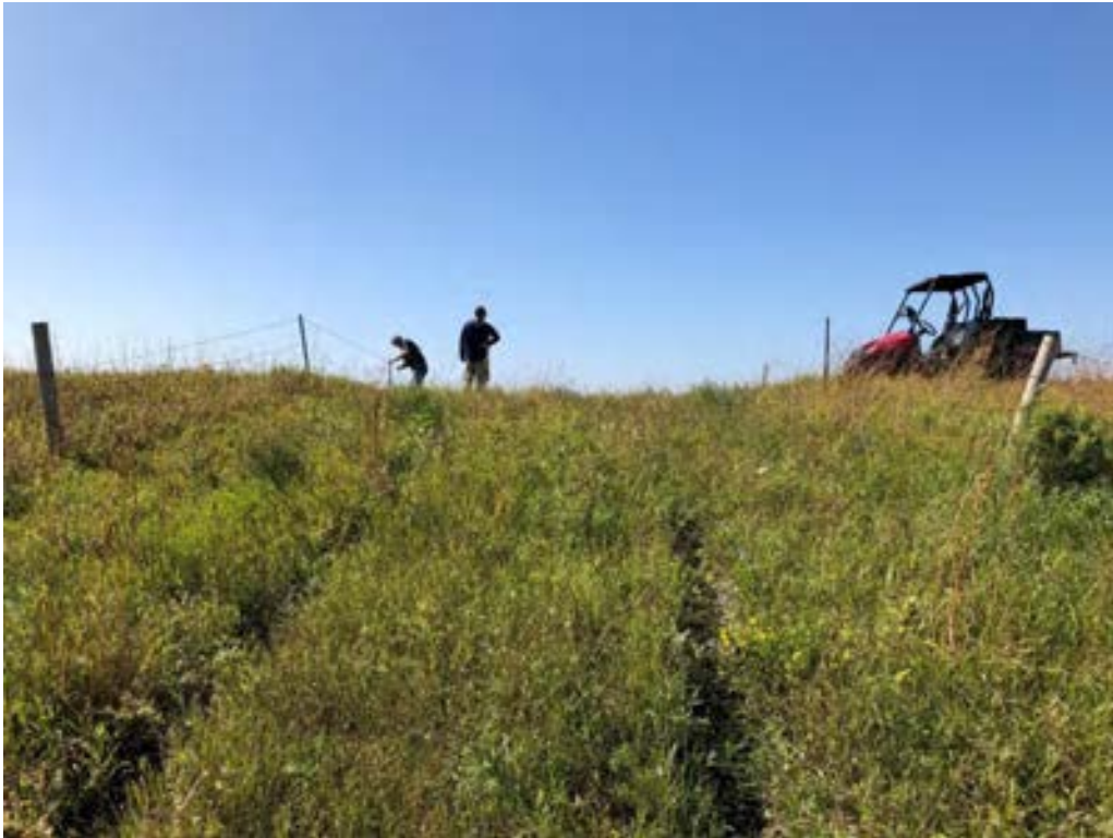
Photo 39 Tracks and rutting on downstream face of embankment; fencing across embankment for cattle access
