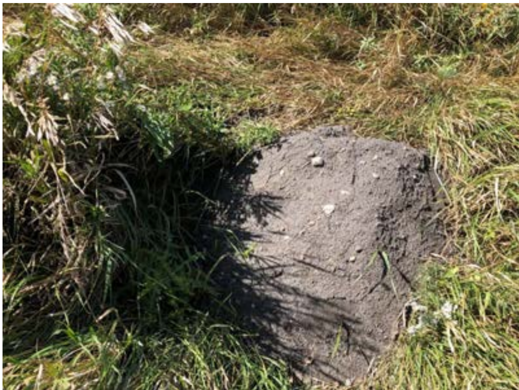
Photo 42 Animal burrow on crest of dam
