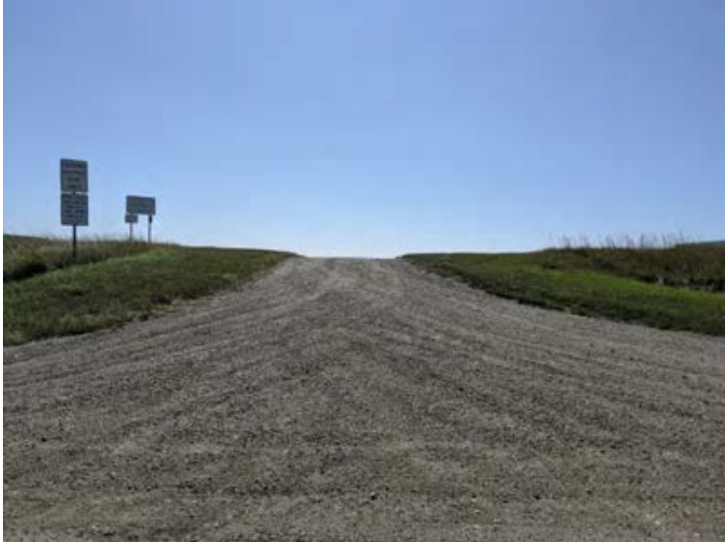
Photo 41 Graveled vehicle access across embankment of dam
