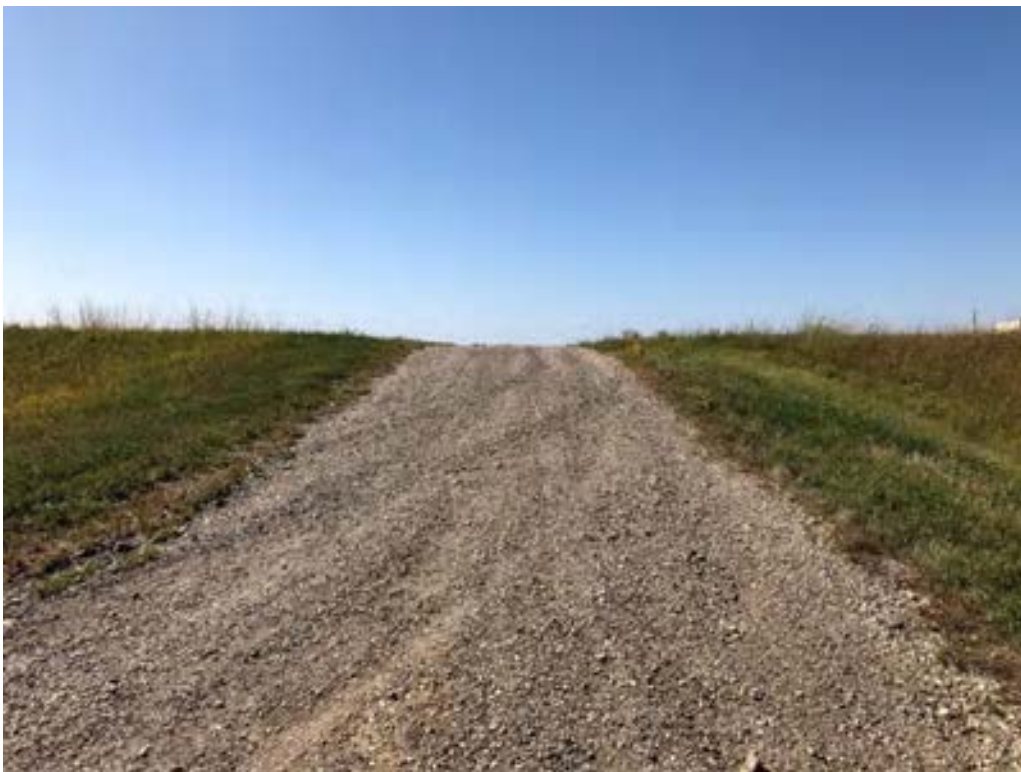
Photo 40 Graveled access across embankment of dam
