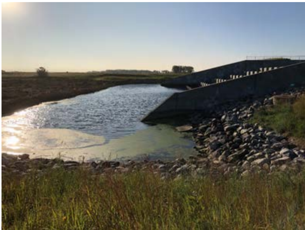
Photo 11 Auxiliary spillway stilling basin; bottom of spillway and drain access manhole submerged
