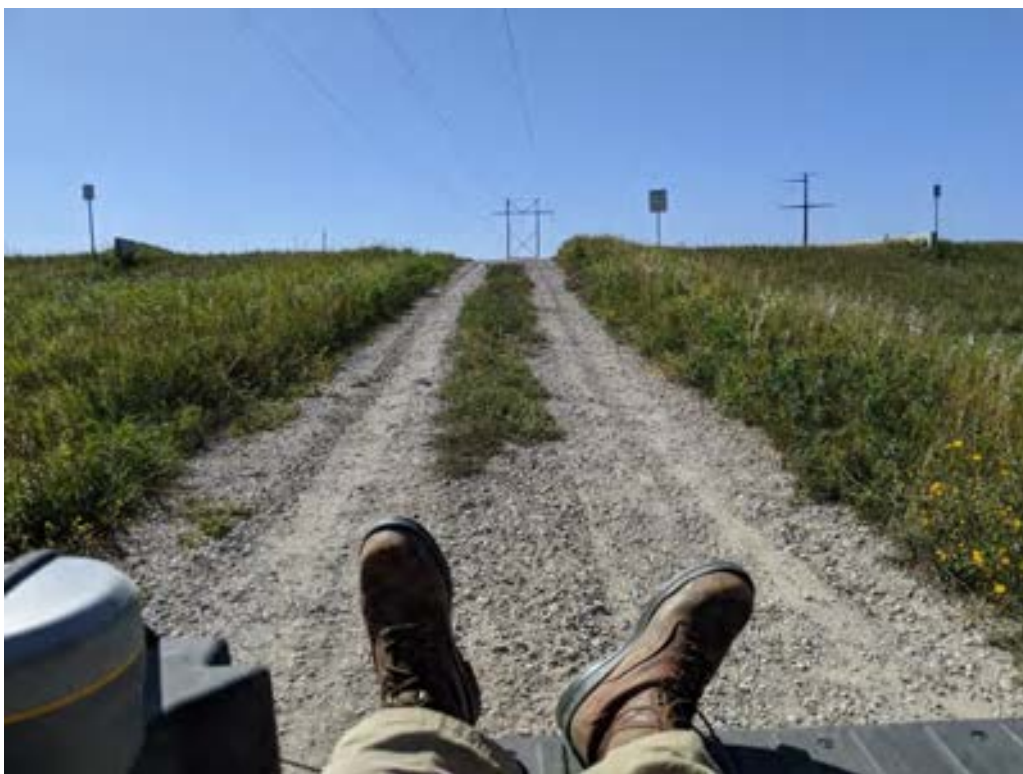
Photo 38 Graveled vehicle access across embankment of dam
