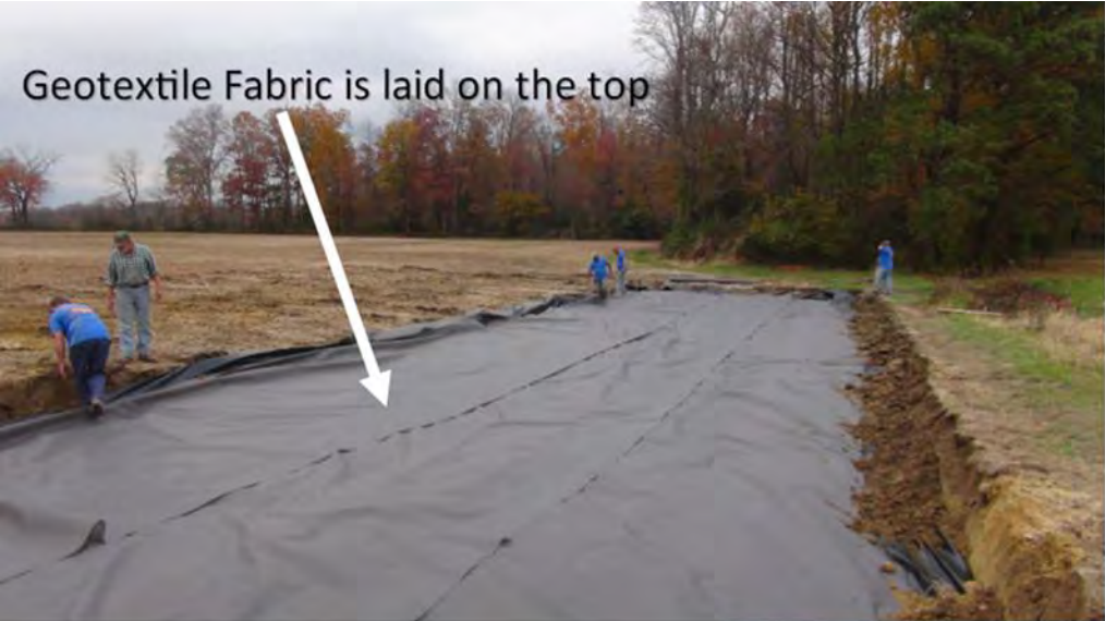
Trench is backfilled to surface elevation on the edge with slight crown in center
