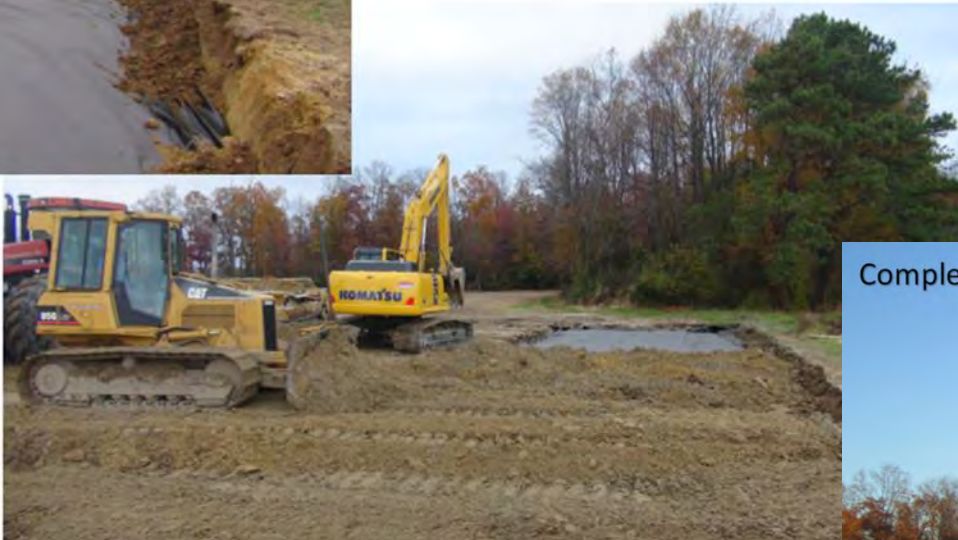
Trench is backfilled to surface elevation on the edge with slight crown in center
