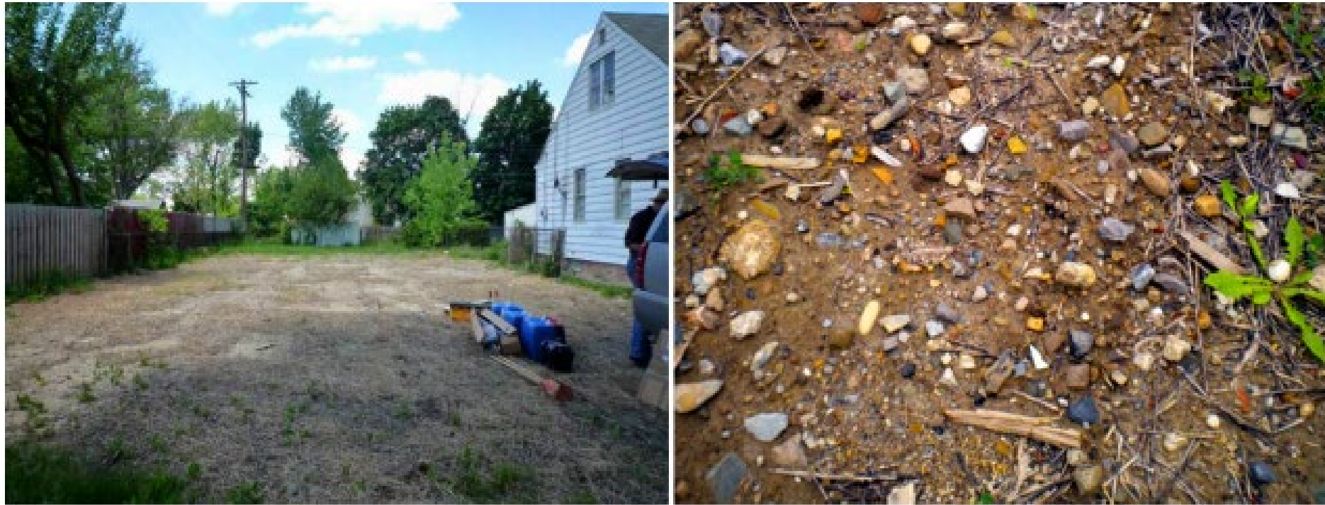
Figure 5. The case study location. Left photo shows the site post-demolition. Photo on the right shows an example of construction debris left after demolition.
