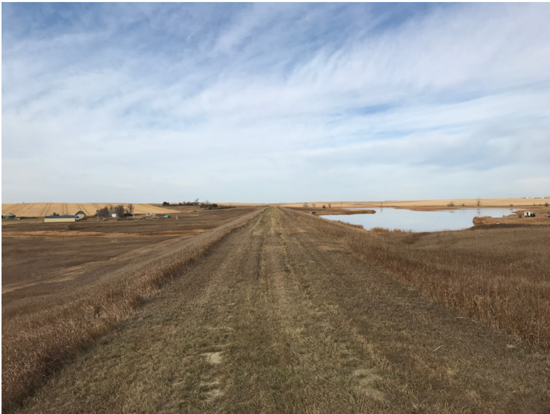
Photo #2 - View from Left Abutment looking along Dam Crest
