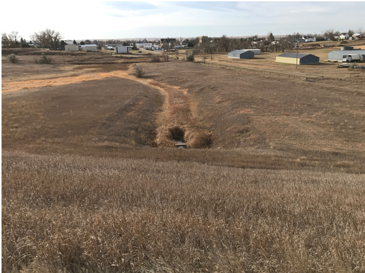
Photo #10- View of Principle Spillway Outlet Works from atop Dam Crest
