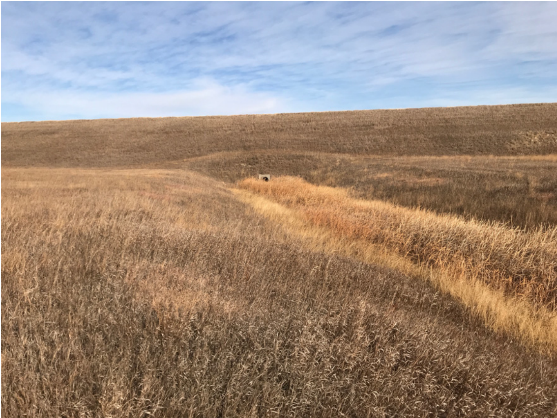
Photo #56- View looking at Outlet Conduit and Plunge Pool from Outlet Channel
