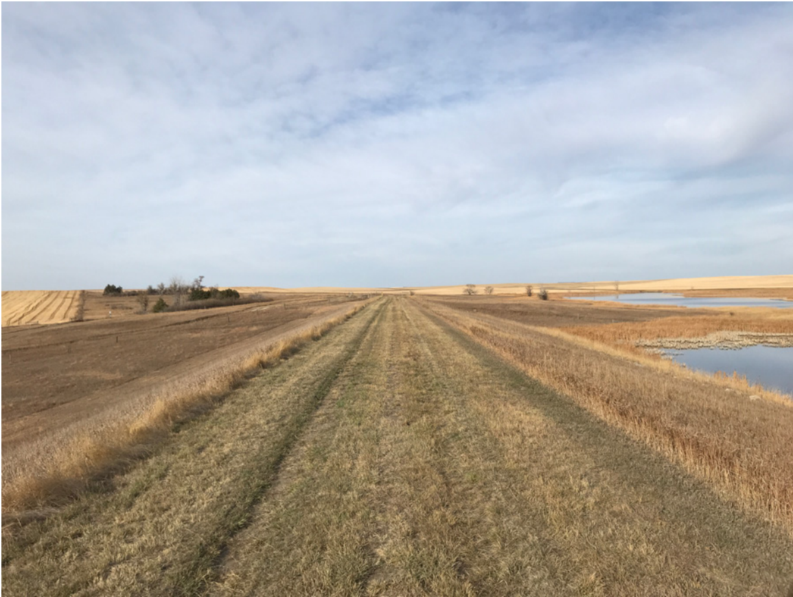
Photo #11 - View from Dam Crest looking toward Right Abutment
