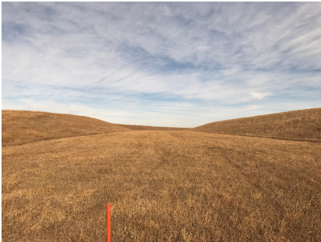
Photo #54- View from End of Exit Section looking up Auxiliary Spillway
