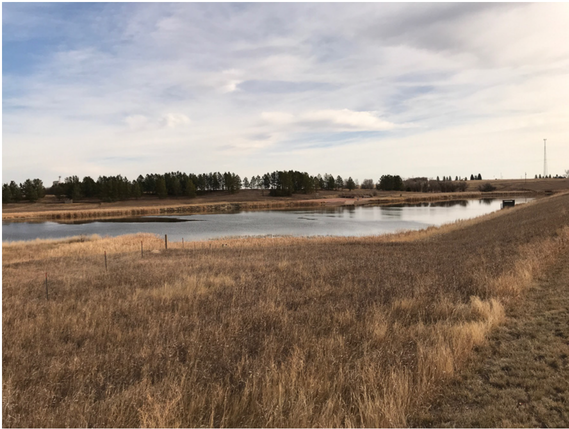
Photo #37 - View looking down Right Abutment Upstream Groin
