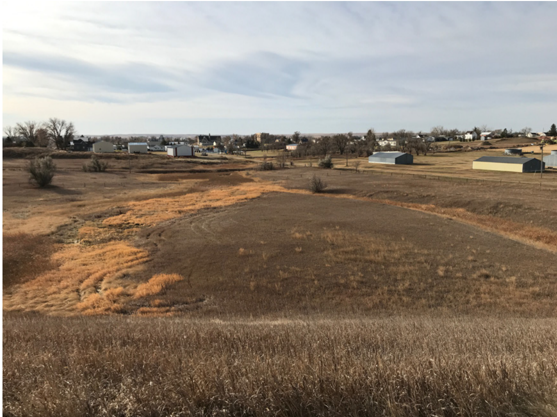
Photo #8- View of Downstream Channels from atop Dam Crest
