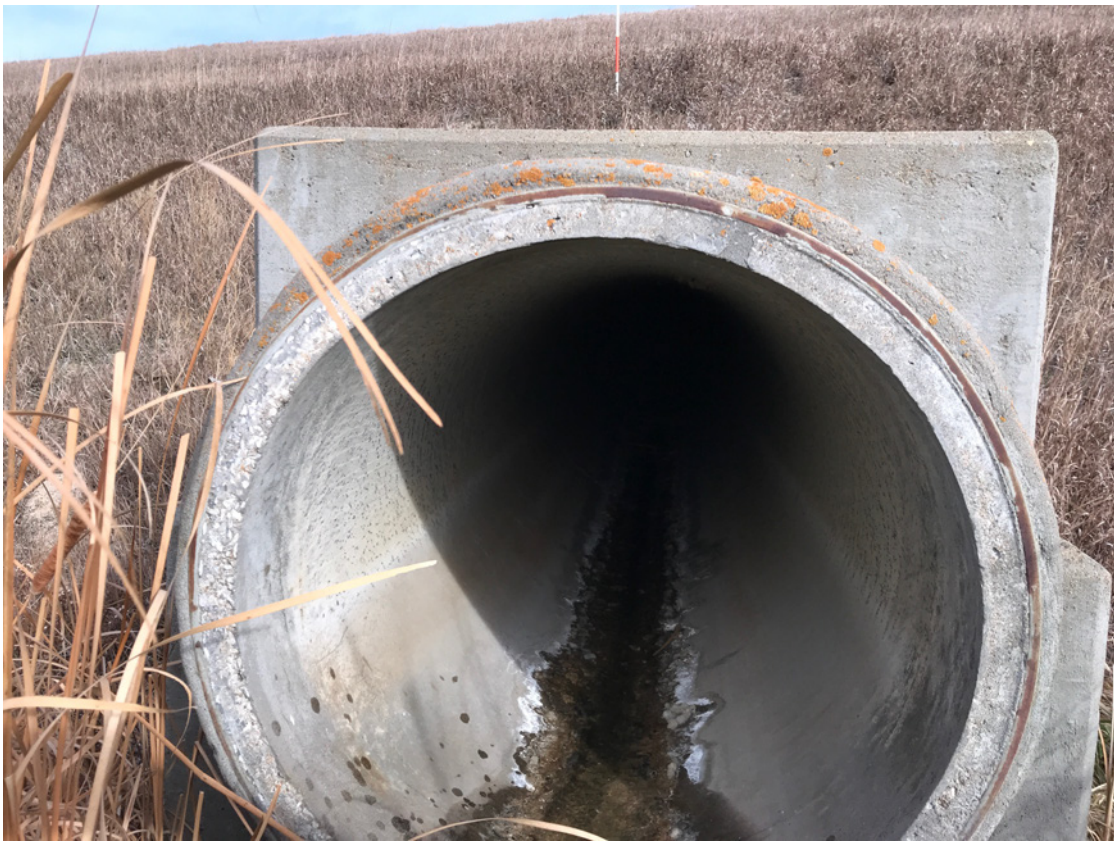
Photo #31 - View of Outlet Conduit End
