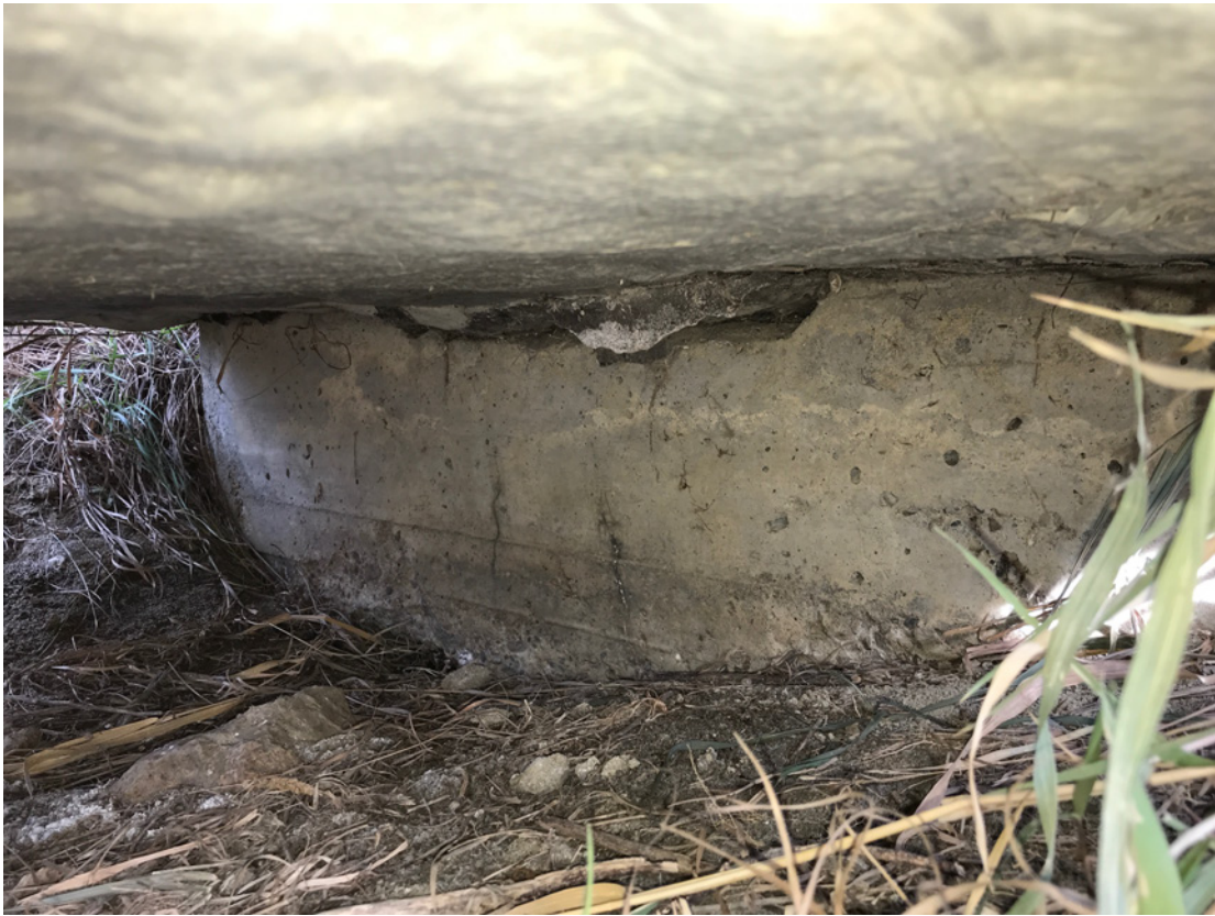
Photo #35 - View of Foundation Wall Supporting Outlet Conduit Cradle
