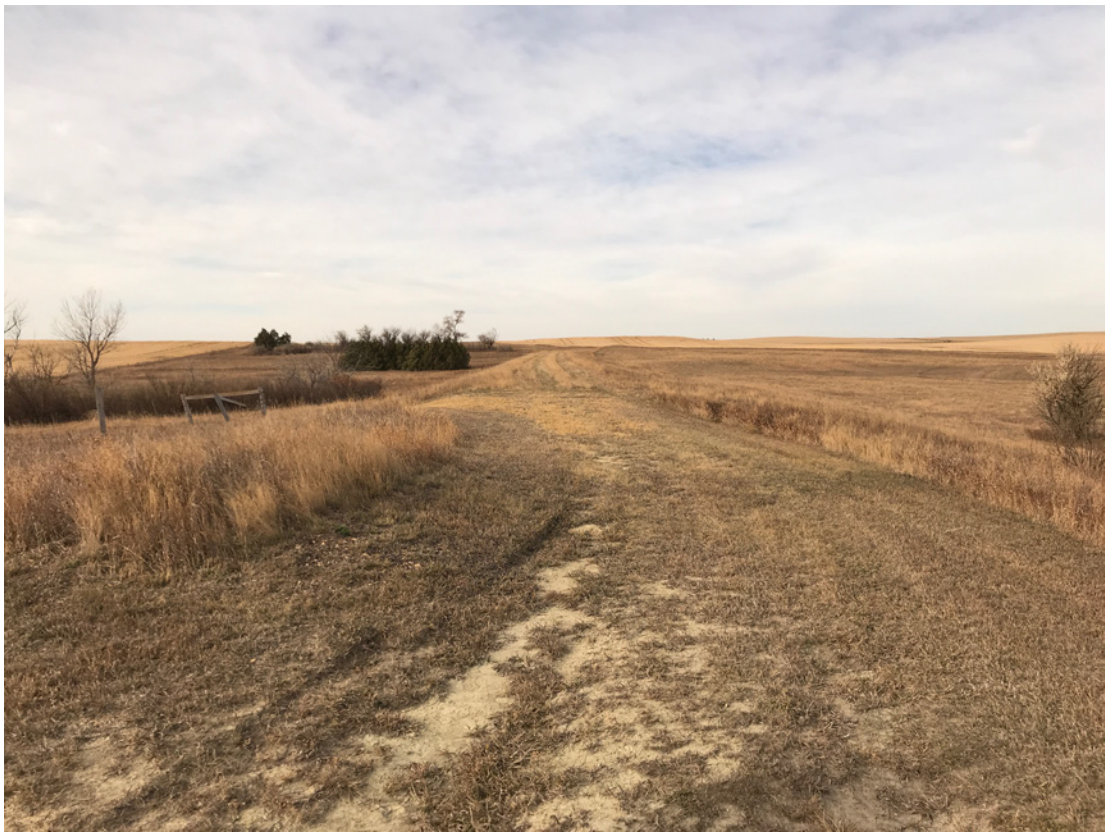
Photo #39 - View looking West long Embankment Crest
