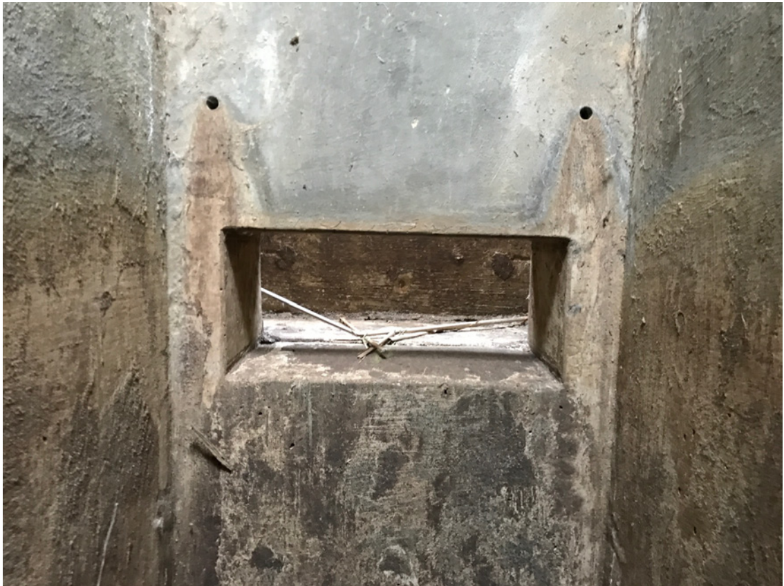
Photo #14 - View of Stage-1 Inlet Orifice from with Riser Tower Structure
