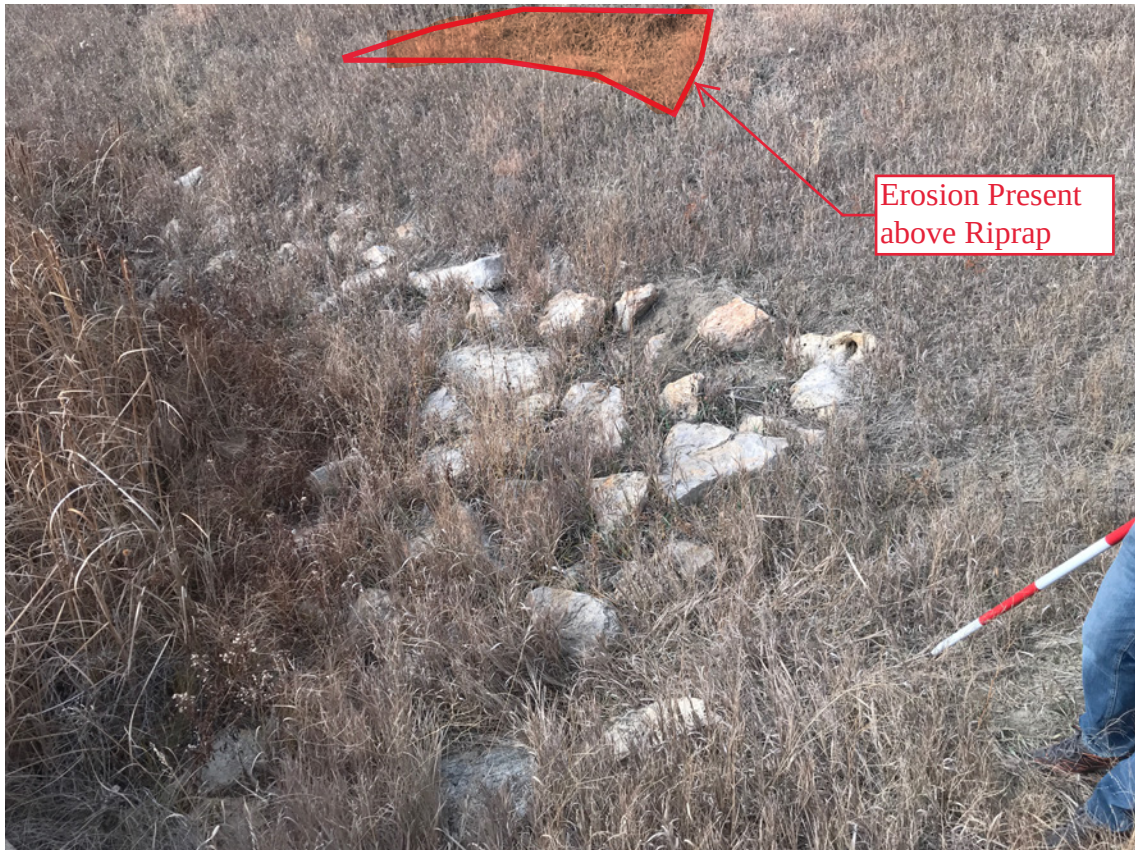
Photo #30- View of Plunge Pool Riprap with Erosion Present above RipRap
