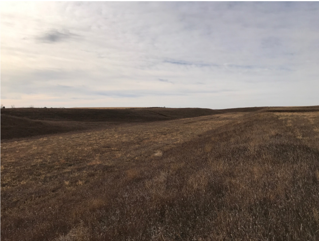
Photo #48- View looking into Auxiliary Spillway
