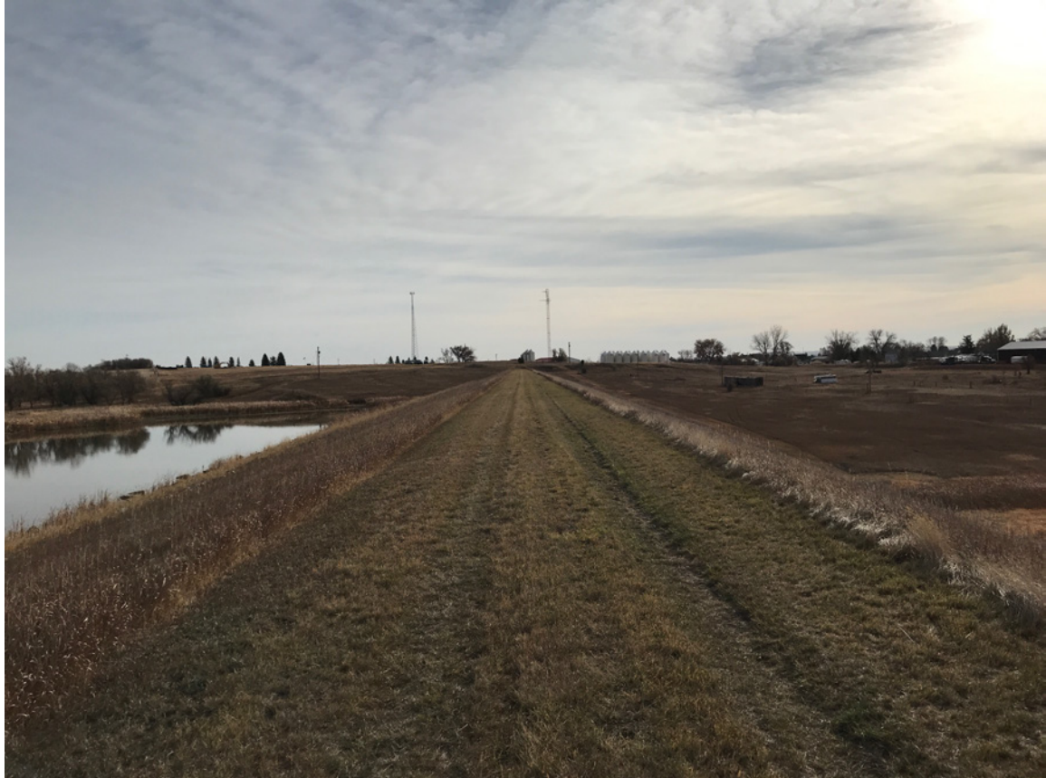
Photo #12 - View from Dam Crest looking toward Left Abutment
