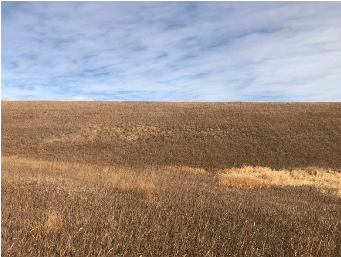
Photo #57 - View of Downstream Face of Embankment
