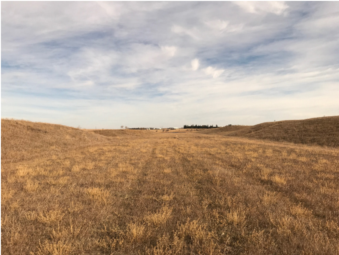
Photo #50- View within Auxiliary Spillway looking toward Reservoir
