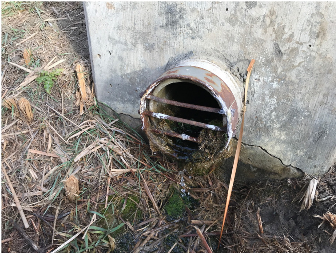
Photo #6 - View of Foundation Drain at Toe of Downstream Face
