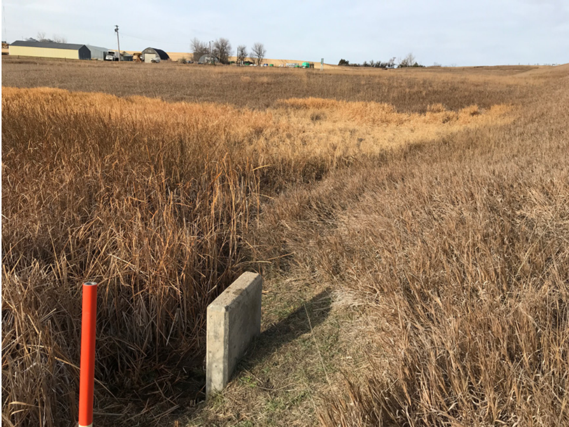
Photo #7- View of Foundation Drain Outlet Structure
