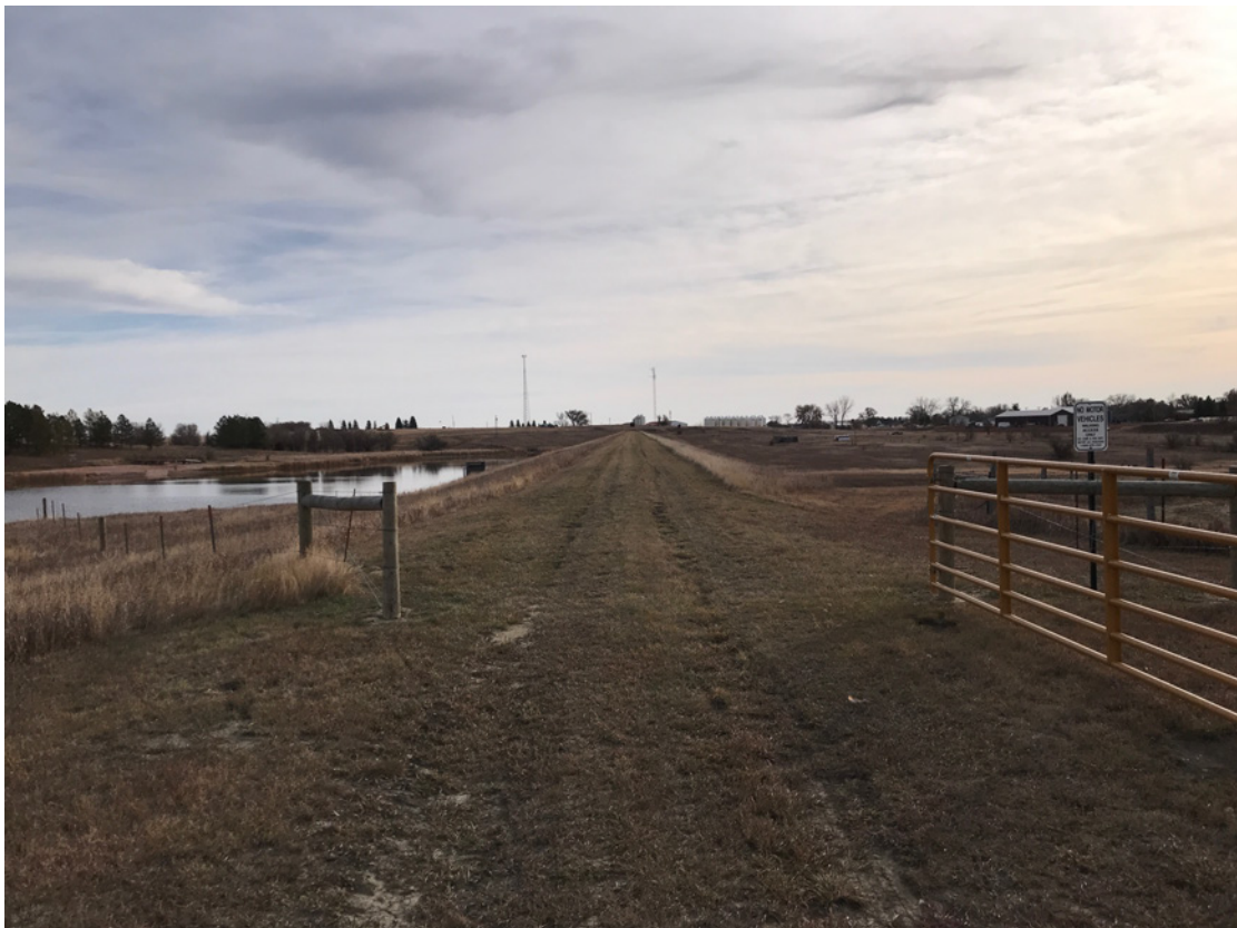
Photo #40- View looking East along Embankment Crest from Gate Entrance to Main Dam Embankment
