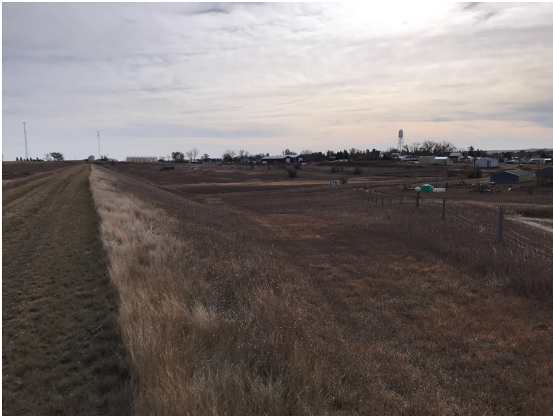
Photo #38- View looking down Right Abutment Downstream Groin
