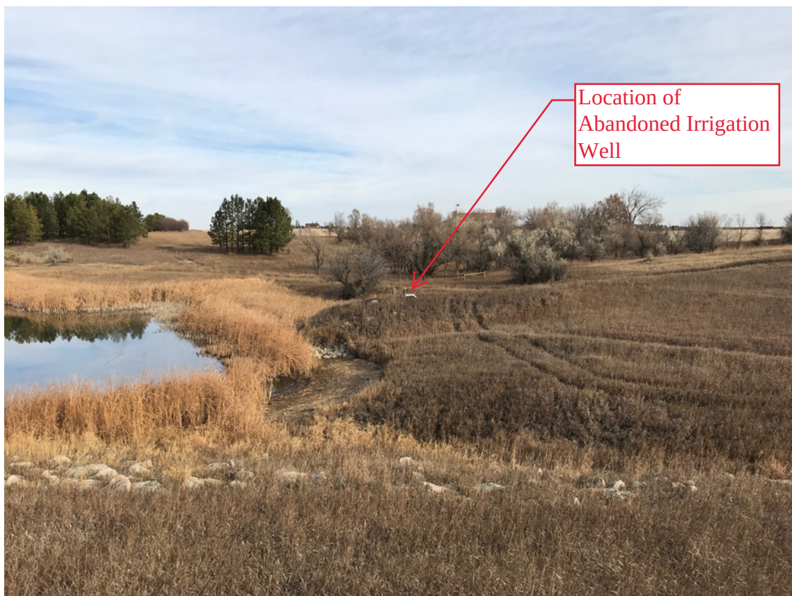
Photo #4 - View from Dam Crest looking to Abandoned Irrigation Well for Cemetery
