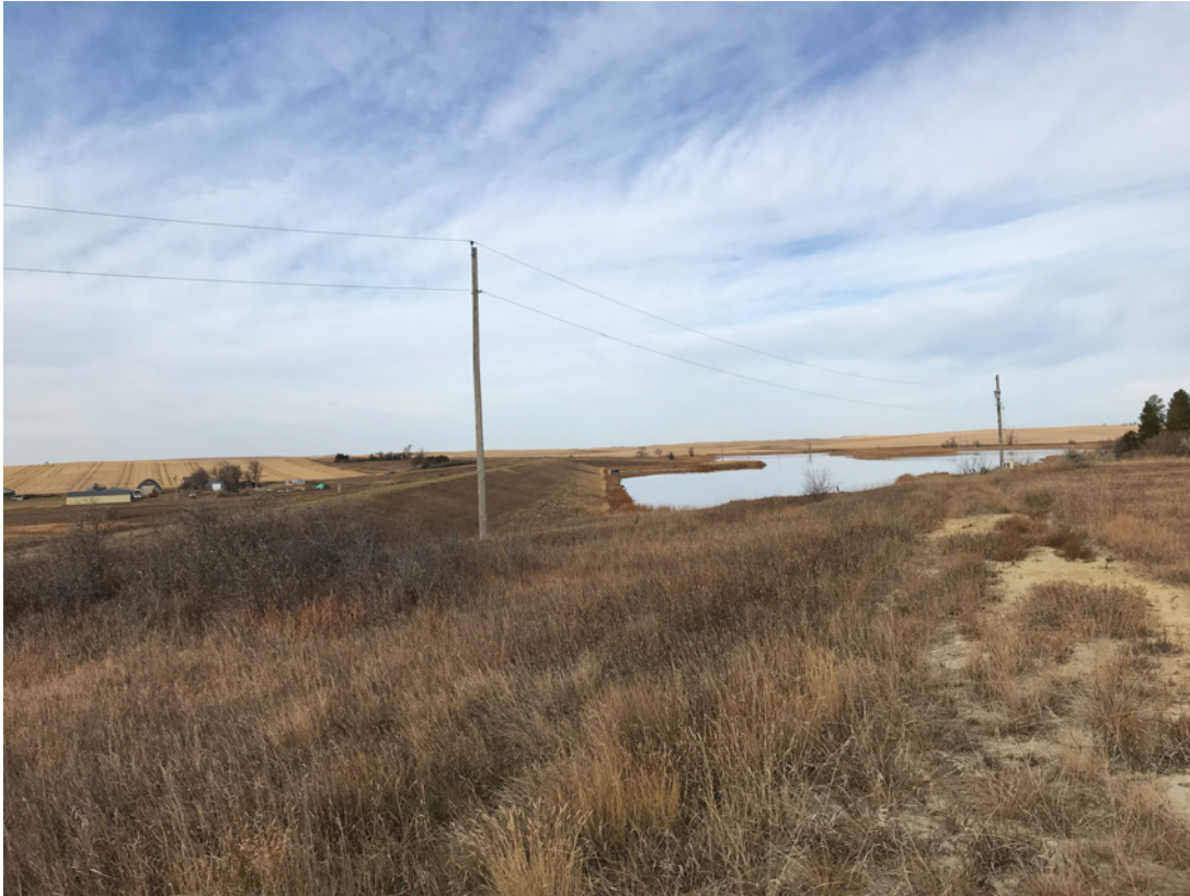
Photo #1 - View from Left Abutment looking along Waterline of Upstream Face
