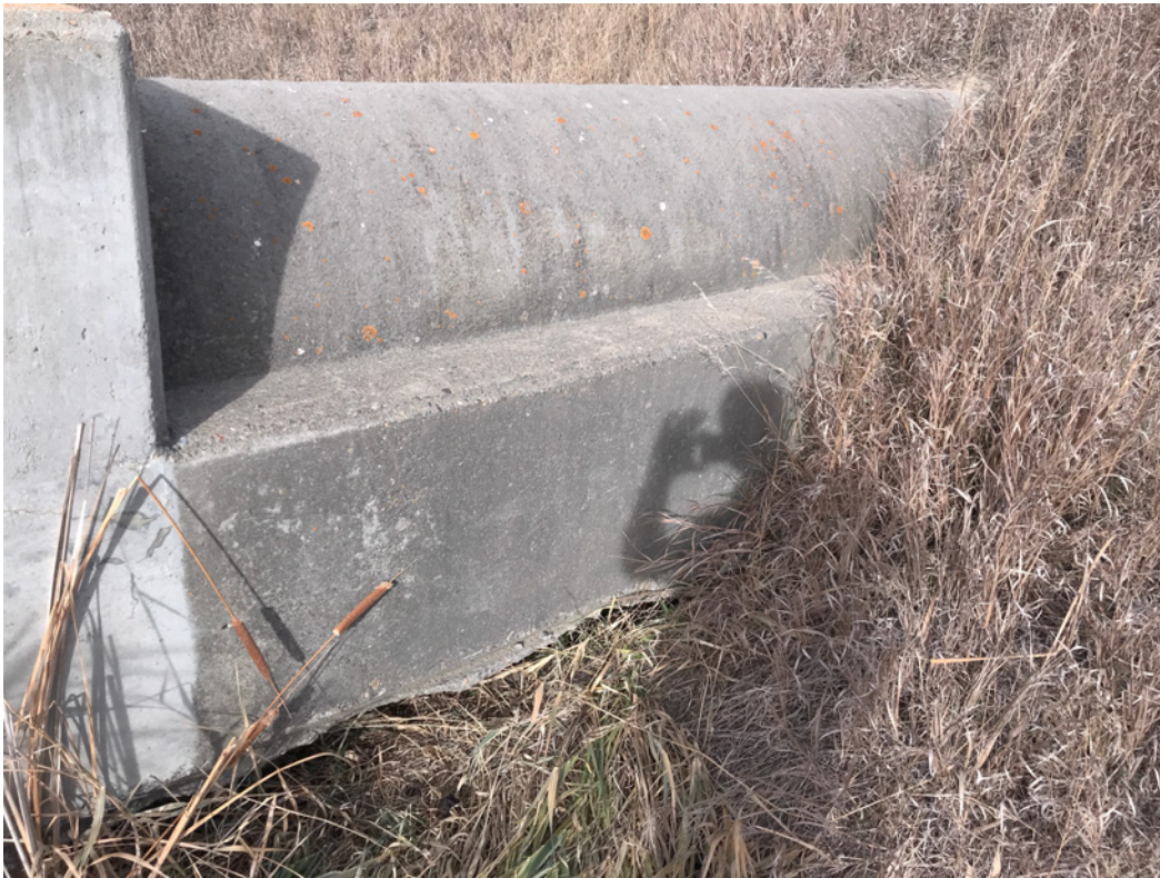
Photo #34- View of Outlet Conduit and Support Cradle
