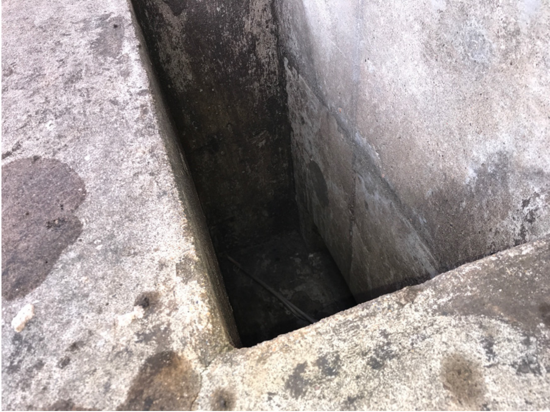
Photo #23- View of looking down Stage-1 Inlet from within Trash Rack
