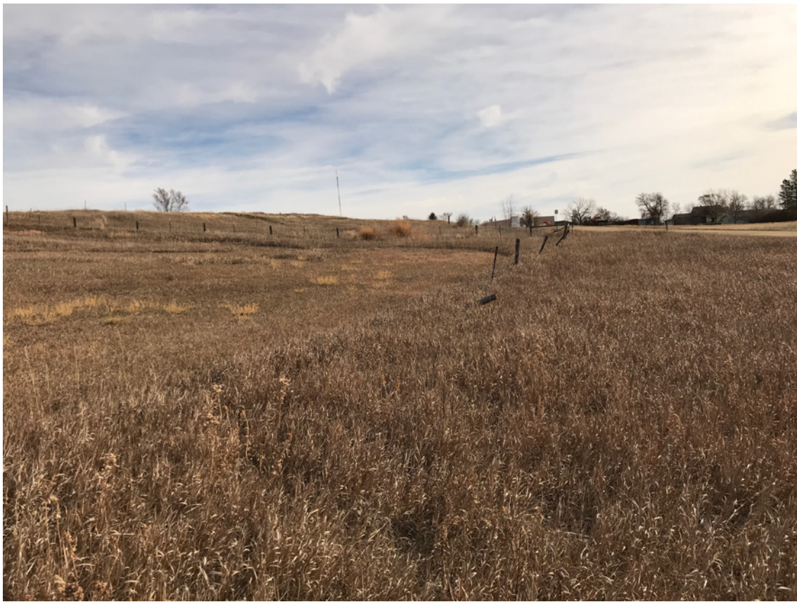
Photo #55 - View looking along End of Exit Section of Auxiliary Spillway
