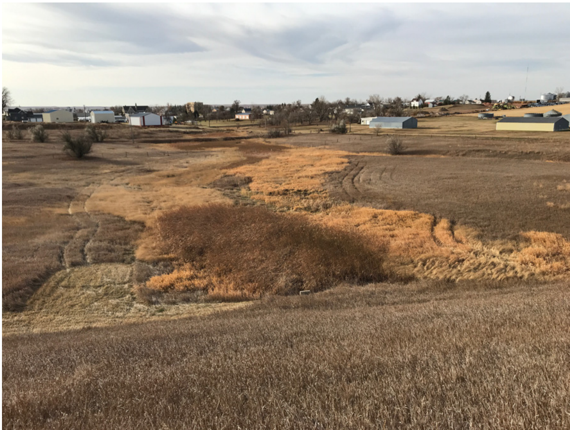
Photo #5 - View from Dam Crest looking down to Foundation Drain at Toe of Downstream Face
