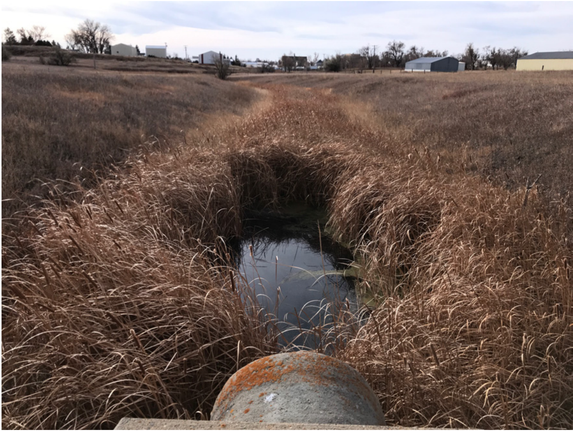
Photo #29 - View of Plunge Pool from atop Outlet Conduit
