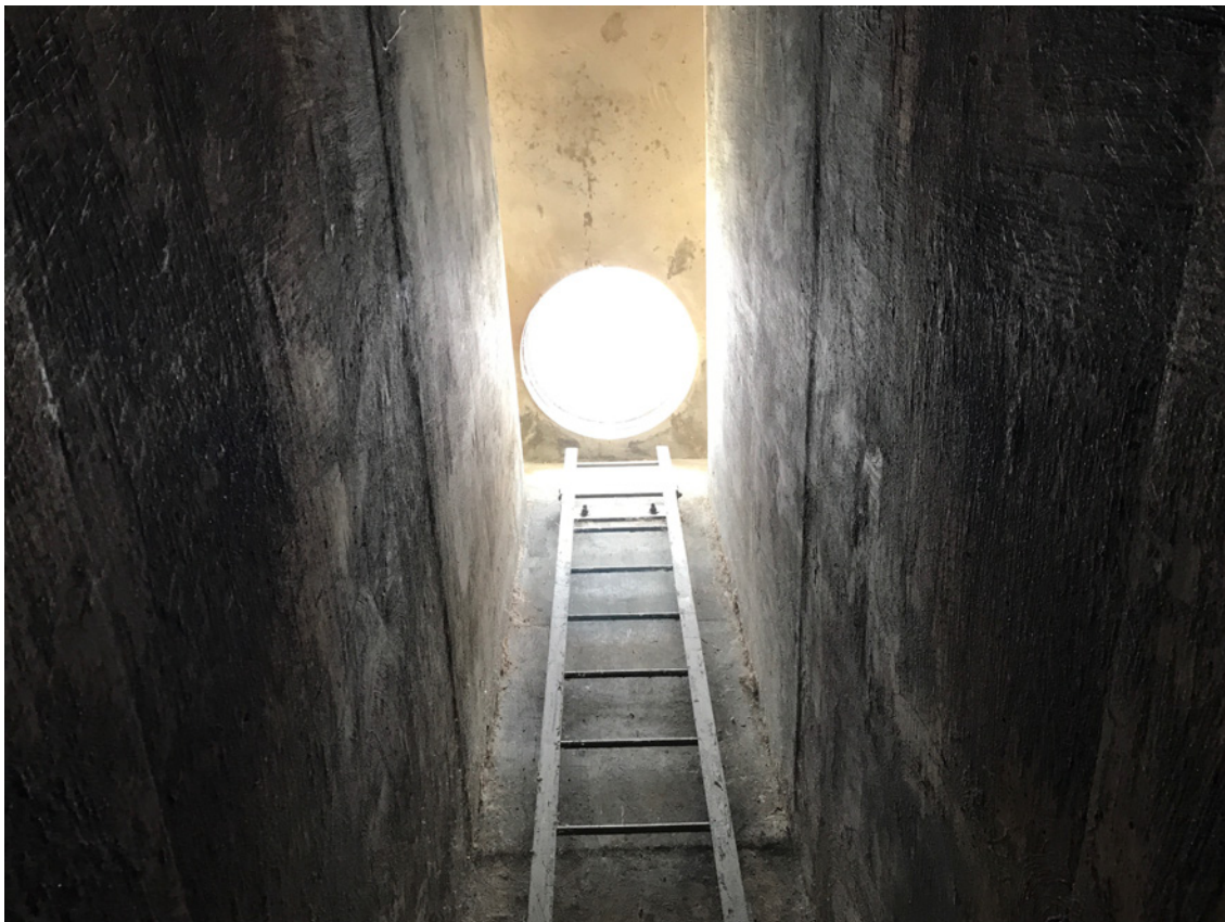
Photo #16 - View looking up at Manhole from within Riser Tower Structure
