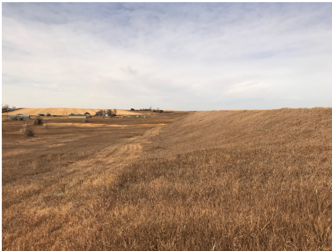
Photo #58- View of Downstream Face of Embankment from Left Abutment Groin
