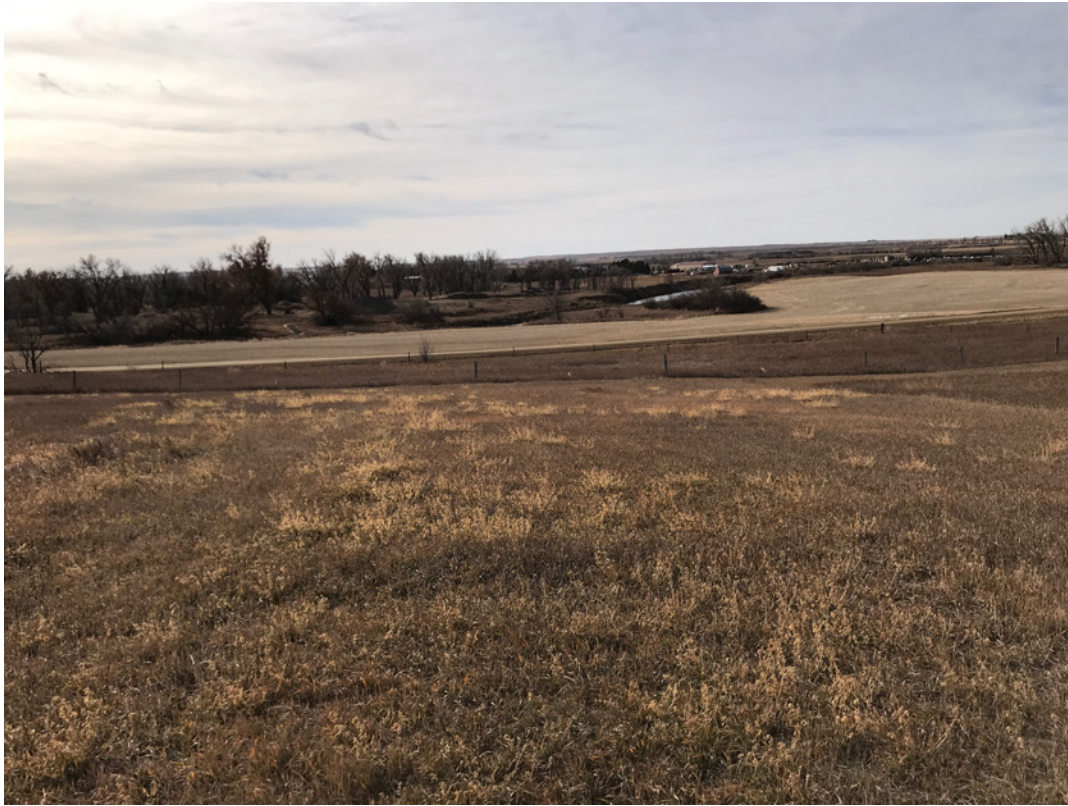
Photo #53 - View looking at end of Exit Section of Auxiliary Spillway
