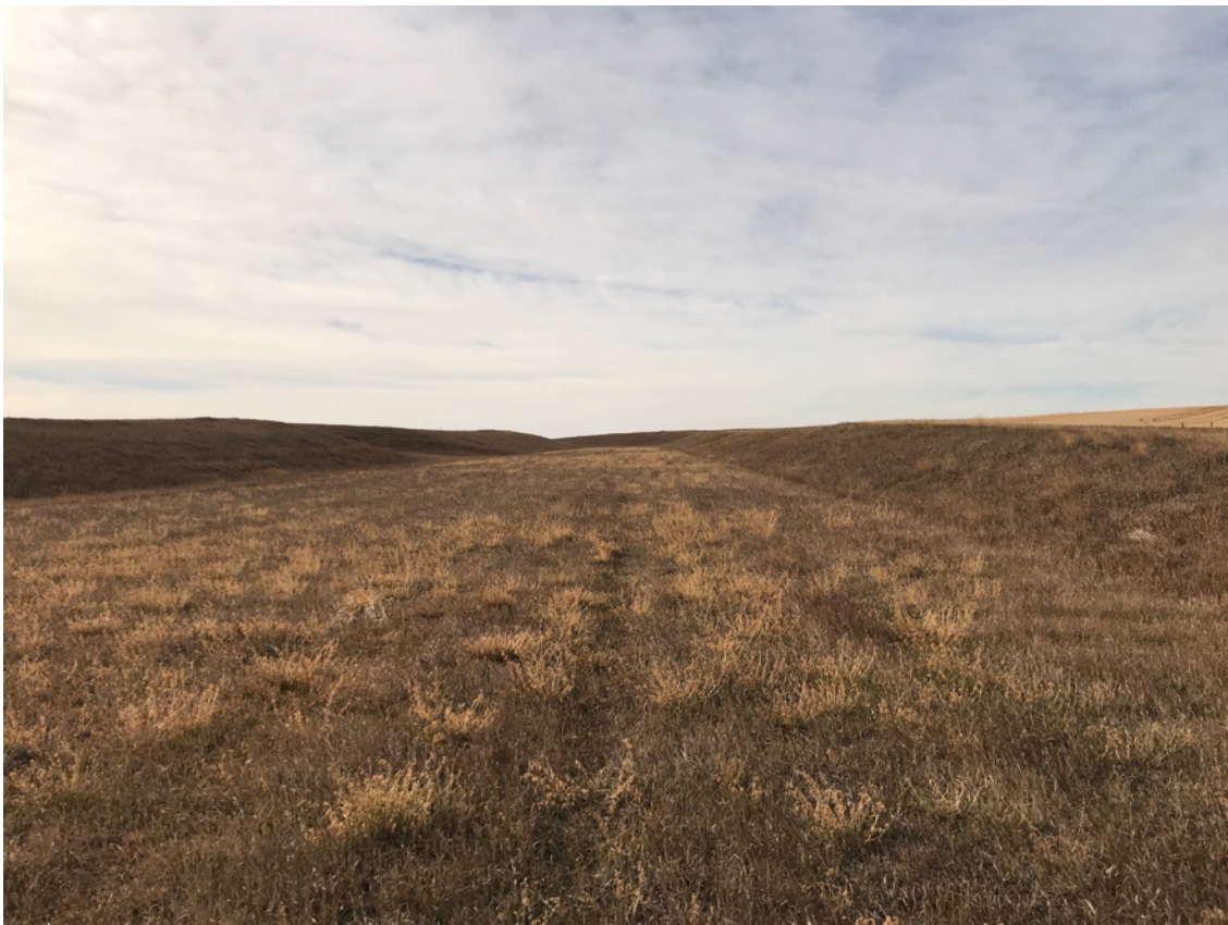
Photo #47 - View within Auxiliary Spillway
