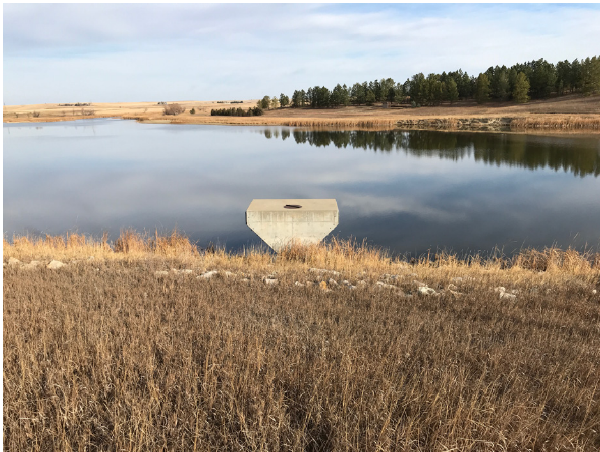
Photo #9 - View of Principle Spillway Riser Tower Structure from atop Dam crest
