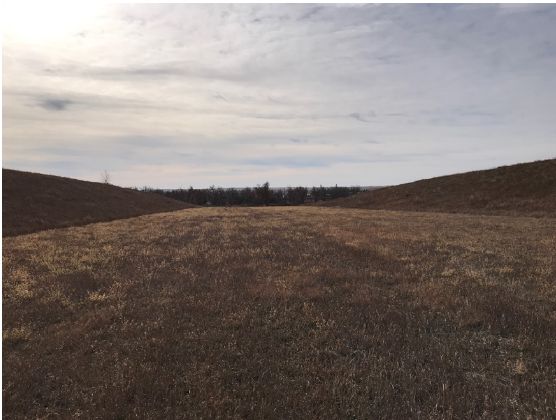
Photo #52- View within Auxiliary Spillway looking toward Reservoir
