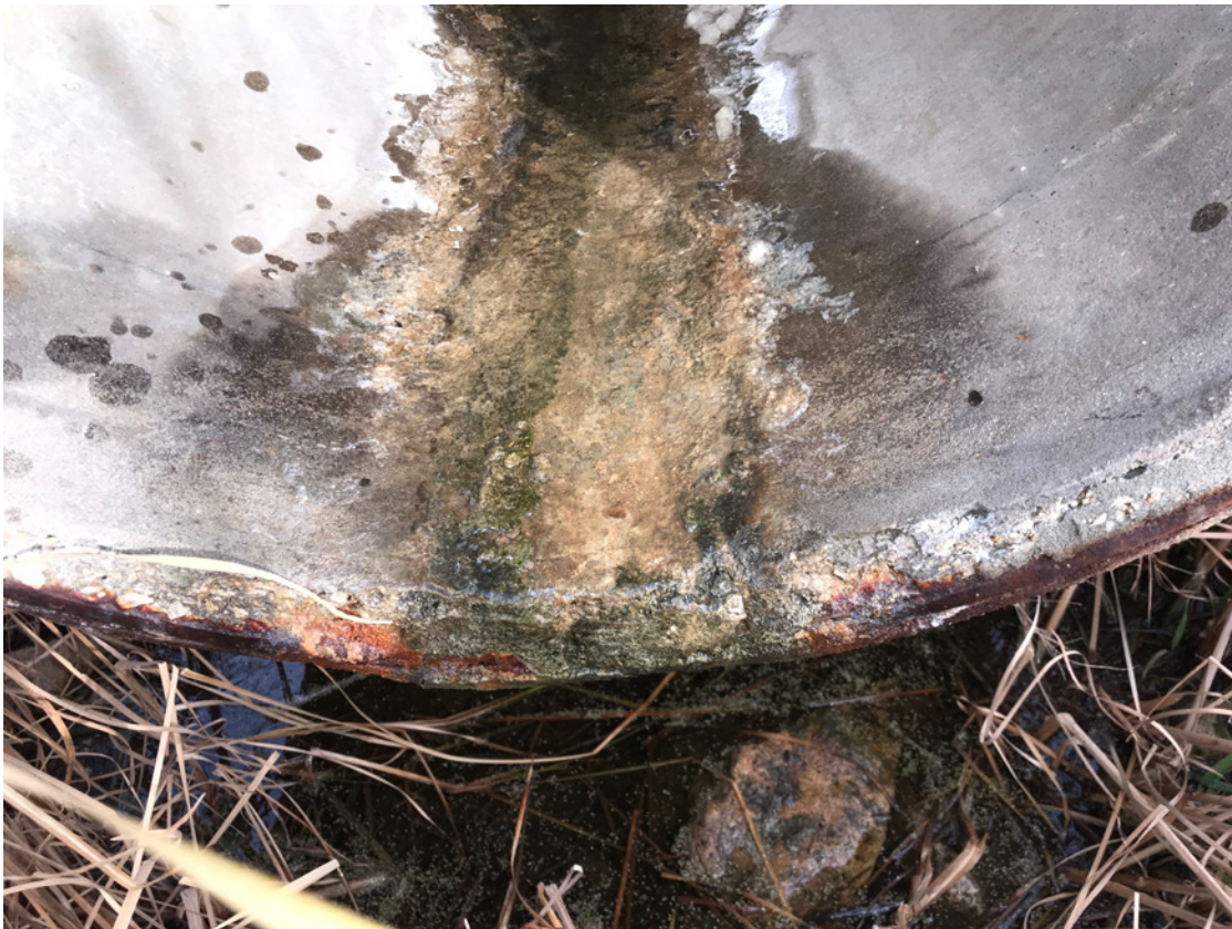
Photo #32- View of of Bottom Edge of Outlet Conduit End
