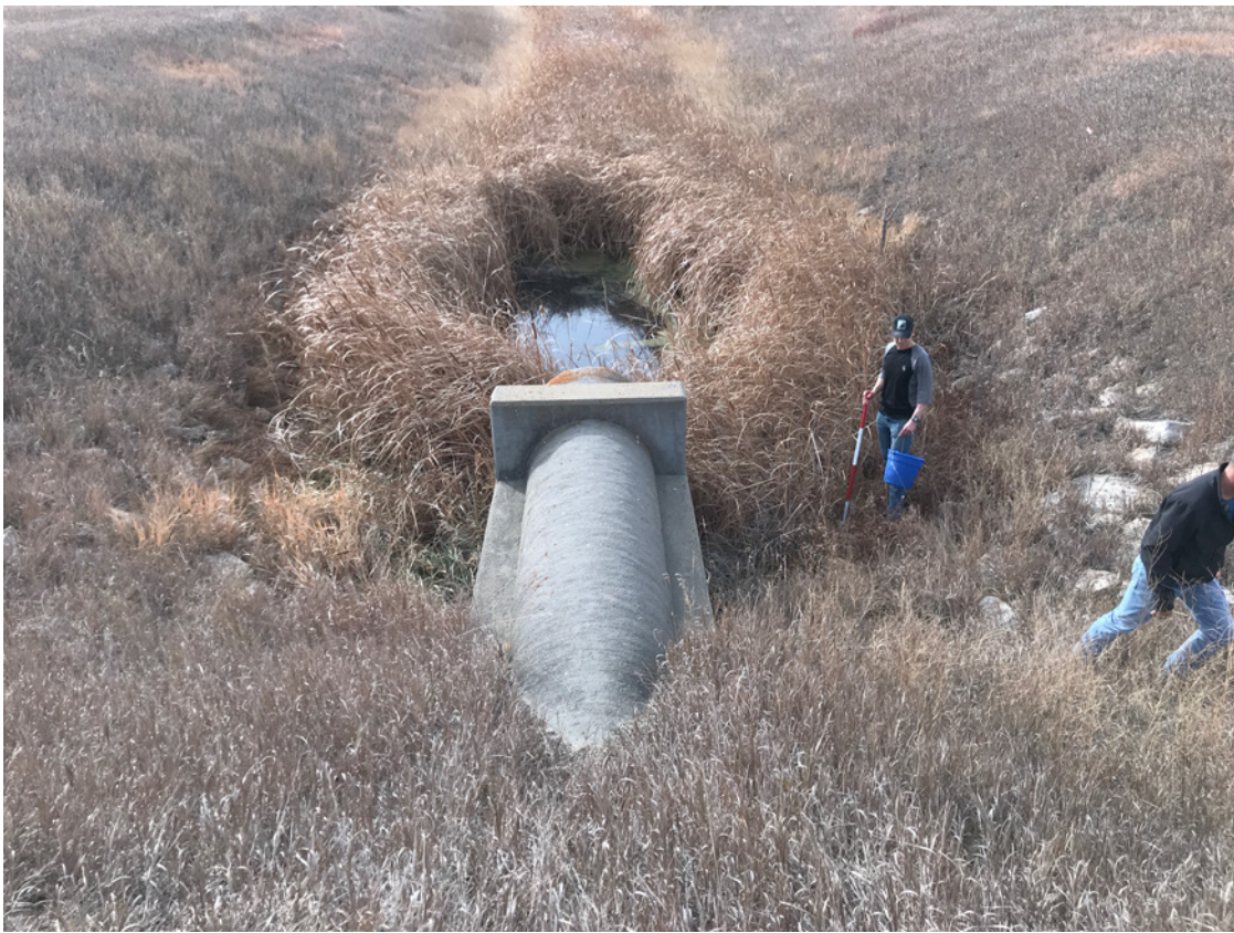
Photo #27 - View of Principle Spillway Outlet Conduit and Plunge Pool
