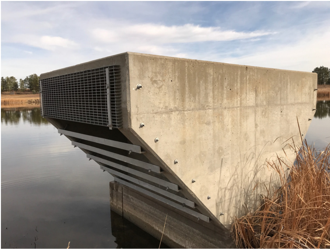
Photo #25 - View Riser Tower Structure
