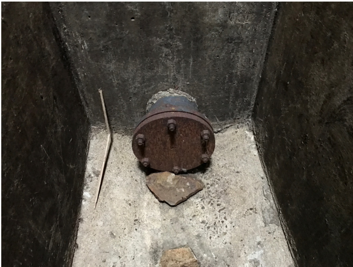
Photo #15 - View of Low-Level Inlet from within Riser Tower Structure
