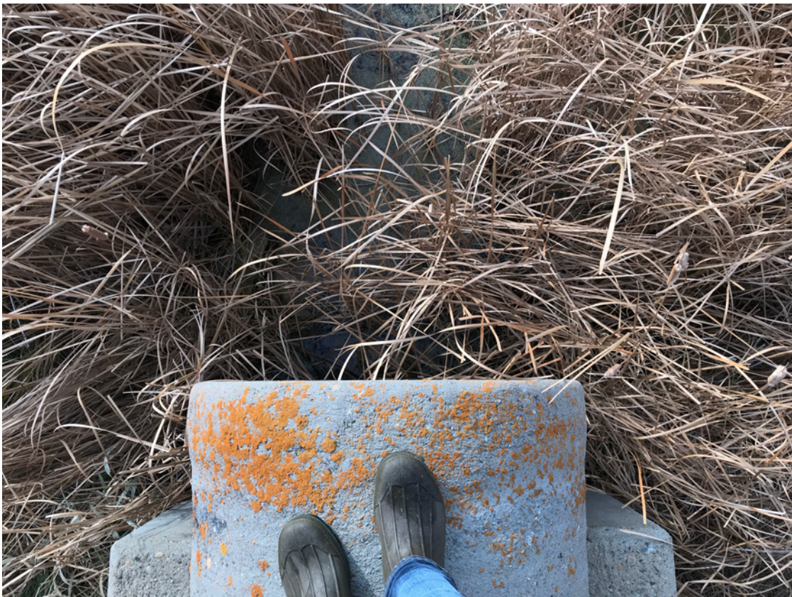
Photo #28- View of Principle Spillway Outlet Conduit End
