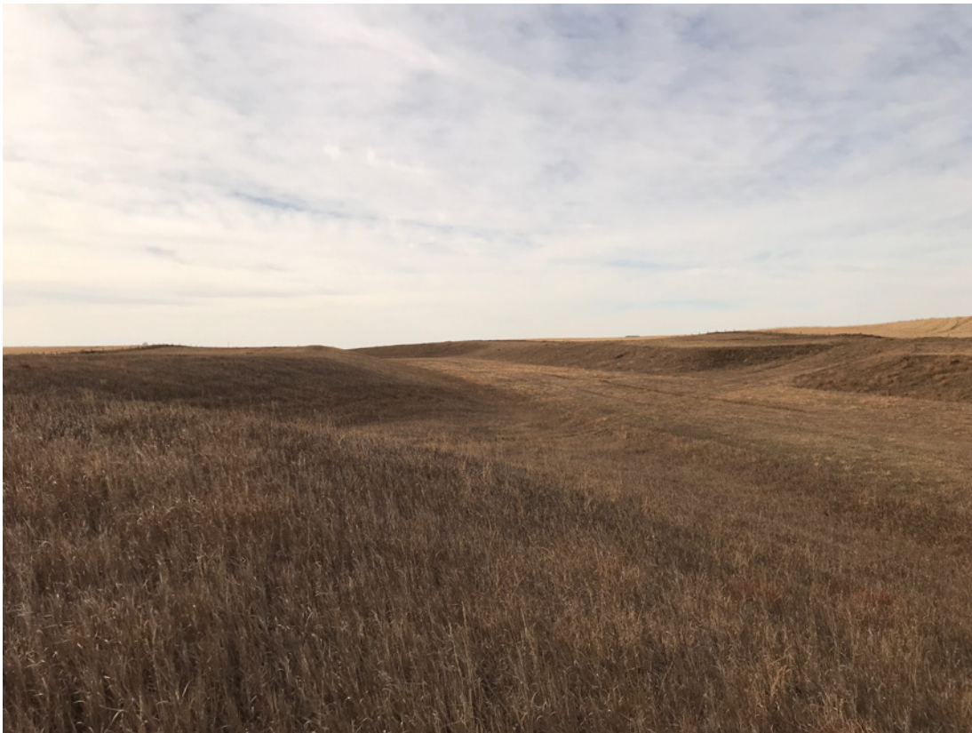
Photo #46- View looking into Auxiliary Spillway
