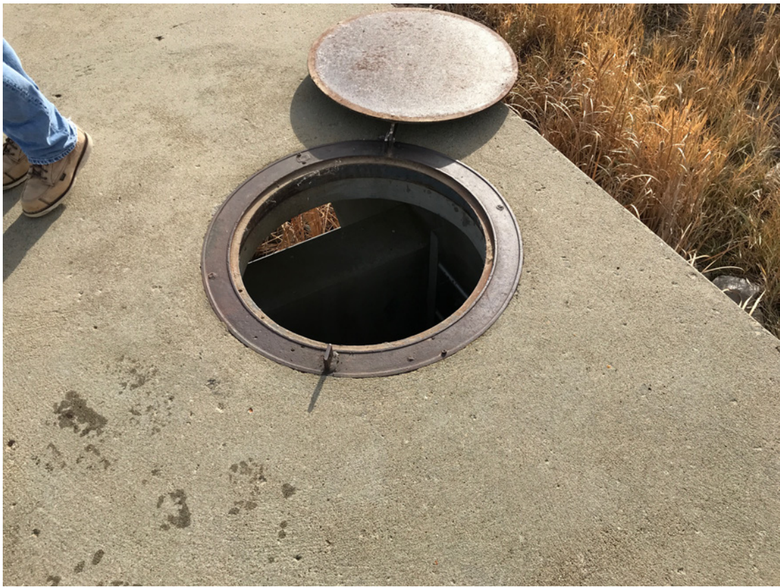
Photo #13 - View of Manhole atop Riser Tower Structure
