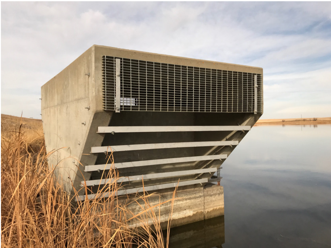
Photo #26- View Riser Tower Structure
