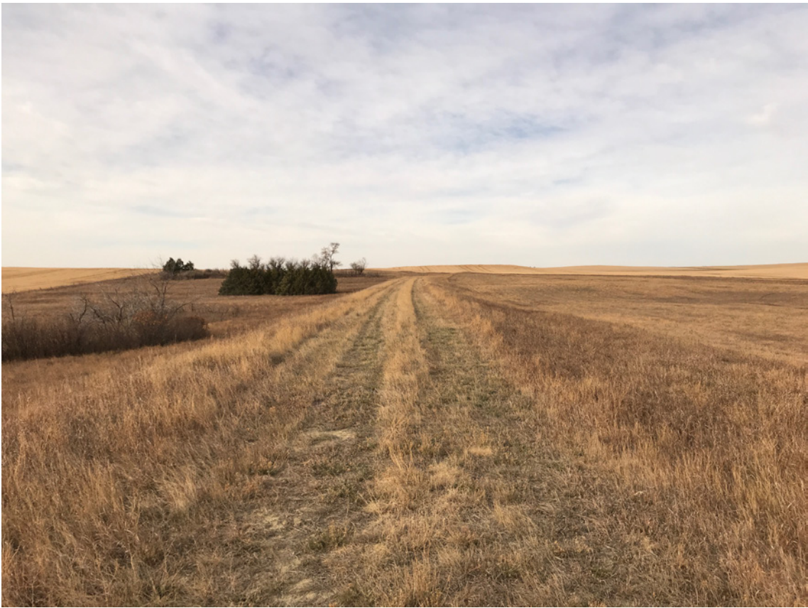
Photo #41 - View of looking West along Dam Embankment
