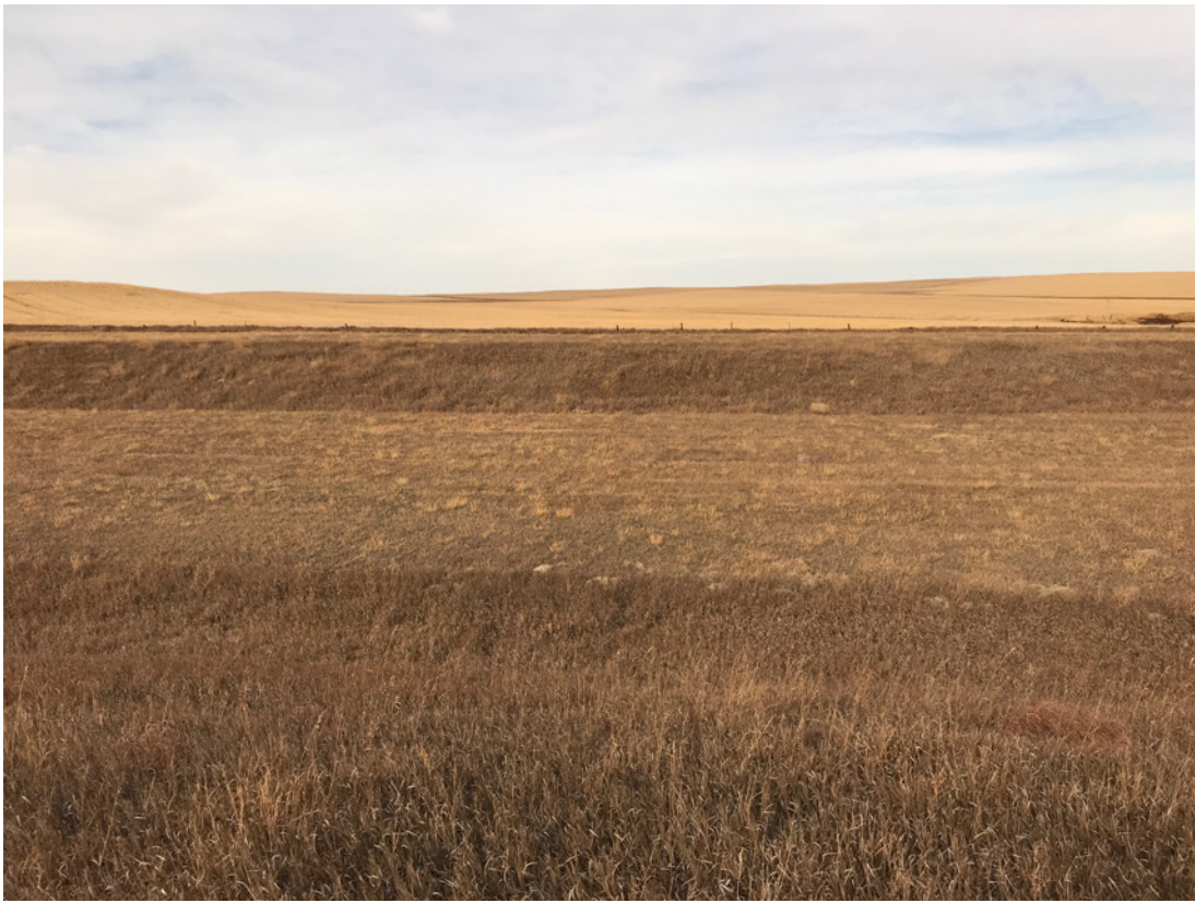
Photo #45 - View looking into Auxiliary Spillway
