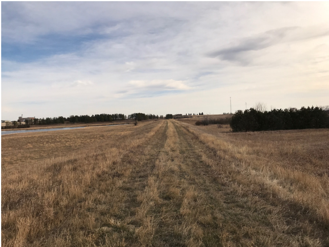
Photo #42- View of looking West along Dam Embankment
