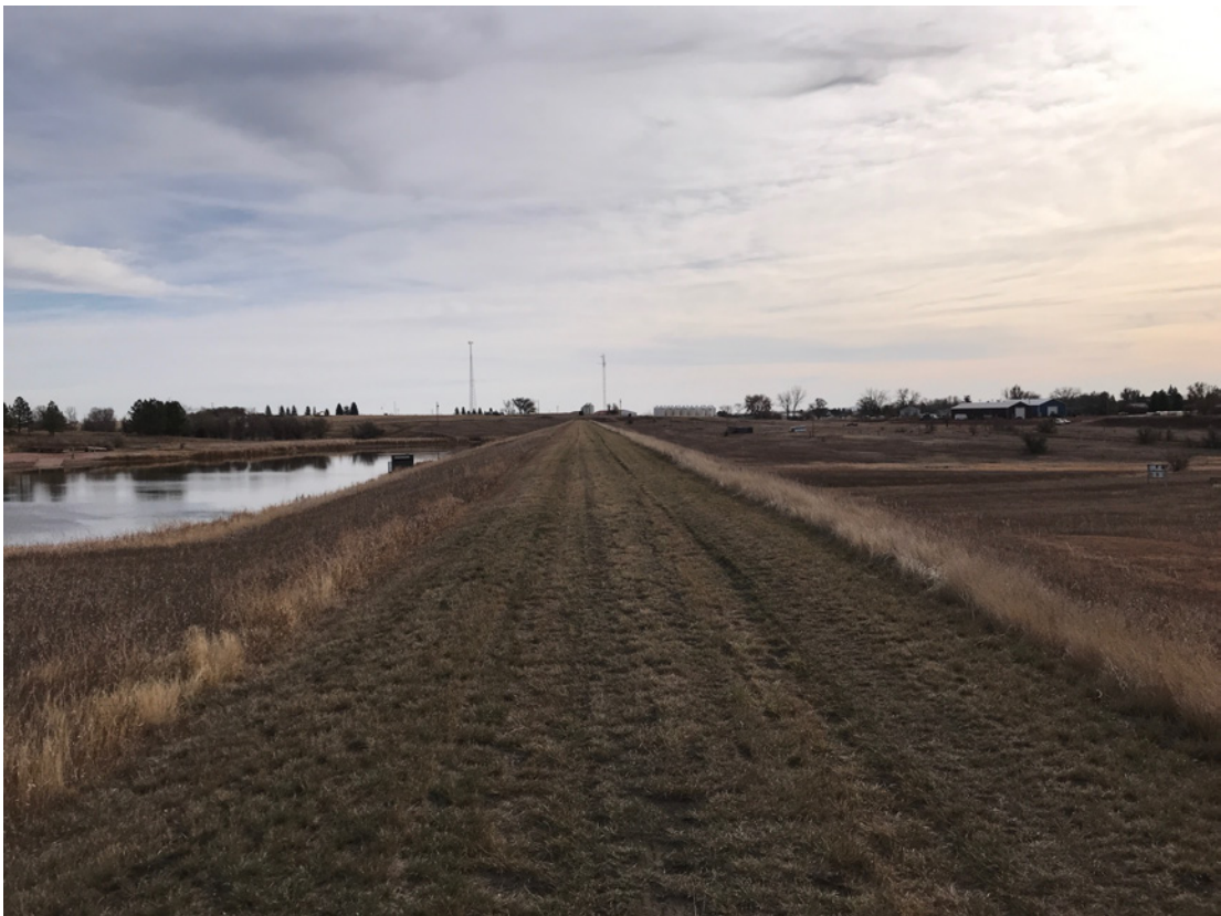
Photo #36- View from Right Abutment looking Along Dam Crest
