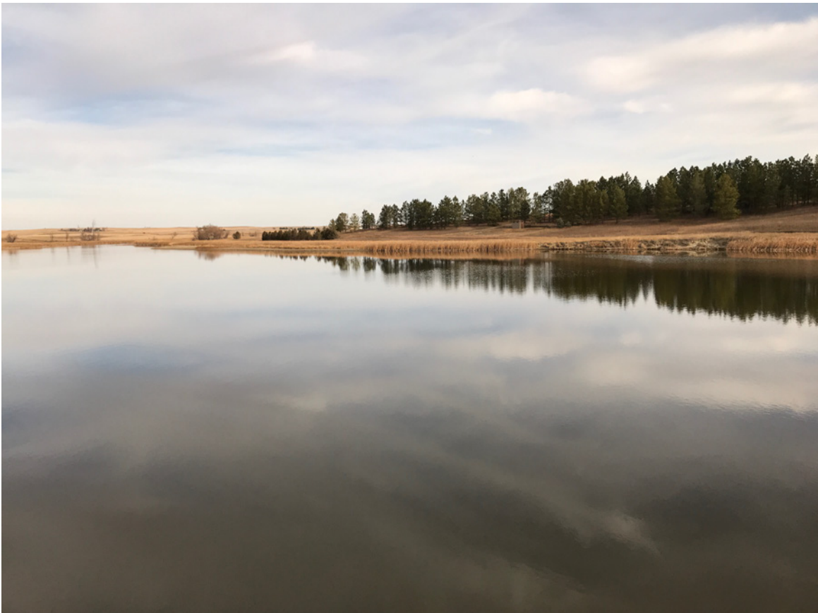
Photo #20- View of Reservoir looking North from atop Riser Tower Structure
