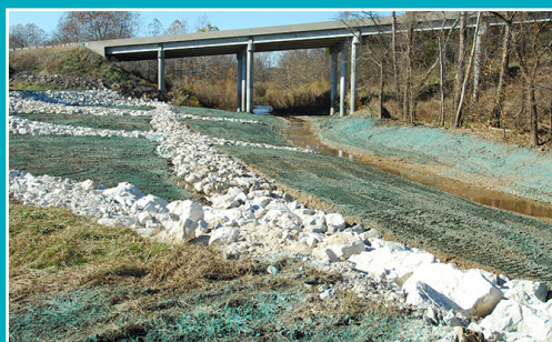
The before-and-after photos above show EWP work to repair damage at the Highway 38 bridge over Greasy Creek in Dallas County.
